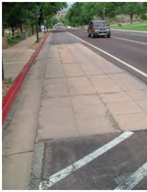
Concrete shuttle pad at Driftwood Lodge
