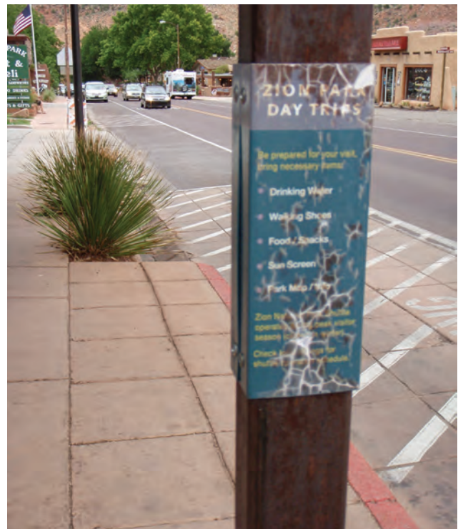
Damaged shuttle information sign
