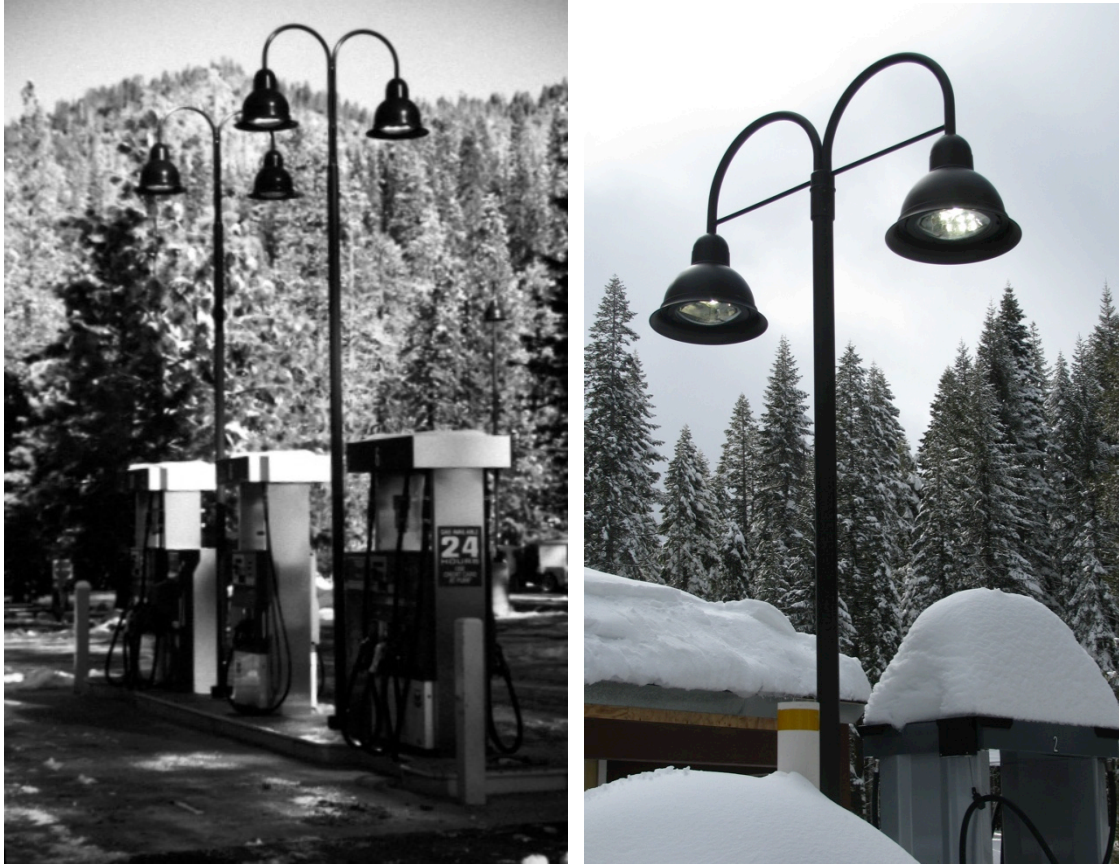
Figure 5 –Tall Pole Lights at (l.) Wawona Gas Station (r.) Crane Flat Gas Station. This design was developed prior to the completion of these Guidelines. Fewer lumens (lower wattage lamps) should be used on similar installations in the future.
