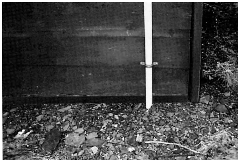
Use concrete to seal holes under foundation
