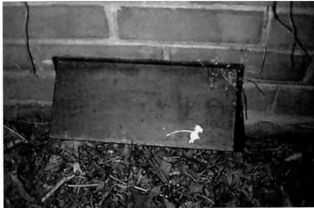
Exhaust flap closes easily and is not blocked open.
