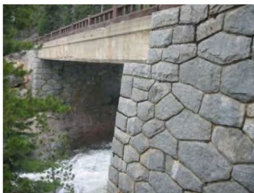
FIGURE 19. SOUTH FORK TUOLUMNE RIVER BRIDGE
