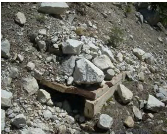
FIGURE 11. ROCKFALL COVERING CULVERT INLET
