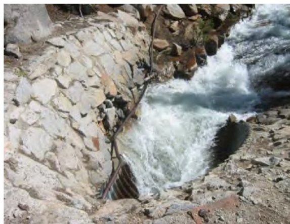
FIGURE 6. CULVERT STONEMWORK
