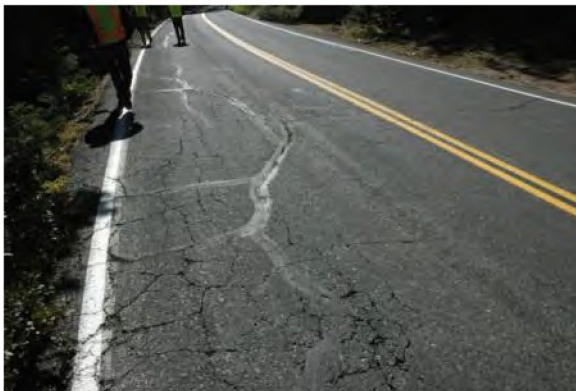
FIGURE 31. CRACK SEALING
