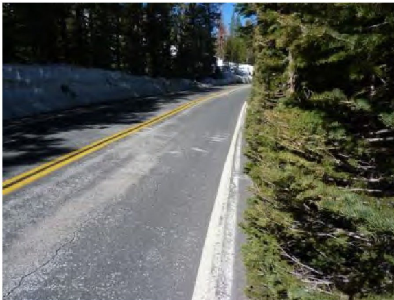
FIGURE 7. VEGETATION ALONG ROAD SHOULDER
