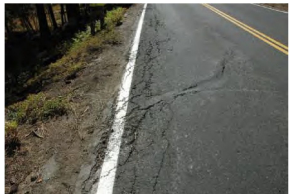
FIGURE 25. CRACKED ASPHALT
