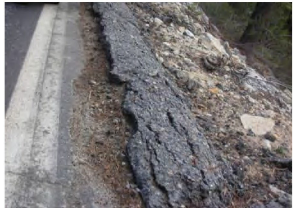
FIGURE 4. FAILED CURB
