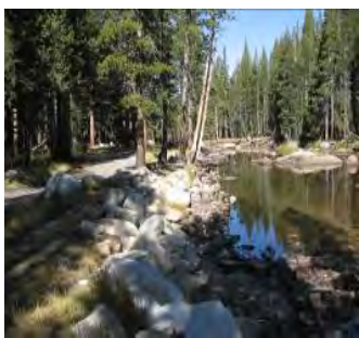
Fig. 1-27. Riprap along river in Tuolumne Campground
