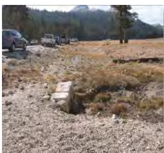
Fig. 1-17. Culvert set too low in meadow
