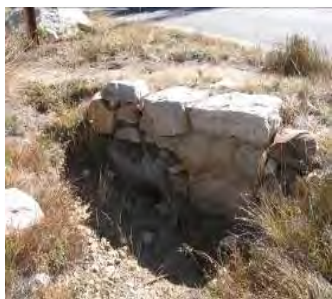
Fig. 1-16. Partially blocked culvert
