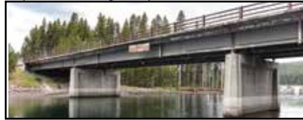
Bridge at Bridge Bay Marina
