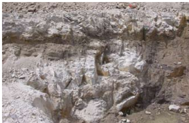
Figure 9. Natural fractures exposed in an excavation for the Norris wastewater treatment plant, June 2004. Notice the near-vertical natural fractures, the spacing of fractures, and the hydrothermally altered fracture surfaces of the Lava Creek B tuff. Dark colors show moist zones within the outcrop.
