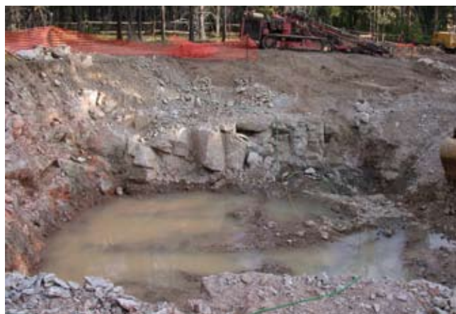
Figure 8. Natural fractures exposed during an excavation for the Norris water treatment plant, September 2003. The water level in the excavation is about ( \pm 1 foot) equal to the water level of the nearby Gibbon River.
