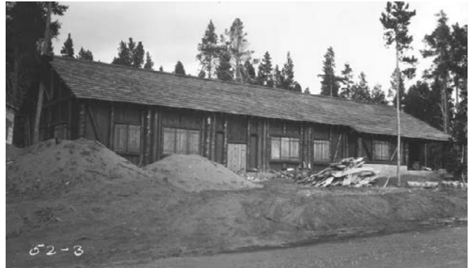
The newly constructed Yellowstone Lake Fish Hatchery, 1928.
