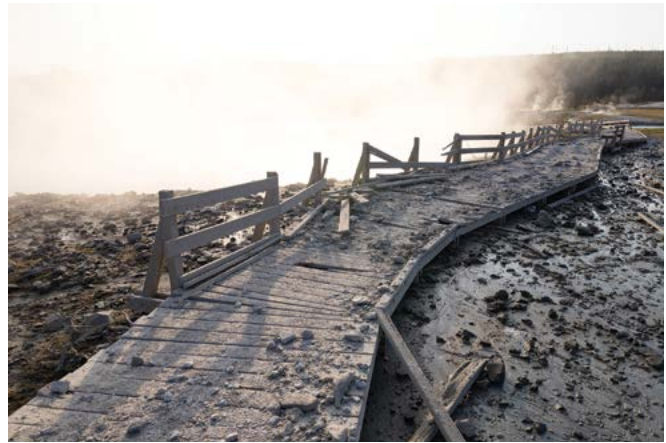
A section of boardwalk near the hydrothermal explosion at Biscuit Basin was destroyed. Although visitors were present at the time of the event, no injuries were reported.
