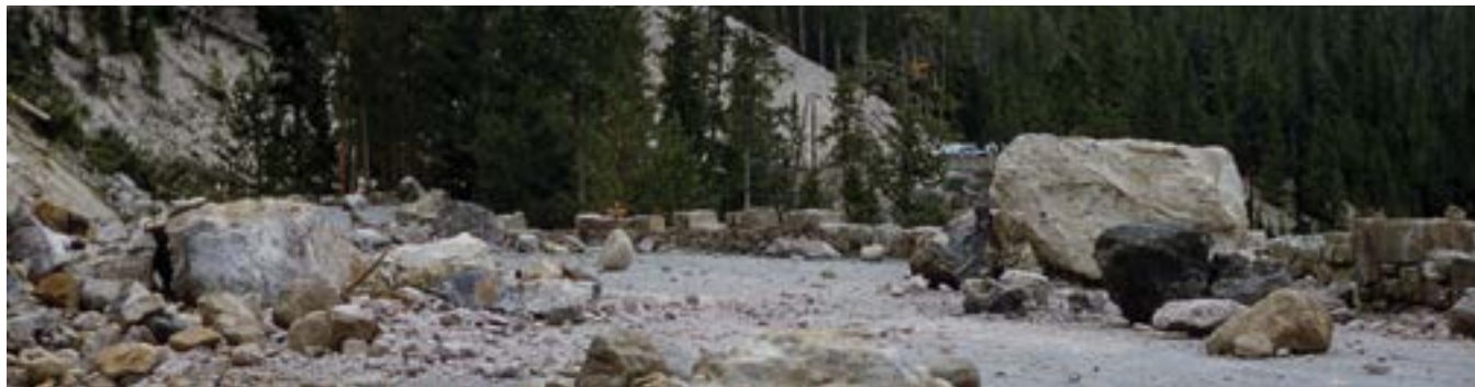
Anywhere from 700 to 3,000 earthquakes occur each year in the Yellowstone area; most are not felt. The 1959 Hebgen Lake earthquake (7.3 M ) caused significant damage to park roads, shown here near Gibbon Falls.
