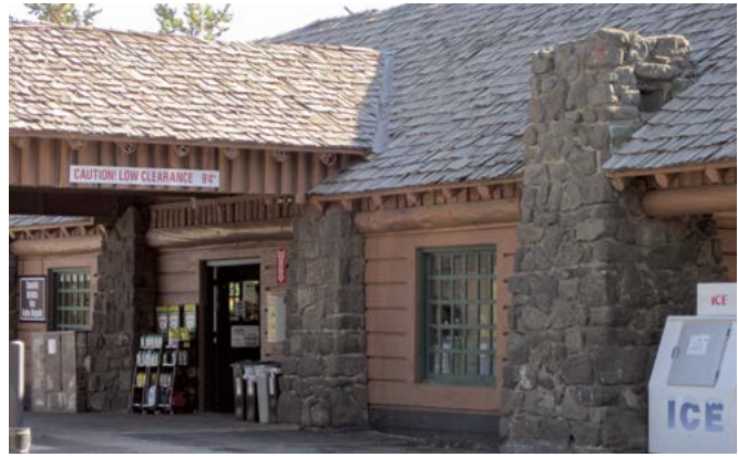
The Old Faithful Upper Service Station, built in 1929, is an example of rustic architecture, intended to enhance rather than detract from the setting of the Old Faithful Geyser.
