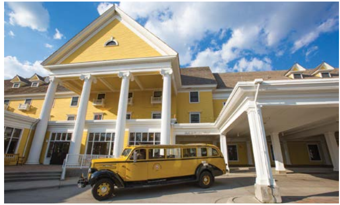
Lake Hotel resembled other hotels financed by the Northern Pacific Railroad when it opened in 1891.
