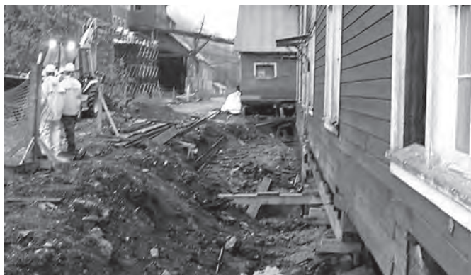
Stabilizing the machine shop (NPS photo)
