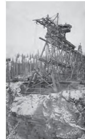
Construction of the Kuskulana bridge
