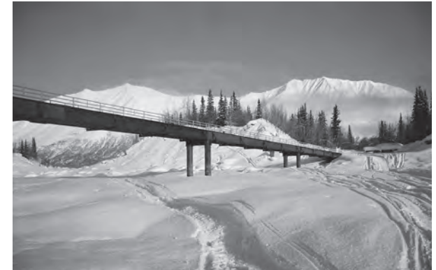
The footbridge was built in 1997.
