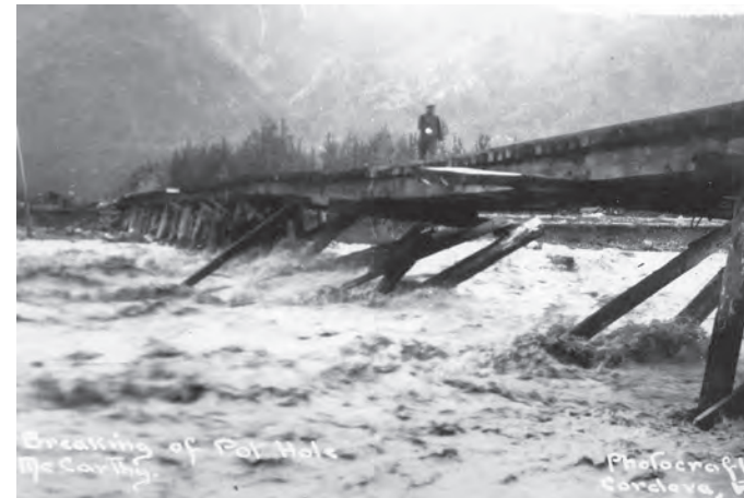
Glacial outbreak flood washing out the railroad bridge across the Kennicott River, which had to be rebuilt frequently. (Candy Waugaman Collection, Fairbanks)
