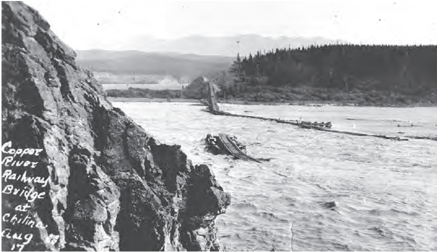
The Copper River bridge at Chitina washed out frequently, as shown here during the flood from a glacial lake break-out in 1932. (Photo courtesy of Geof Bleakley)
