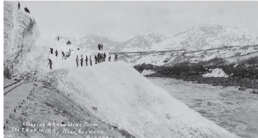
Winter snow slides delayed train operation for weeks at a time while crew of men worked to clear the track.
