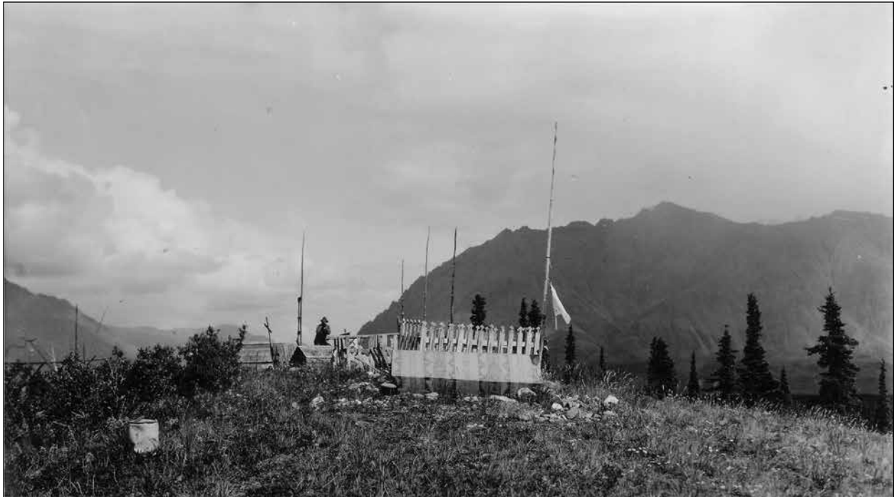
Figure 28. Cross Creek Village Cemetery, 1939. T. W. Ranta no. 56, USGS Photo Archives, Denver.
