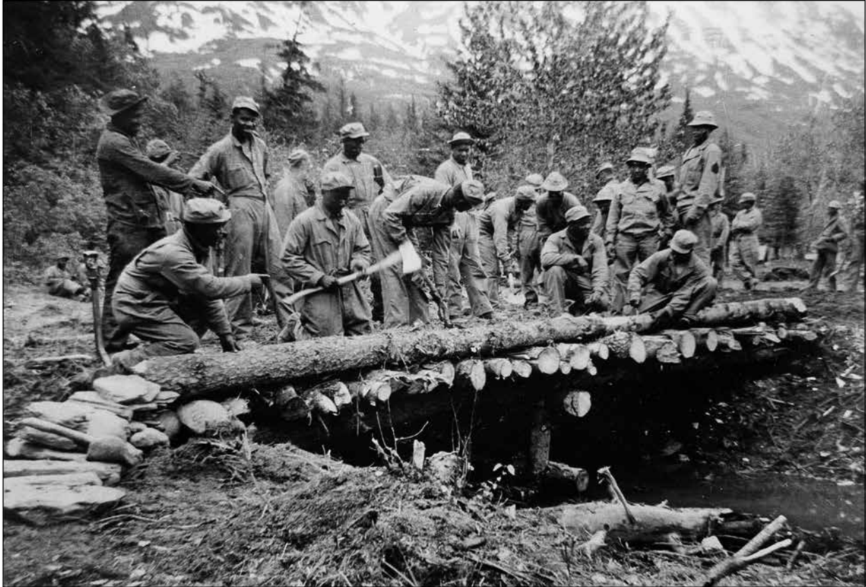
Figure 35. Walter Mason's A Company 97th Engineer Regiment building a pioneer bridge. Photo by Walter E. Mason. Lael Morgan Collection, UAF-2012-71-351. Archives, Elmer E. Rasmuson Library, University of Alaska Fairbanks.
