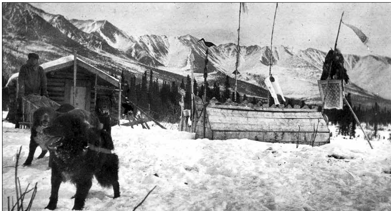
Figure 14. Cross Creek Village, c. 1915, showing “spirit houses” constructed above graves. Lewis V. Stanley Collection, Tacoma Public Library.
