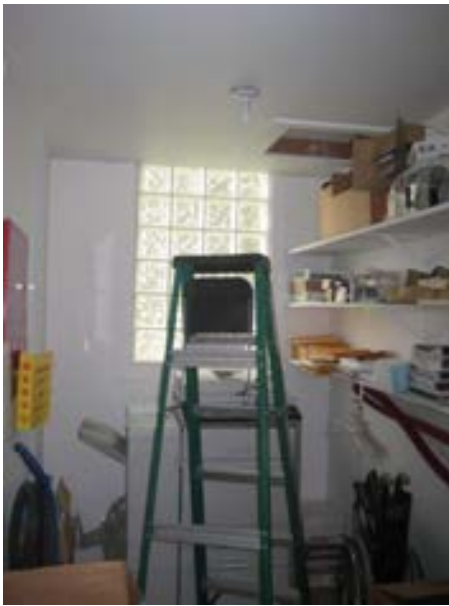
FIGURE 328. Glass block window in storage (room 107) on the south wall. Photograph by BVH, October 16, 2012.
