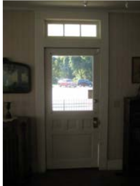
FIGURE 93. Front door of the house looking west. Photograph by BVH, October 16, 2012.
