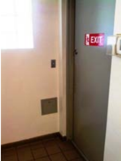
FIGURE 468. Wall access door for shut-off valve at west wall of men's restroom. Photograph by Alvine, May 15, 2013.
