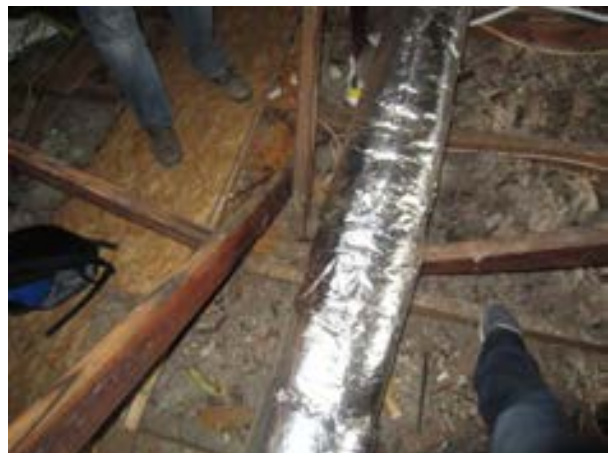
FIGURE 190. Bearing conditions of cross-bracing over the central bearing wall in the north-south and east-west conditions, view looking south. Photograph by WJE, October 16, 2012.
