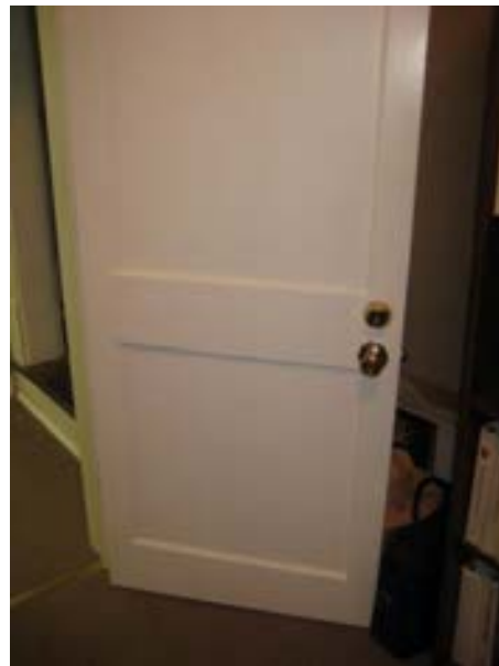
FIGURE 321. Corridor door on the north wall of the superintendent office. Photograph by BVH, October 16, 2012.
