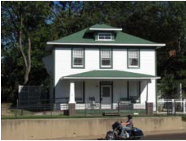
FIGURE 66. The west elevation of the Cassidy House. Photograph by WJE, October 15, 2012.
