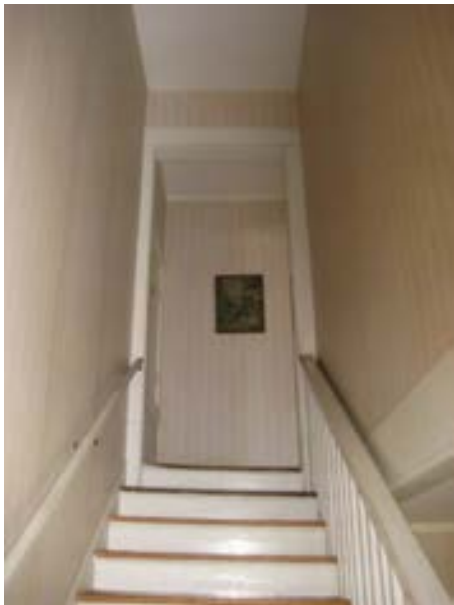
FIGURE 103. Upper run of stairs with original rail at right, and added safety rail at left, looking east. Photograph by BVH, October 16, 2012.
