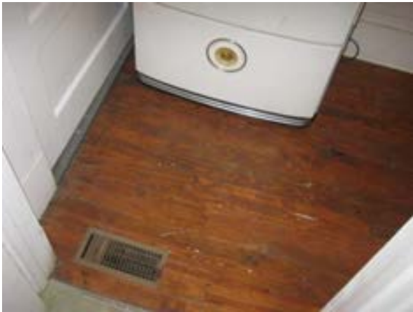
FIGURE 135. Floor of the back porch looking east. Photograph by BVH, October 16, 2012.
