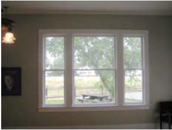
FIGURE 292. Triple window assembly on the north side of the room. Photograph by BVH, October 16, 2012.
