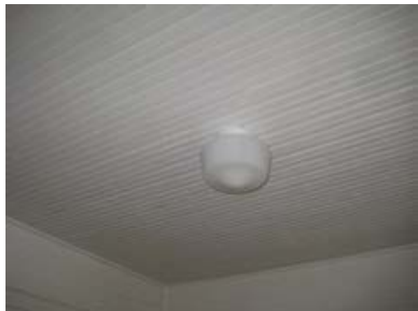
FIGURE 125. Tongue-and-groove kitchen ceiling. Photograph by BVH, October 16, 2012.
