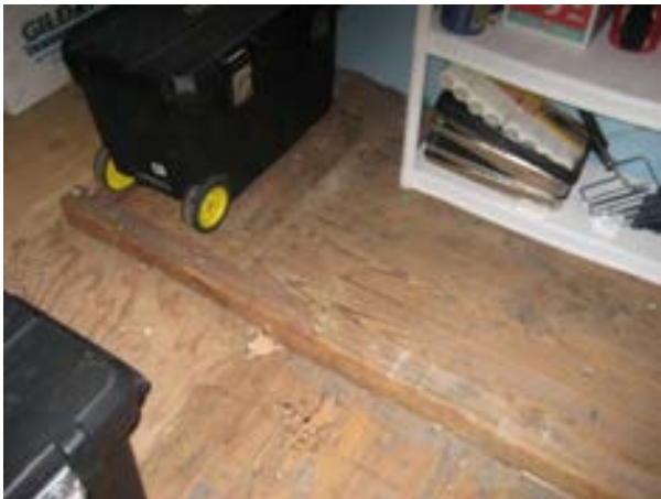
FIGURE 356. Plywood floor, facing south in room 203. Photograph by BVH, October 16, 2012.
