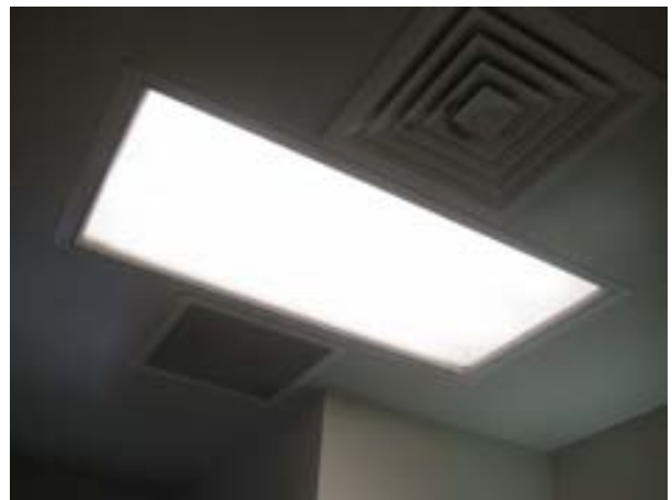
FIGURE 442. ceiling of the men's room looking west. Photograph by BVH, October 16, 2012.
