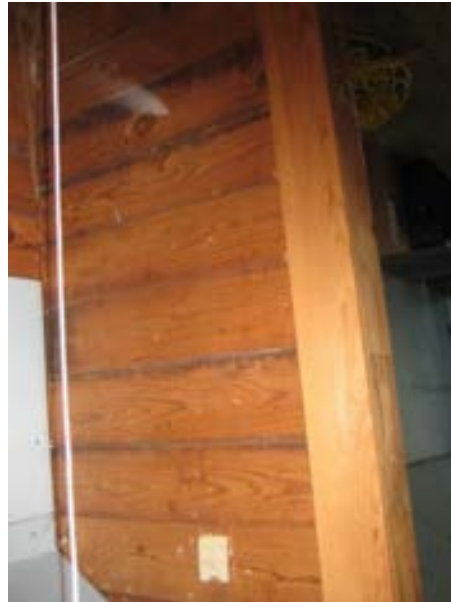
FIGURE 357. Horizontal half-lap wall boards, facing west. Photograph by BVH, October 16, 2012.
