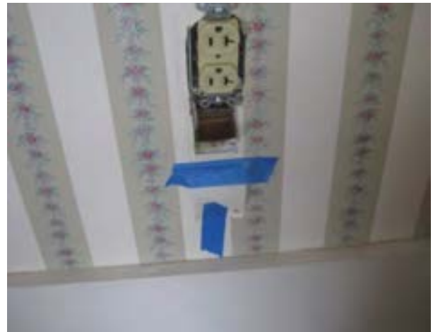
FIGURE 159. Material assembly of wall construction, showing the horizontals half-lap wood wall boards behind the gypsum board, located south of the door on the east wall. Photograph by BVH, October 16, 2012.
