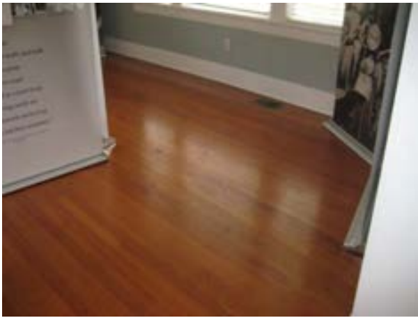
FIGURE 295. Hardwood floor of the exhibit room, looking north. Photograph by BVH, October 16, 2012.
