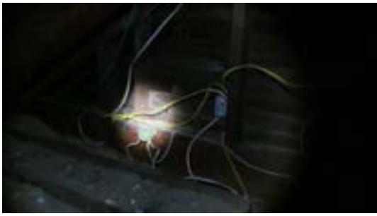
FIGURE 399. Electrical wiring in attic with incorrectly routed and unsupported cables. Photograph by Alvine, May 15, 2013.
