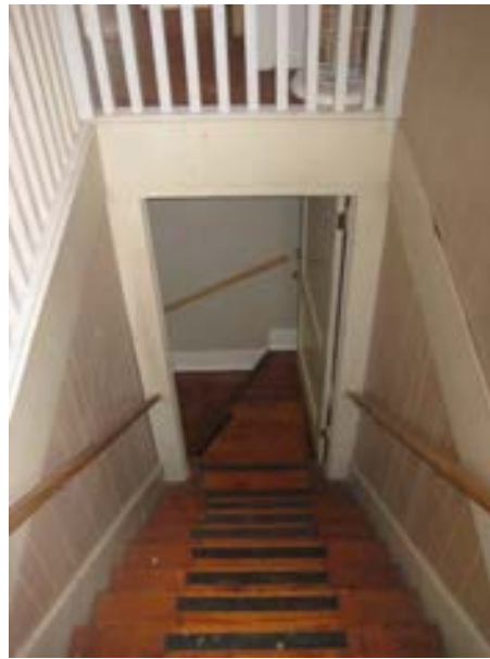
FIGURE 343. The panel door located at the intermediate landing of the stairs, looking north. Photograph by BVH, October 16, 2012.
