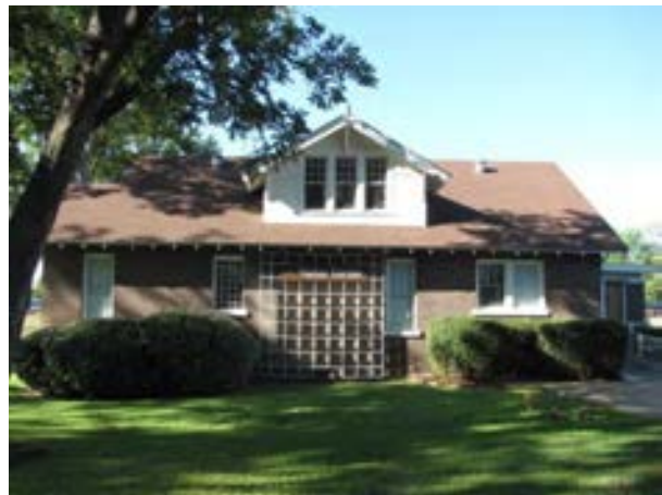
FIGURE 263. A view of the south elevation of the visitor center. The enclosed porch can be seen on the far right. Photograph by WJE, October 15, 2012.
