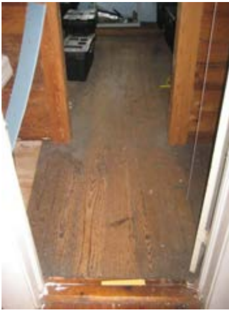
FIGURE 355. Tongue-and-groove flooring, facing west. Photograph by BVH, October 16, 2012.
