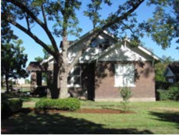
FIGURE 267. A view of the west elevation of the visitor center. The projecting bay can be seen on the right. Photograph by WJE, October 15, 2012.
