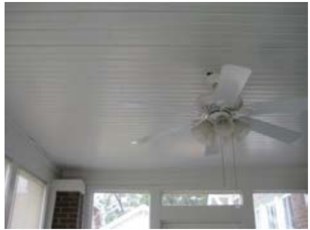
FIGURE 280. Tongue-and-groove ceiling with ceiling fan, looking south. Photograph by BVH, October 16, 2012.
