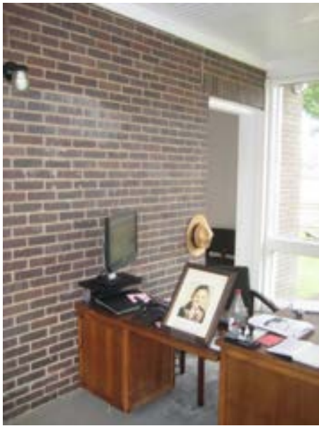
FIGURE 278. The west wall of the entry. The door openings remain but the doors were removed as part of the 1997 work. Photograph by BVH, October 16, 2012.
