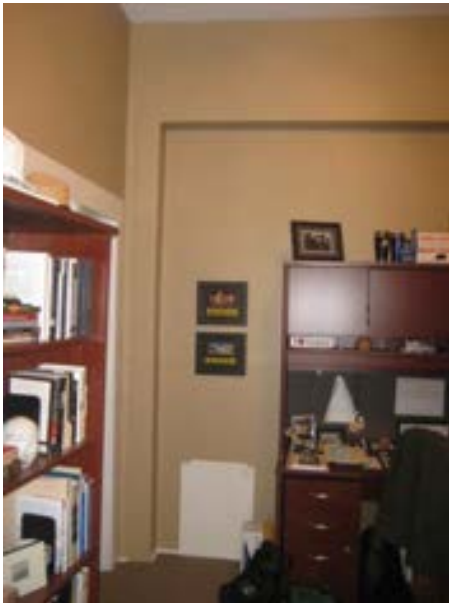
FIGURE 316. The inset portion of the wall is new construction, where the breakfast room once protruded from the south end of the house. Photograph by BVH, October 16, 2012.
