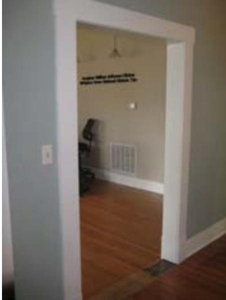
FIGURE 300. East wall door opening between the reception and exhibit spaces. The door was removed and the opening was widened as part of the 1997 work. Photograph by BVH, October 16, 2012.
