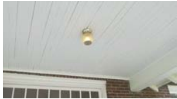
FIGURE 406. Front porch lighting fixture. Photograph by Alvine, May 15, 2013.
