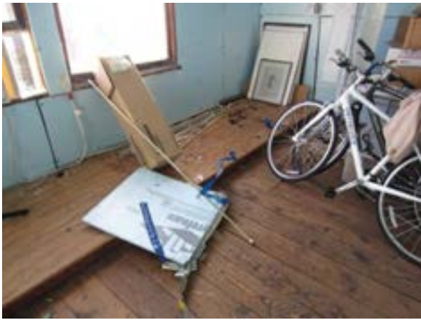
FIGURE 371. Plywood platform framed out at the east end of the second floor, view looking southeast. Photograph by WJE, October 17, 2012.
