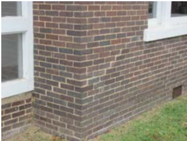
FIGURE 270. An example of stepped cracking at the northeast corner of the building. Photograph by WJE, October 16, 2012.
