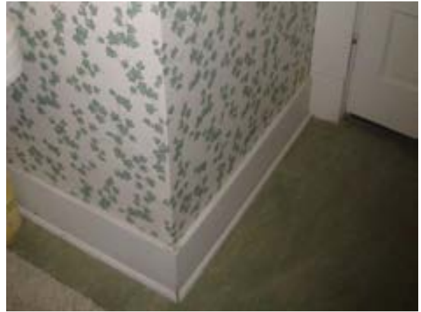
FIGURE 153. Bathroom walls with wall base, looking south. Photograph by BVH, October 16, 2012.
