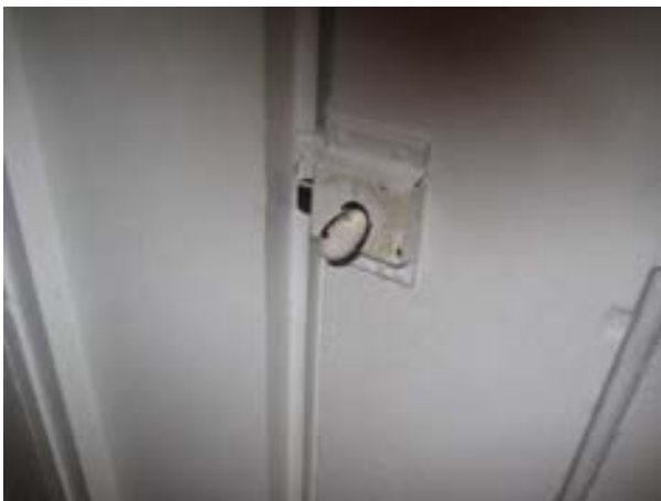
FIGURE 179. Spring-loaded latch of the linen closet door. Photograph by BVH, October 16, 2012.
