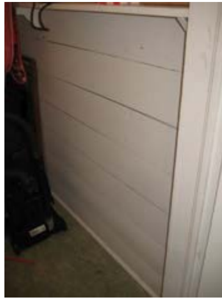
FIGURE 133. Wall assembly in the pantry, looking north. Photograph by BVH, October 16, 2012.
