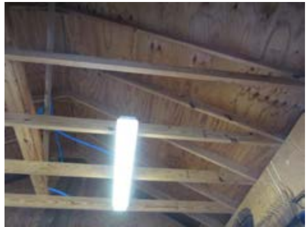
FIGURE 445. Typical 2x6 roof framing. Looking south. Photograph by WJE, October 17, 2012.
