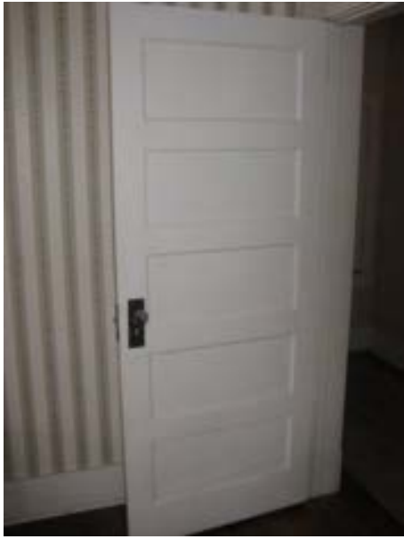
FIGURE 164. Bedroom 204 door on the east wall of the room. Photograph by BVH, October 16, 2012.
