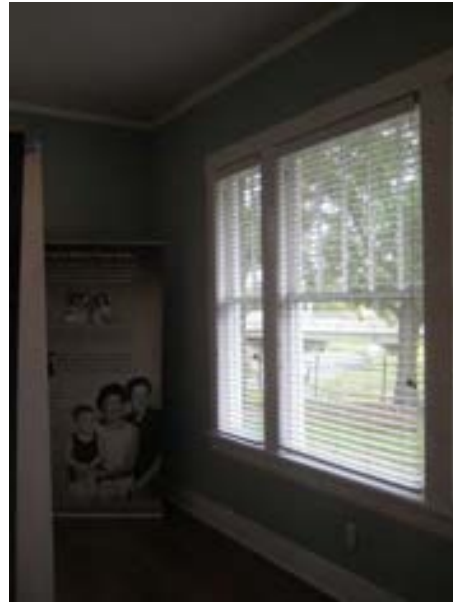
FIGURE 301. Triple window assembly on the north side of the room. Photograph by BVH, October 16, 2012.
