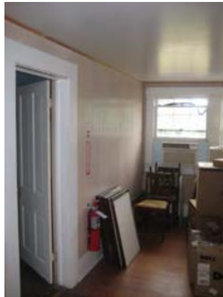
FIGURE 341. Wood veneer paneling, looking north. Photograph by BVH, October 16, 2012.
