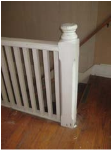
FIGURE 338. Railing and newel post looking east. Photograph by BVH, October 16, 2012.
