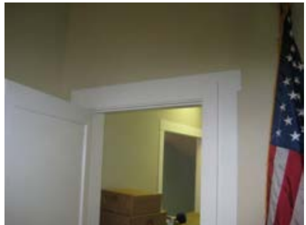
FIGURE 334. Double door frame, looking northeast. Photograph by BVH, October 16, 2012.
