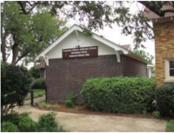
FIGURE 419. The south elevation of the comfort station. Photograph by WJE, October 16, 2012.
