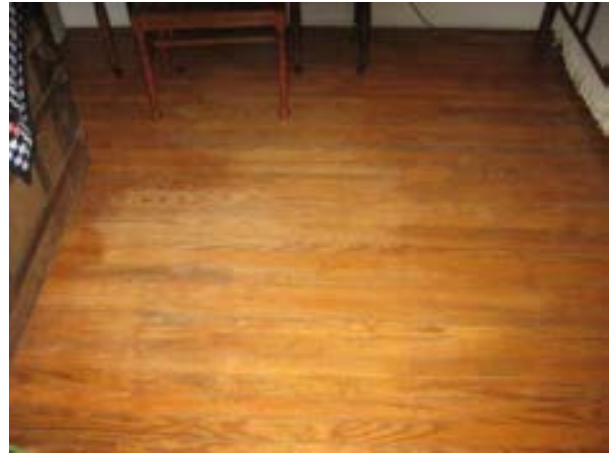
FIGURE 166. Floor of bedroom 205, looking east. Photograph by BVH, October 16, 2012.
