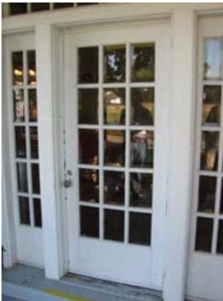
FIGURE 255. View of the door leading from the north porch to the visitor center. Photograph by WJE, October 15, 2012.
