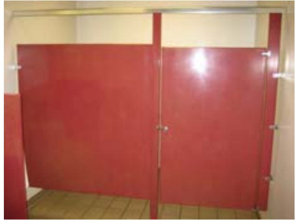
FIGURE 437. Men's room accessible water closet, looking east. Photograph by BVH, October 16, 2012.
