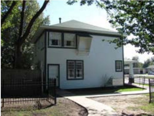
FIGURE 70. The north elevation of the Cassidy House. Photograph by WJE, October 15, 2012.
