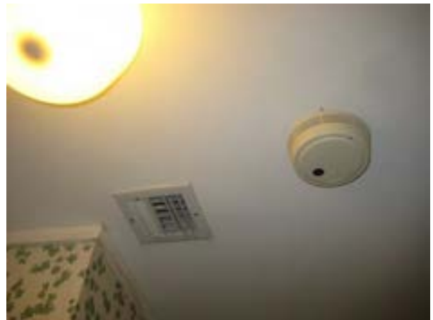
FIGURE 154. Ceiling and light fixture in the bathroom. Photograph by BVH, October 16, 2012.
