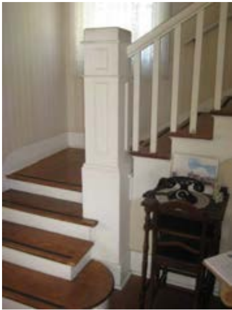
FIGURE 102. Newel post and lower run of stairs, looking north. Photograph by BVH, October 16, 2012.
