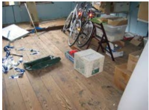
FIGURE 348. Face nailed softwood tongue-and-groove flooring of east storage (room 202), facing east. Photograph by BVH, October 16, 2012.
