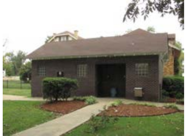
FIGURE 420. A view of the west elevation of the comfort station. Photograph by WJE, October 16, 2012.
