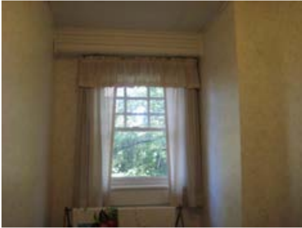
FIGURE 116. The nine-over-one window located on the east wall of the hallway. Photograph by BVH, October 16, 2012.
