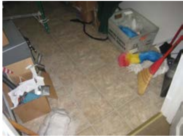
FIGURE 324. Vinyl flooring in storage (room 107) looking south. Photograph by BVH, October 16, 2012.
