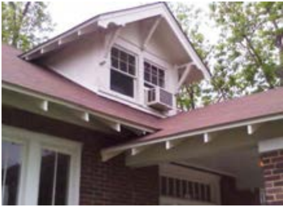
FIGURE 390. Window air conditioner at north/south center storage room 201 of the second floor of the visitor center. Photograph by Alvine, May 15, 2013.
