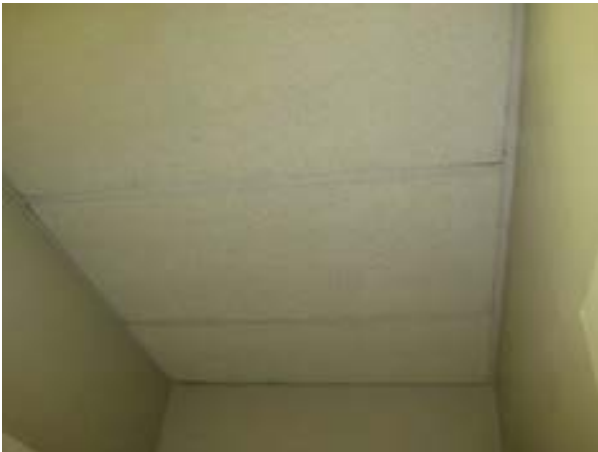
FIGURE 313. Suspended ceiling in the corridor looking west. Photograph by BVH, October 16, 2012.
