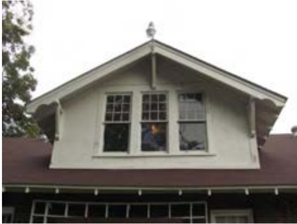
FIGURE 265. A view of the gabled dormer on the south elevation. Photograph by WJE, October 16, 2012.
