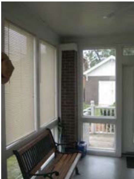
FIGURE 279. Corner brick pier at the southeast corner of the entry. Photograph by BVH, October 16, 2012.
