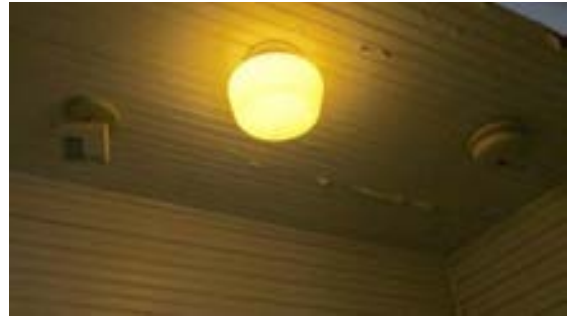
FIGURE 244. Cassidy House back porch 106 lighting fixture. Photograph by Alvine, May 15, 2013.
