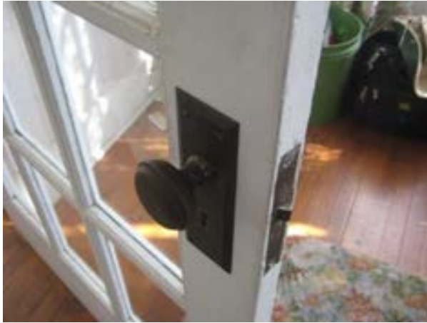
FIGURE 97. Hardware of the north French door. Photograph by BVH, October 16, 2012.
