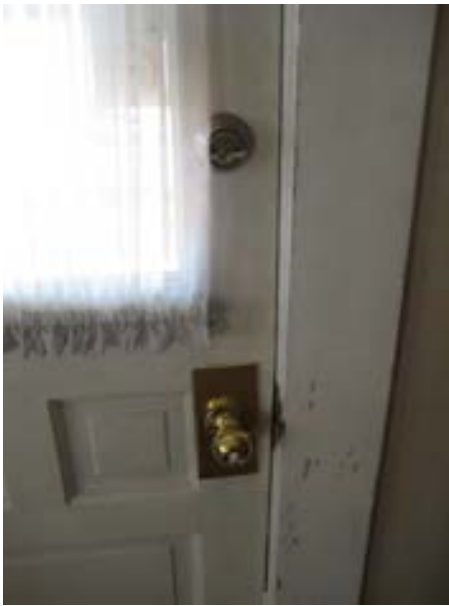
FIGURE 94. Front door hardware. Photograph by BVH, October 16, 2012.
