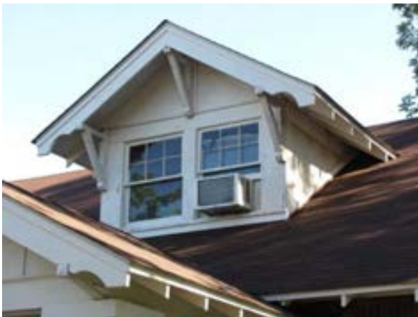
FIGURE 256. A view of the north dormer. Photograph by WJE, October 15, 2012.
