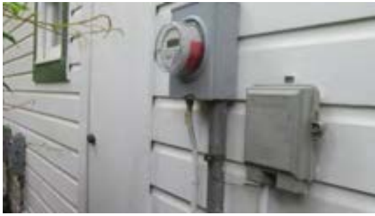
FIGURE 235. Cassidy House electric meter and telephone. DeMark service entrance. Photograph by Alvine, May 15, 2013.
