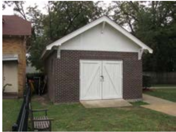
FIGURE 418. The north elevation of the comfort station. Photograph by WJE, October 16, 2012.
