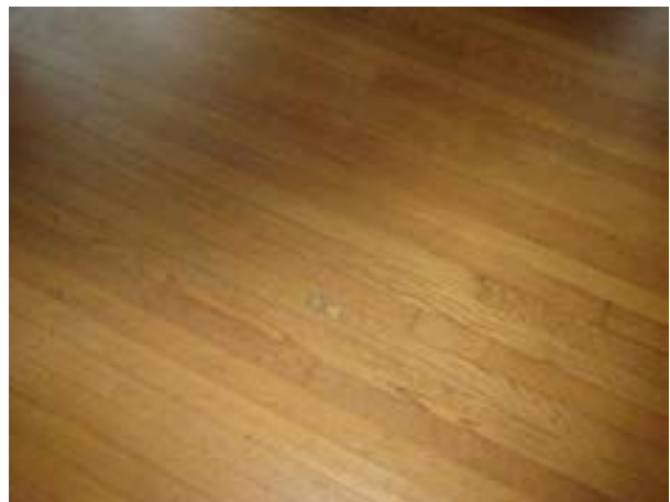
FIGURE 304. Infilled door pin location. Photograph by BVH, October 16, 2012.
