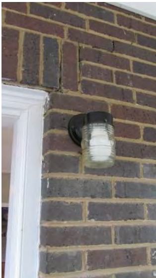
FIGURE 403. Entry 101 wall light. Photograph by Alvine, May 15, 2013.
