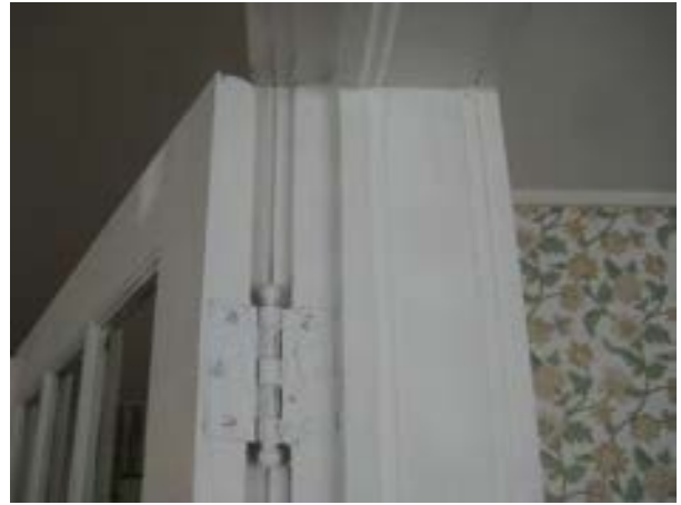
FIGURE 99. Built up layers of wall assembly, looking north. Photograph by BVH, October 16, 2012.
