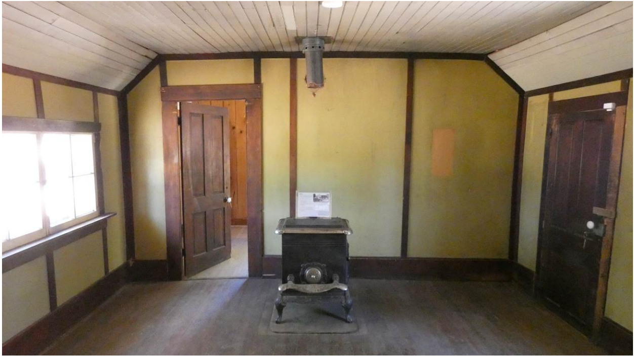
Figure 6. (a) Top, view of Room 3 interior by Paul Beaubien, August 1938, looking northwest. WACA 5530. (b) Bottom, Room 3 as it appeared in 2017, same view. (Photo credit: David E. Purcell).
