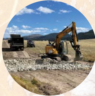
4 miles of pipeline access road reclaimed
