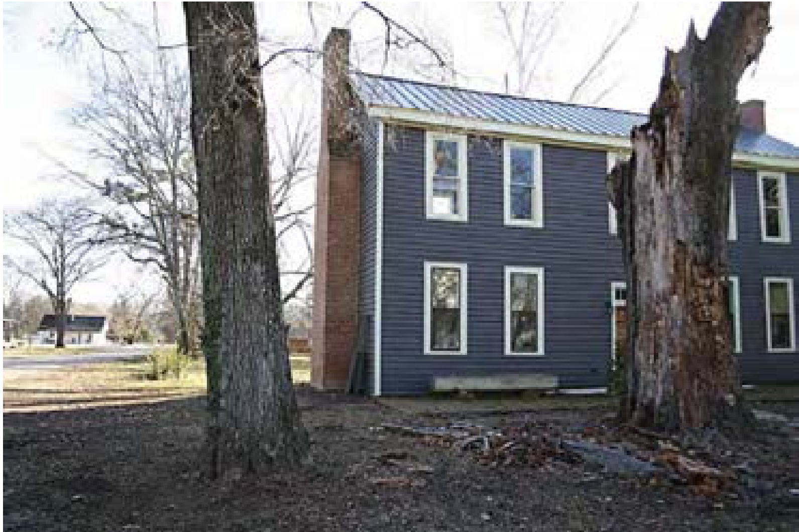
Figure 3.43 Front, north view, of the Harris-Simpson House. In view of the TC&D Railroad. Photo by Marty King.
