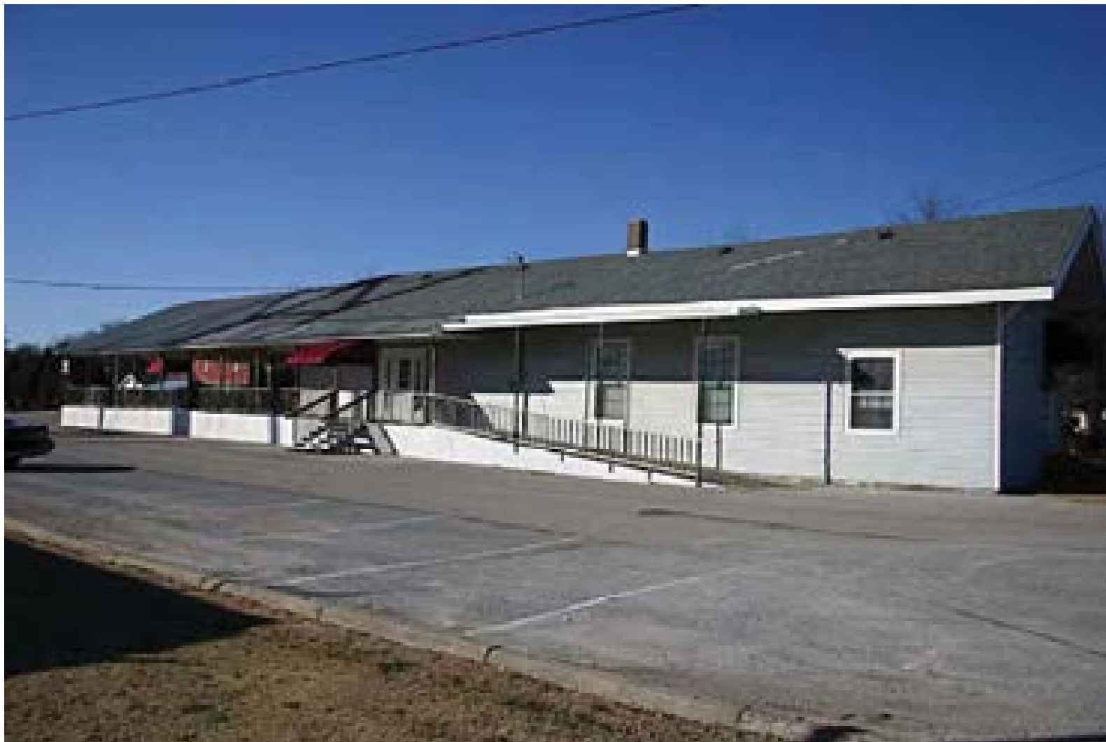
Figure 3.39 Rear view of the Courtland, Alabama Railroad Depot. Photo by Marty King.
