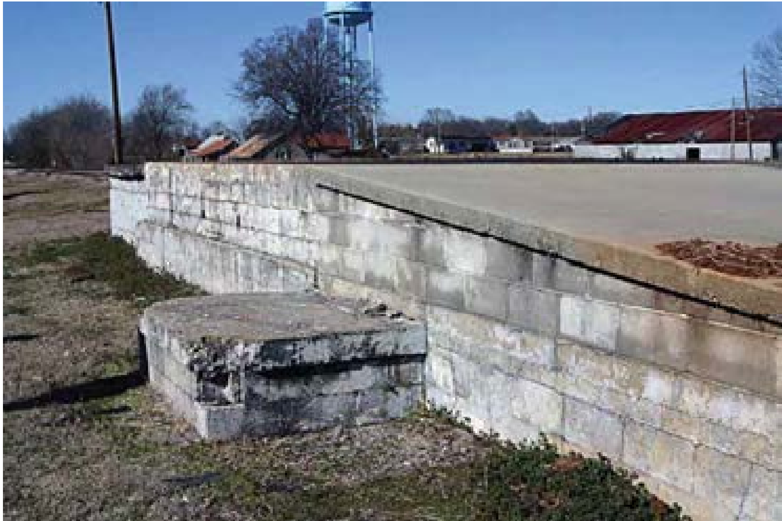
Figure 3.55 The Leighton, Alabama Railroad Depot. Note the foundation is constructed from concrete block which had not been invented in 1832. Photo by Marty King.
