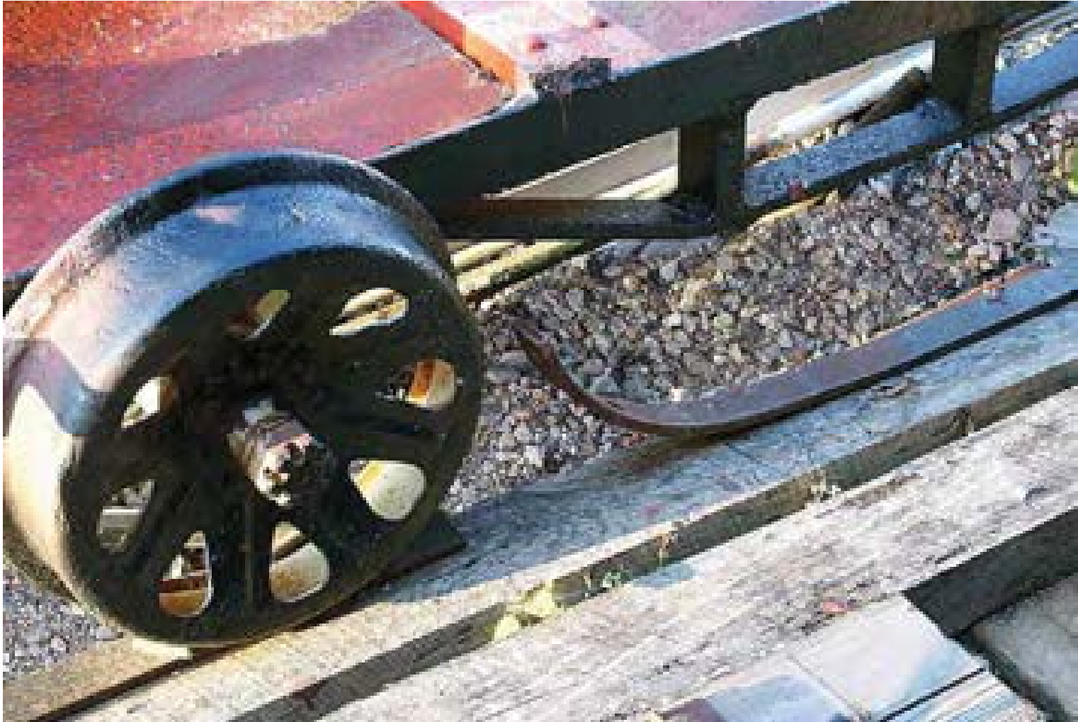
Figure 3.66 Example of 1830's track construction. Note the curved steel. This is called a snake head. If the engineer didn't see it, the wheel of the train would hit it and force it up through the floor of the rail car causing serious bodily injury to the passengers. The first law suit against the railroad was due to such an event. Photo by Marty King.
