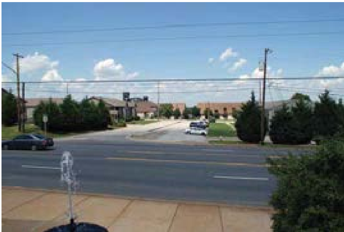
Figure 3.77 Standing where Bank Street ends today the view of the Tennessee River is hidden by the roofs condos. Bank Street went between the two condos seen in the background. Photo by Marty King.
