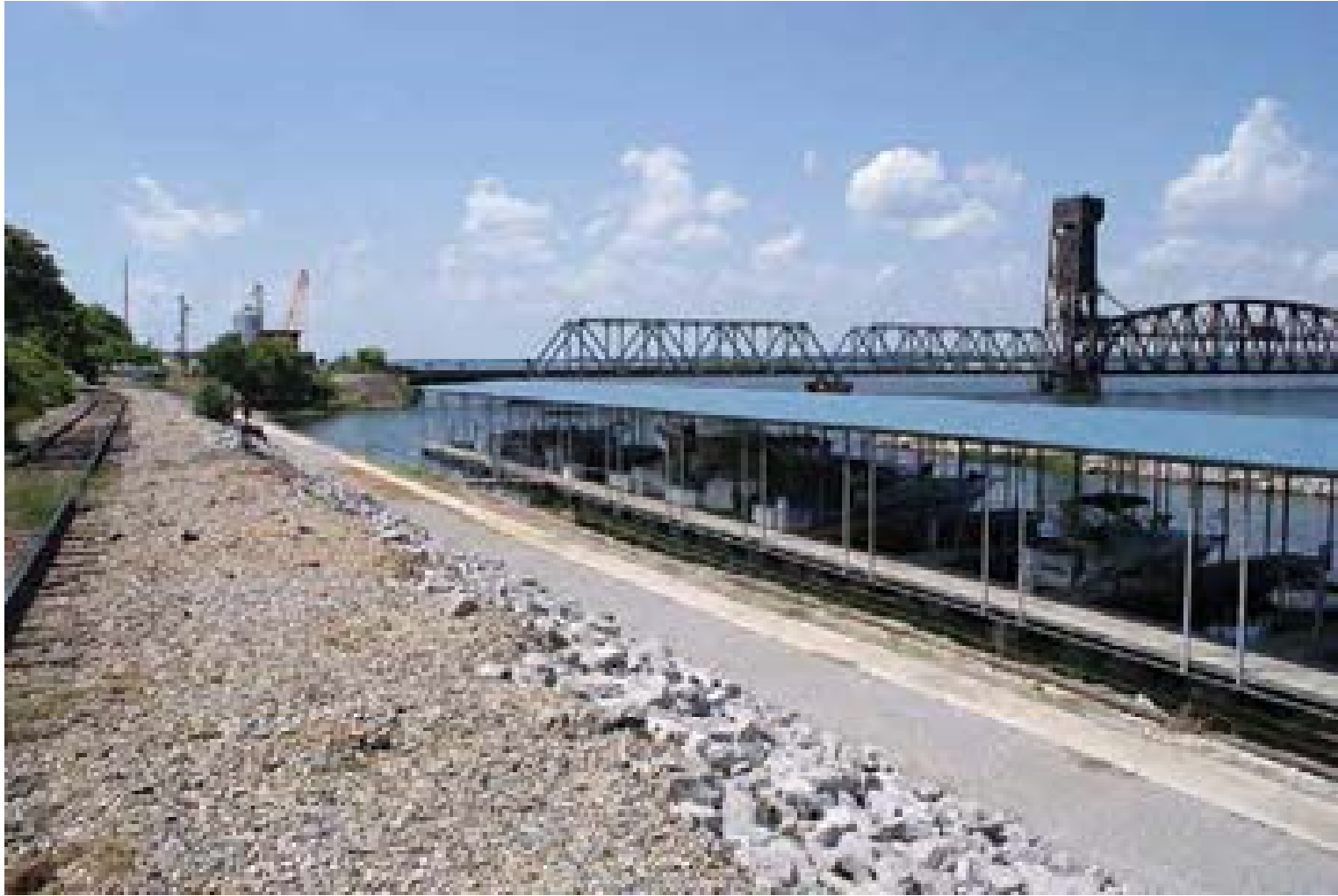
Figure 3.9 This is the location of the Old Steamboat Depot in Decatur Alabama. Note that pleasure boats have replaced the steamboats, and the railroad tracks even now run parallel to the Old Depot location. Photo by Marty King.
