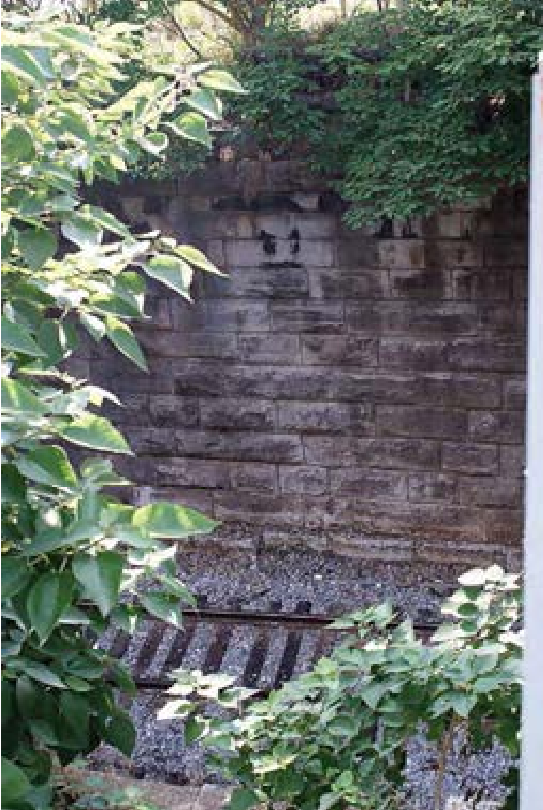
Figure 3.13 “The Cut” in Decatur, Alabama. Photo by Marty King
