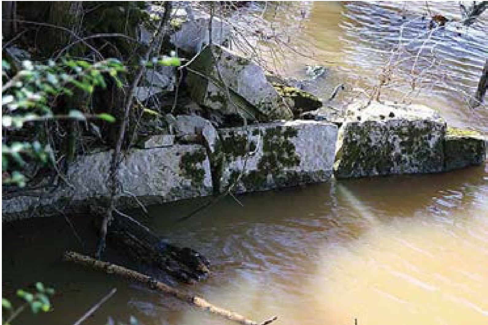
Figure 3.73 Remains of the limestone block steamboat pier at Tuscumbia Landing. Photo by Marty King.
