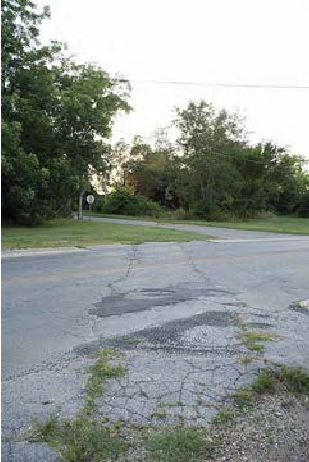
Figure 3.69 Hook Street, Tuscumbia, Alabama. Note the telegraphing of the old rail road bed through the asphalt. Photo by Marty King.
