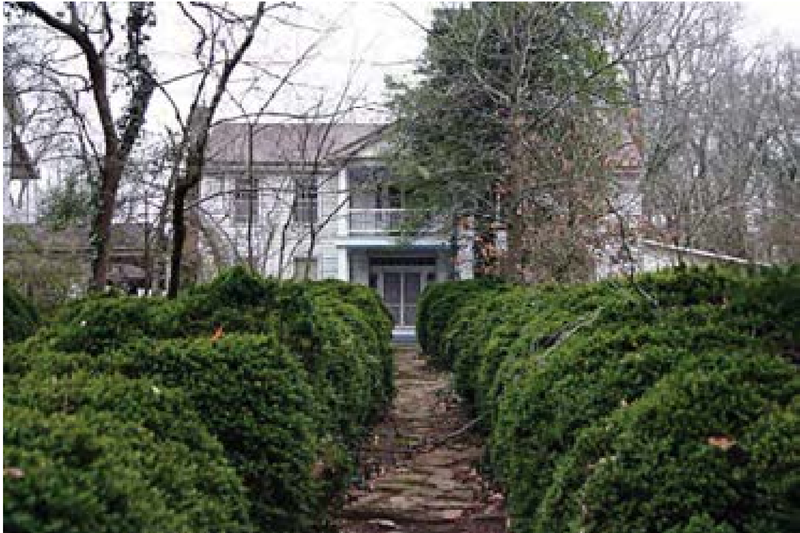
Figure 3.28 The Felix Sherrod (son of Benjamin Sherrod) House, Circa 1818. The house was first constructed as a 1 story log home.. At a latter date a second story was added and the entire structure was covered with wood siding. Adjacent to Wheeler Home. Photo by Marty King.
