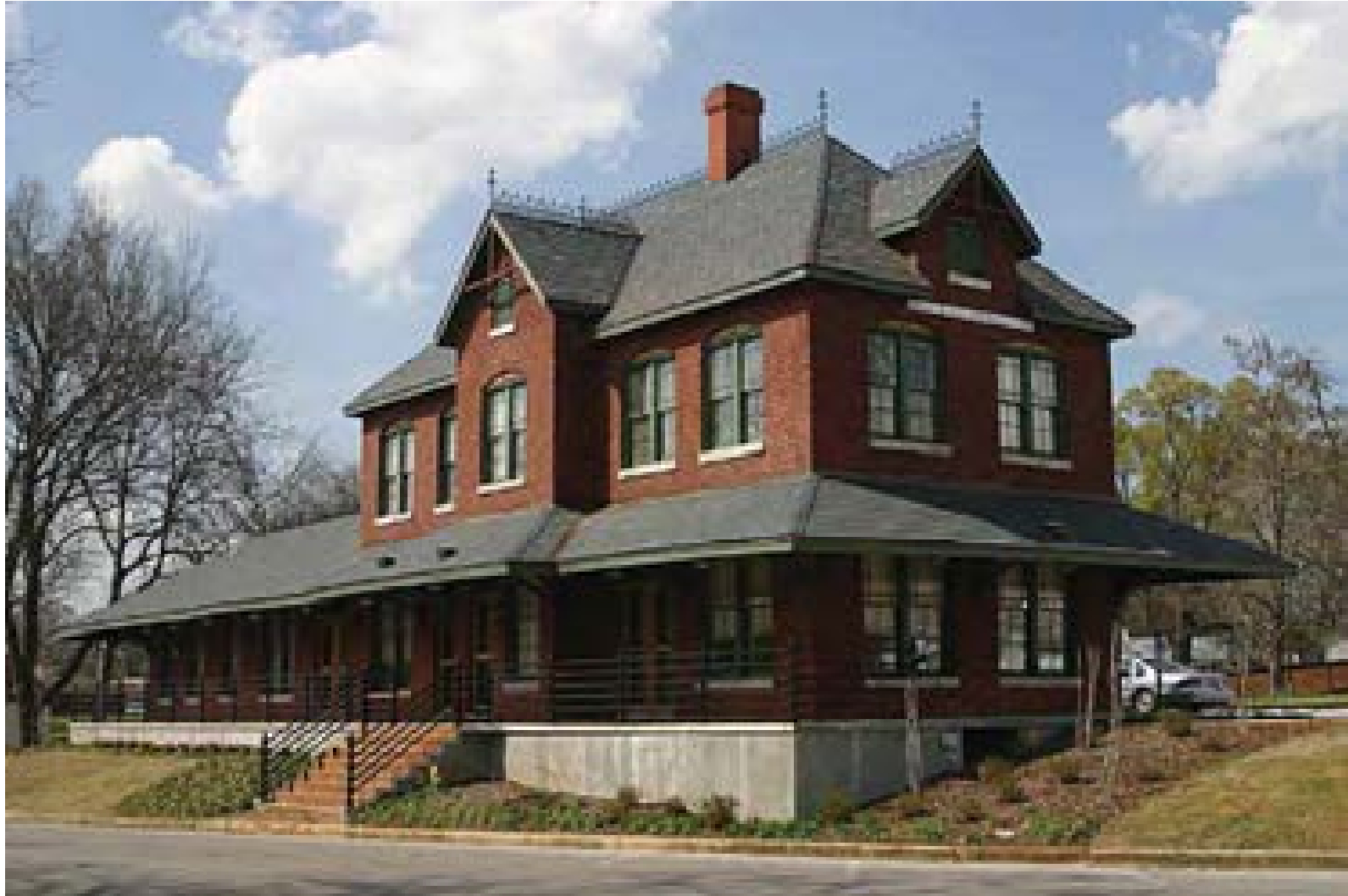
Figure 3.64 Tuscumbia Depot Museum, March 30, 2006. The Old TC&D tracks passed under the silver car seen in the right rear of the museum. This is not the original location of the TC&D Railroad Depot. Photo by Marty King.
