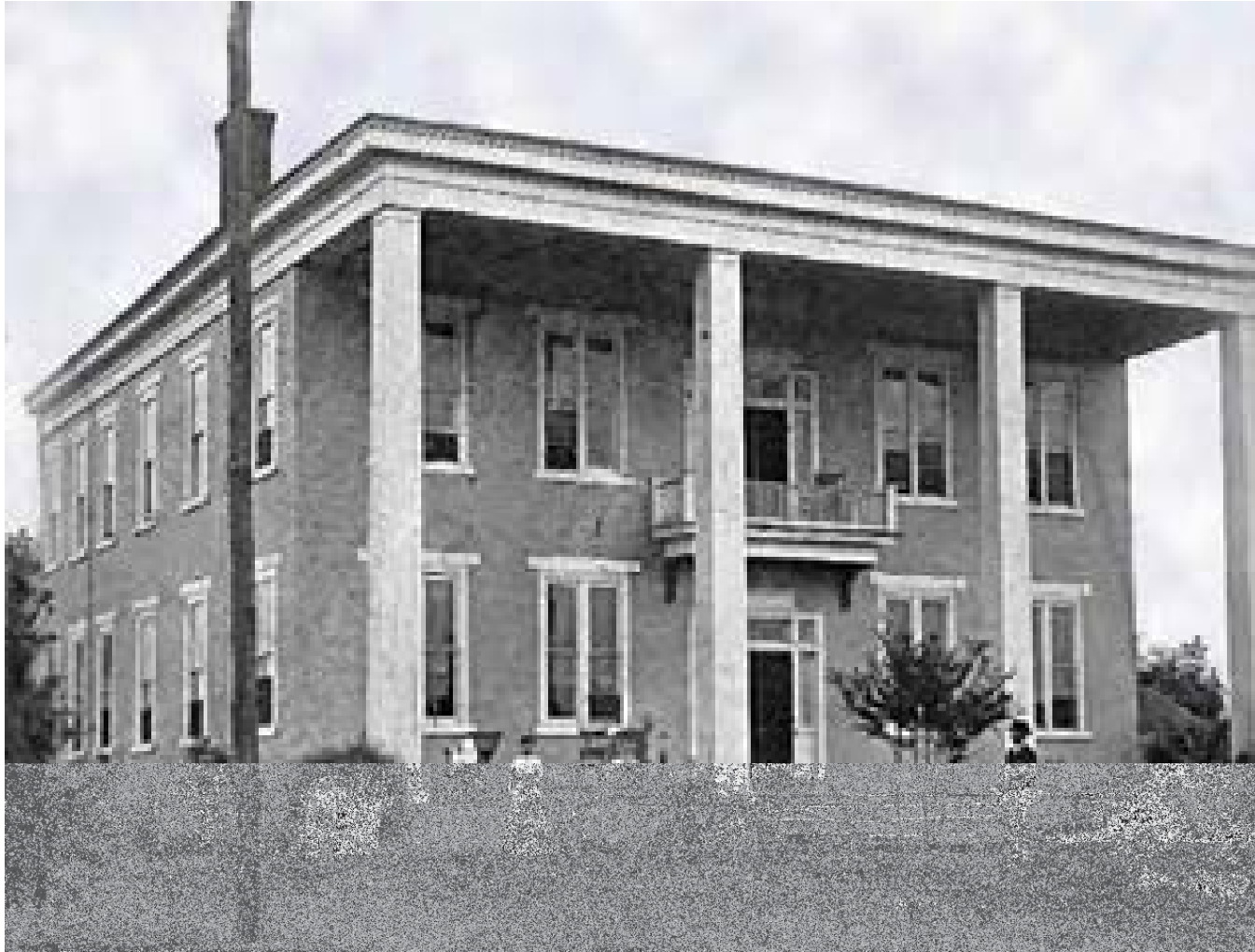
Figure 3.22 Unobstructed view of the Burlison House, Constructed circa 1836, photo circa 1880's. View of TC&D Railroad. Courtesy of the Morgan County Archives. Digitally enhanced by Marty King.
