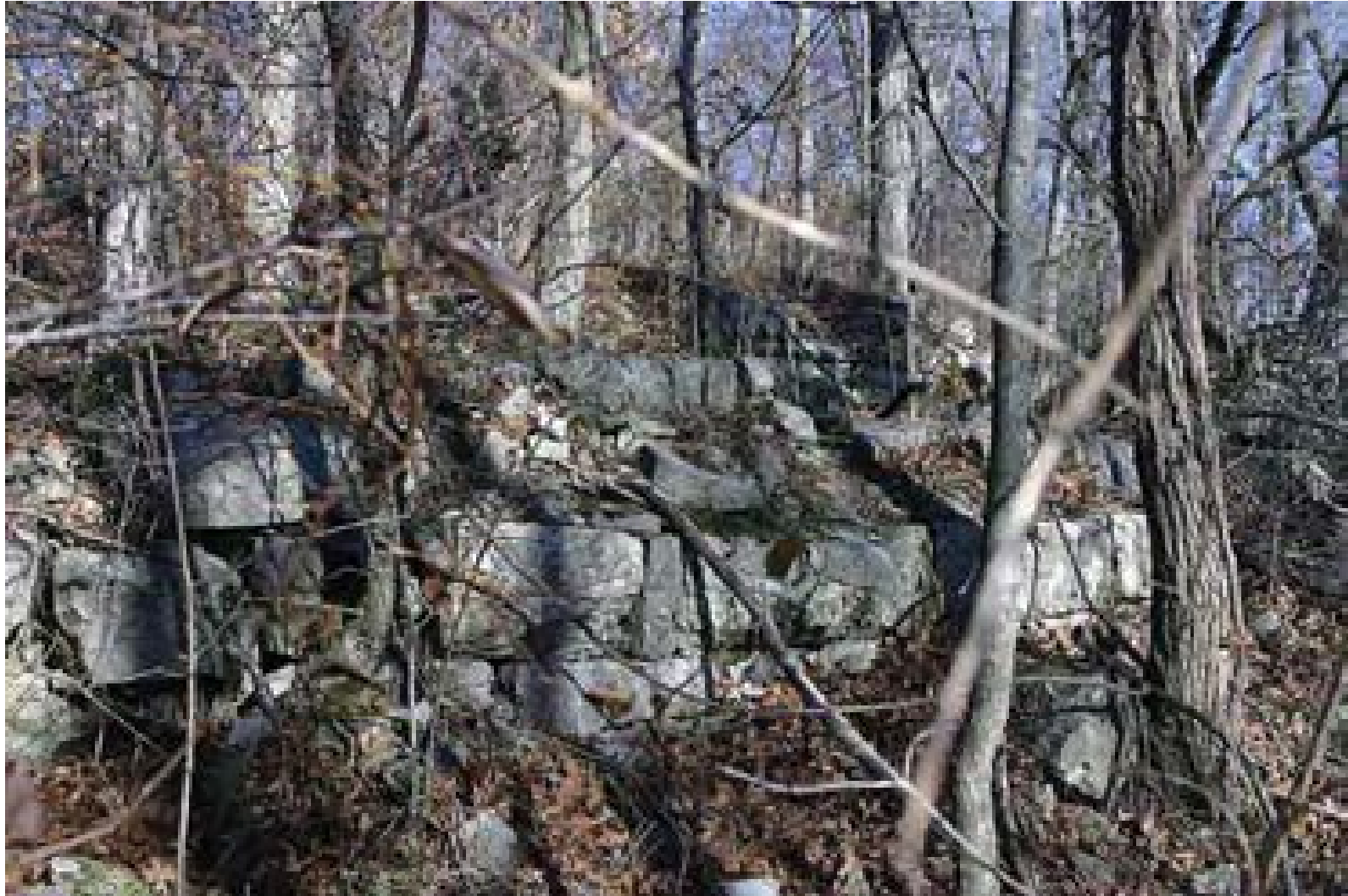
Figure 3.72 Hand cut limestone foundation of the Tuscumbia Courtland and Decatur Rail Road at Tuscumbia Landing. Photo by Marty King.
