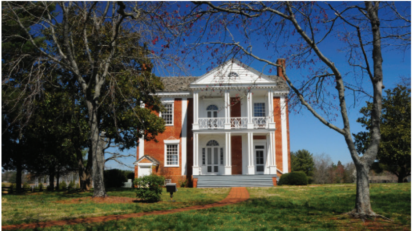
Figure 1. This two-story, Federal-style house was built in Murray County, Georgia, between 1819 and 1823 for Cherokee leader Joseph Vann.
