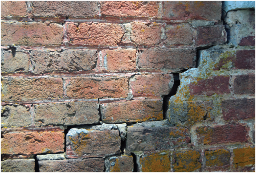
Figure 12. James Brown House, Hamilton County, Tennessee.
