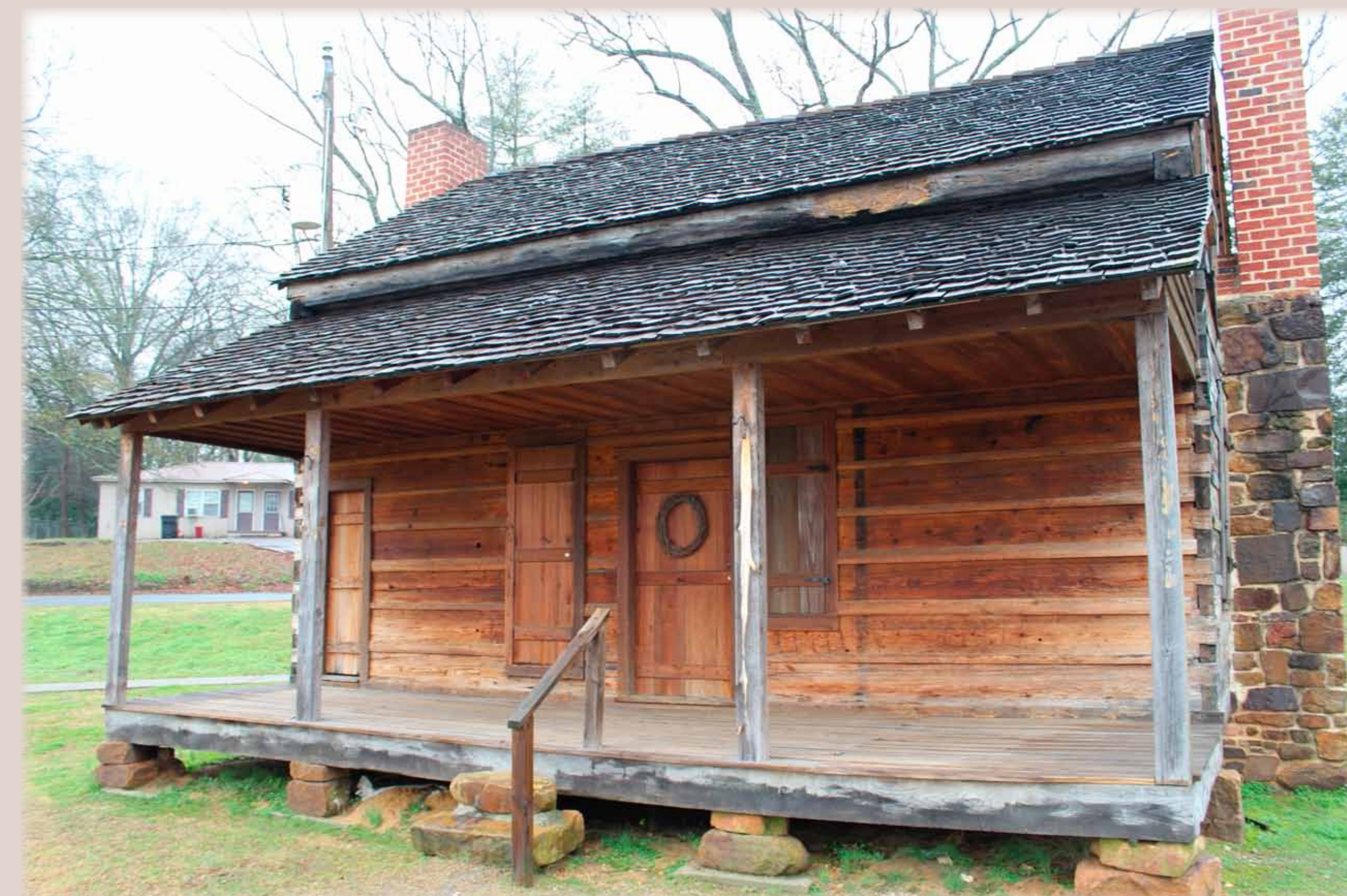
Couey House is representative of the rough hewn log homes built in Dirt Town
