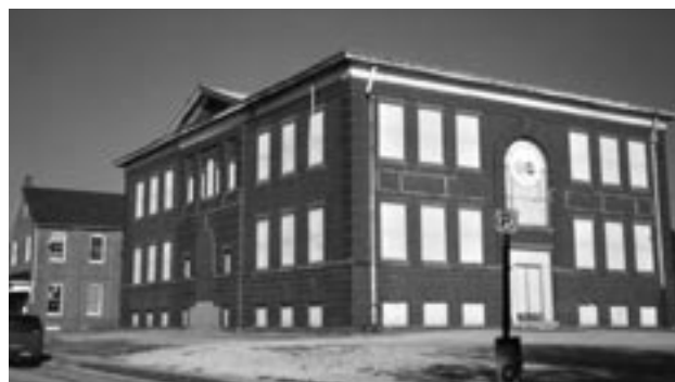
William Shelly School (right) and Annex (left) before rehabilitation. All the original windows remained beneath the plywood.
