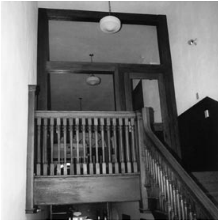
The glass smoke barrier at the top of the stairs is compatible and retains the visual connection between the stairs and the second floor corridor.
