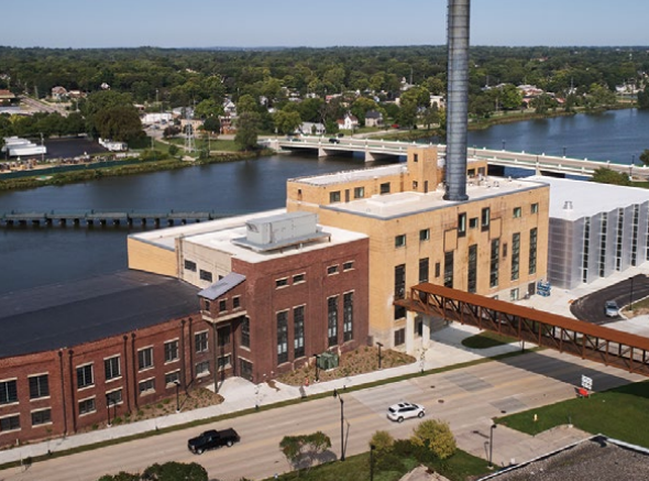
Beloit Water, Gas & Electric Company Powerhouse (below) and former Turbine Hall (right) (1908–1947), now Beloit College Student Union, Beloit, Wisconsin Photos: ©Tom Harris and Studio Gang
