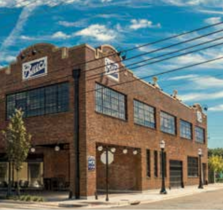
R.J. Reynolds Tobacco Factory Power Plant, Winston-Salem, North Carolina Photo: Triggs Photography
