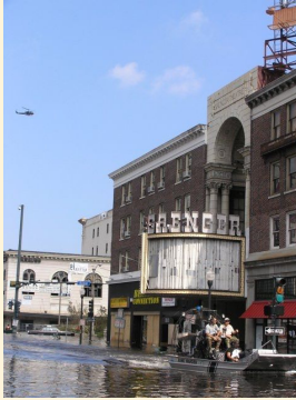
During post-Katrina flooding
