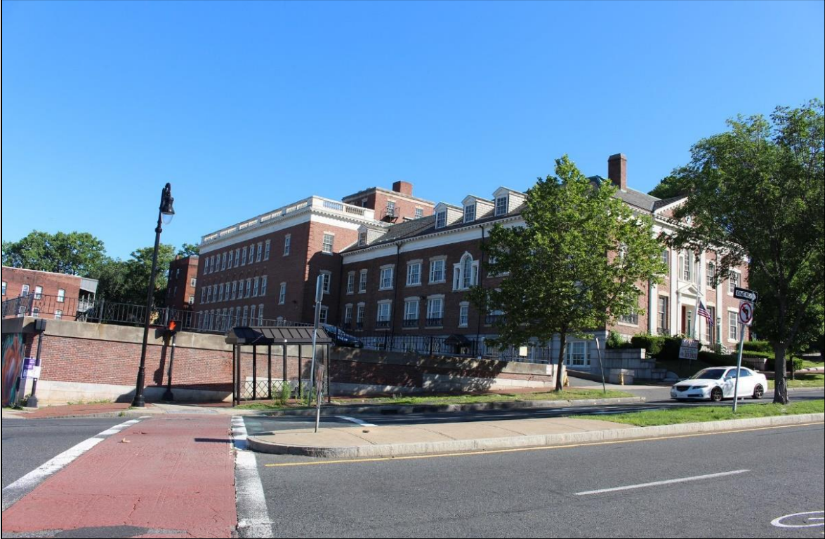
1. South and East Elevations of 1924 Bank Building and 1935 Addition, looking north.
