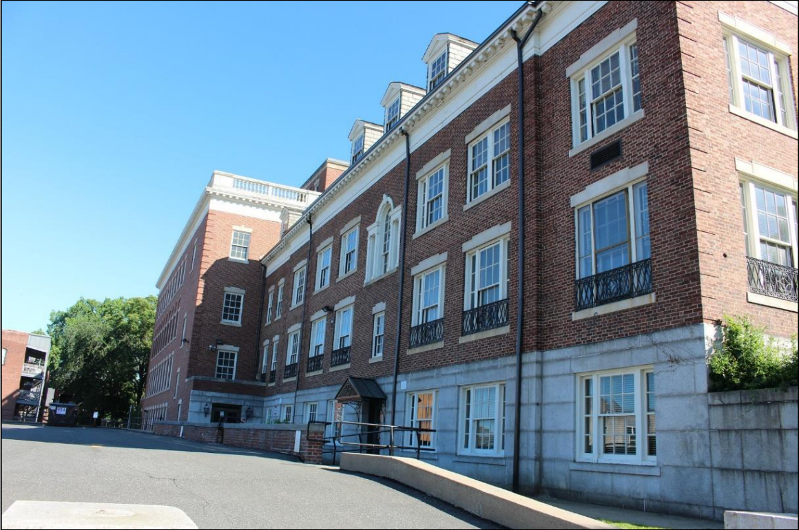
2. South and East Elevation Elevations of 1924 Bank Building and 1935 Addition, looking north.
