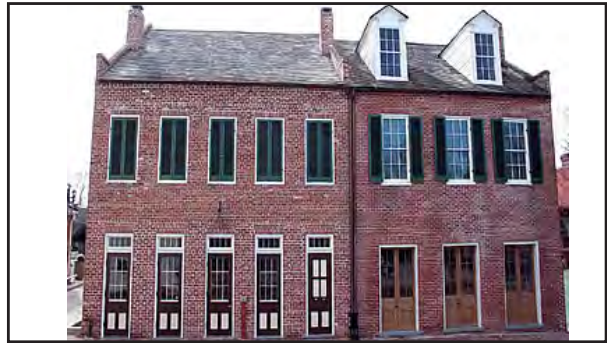
William Johnson constructed this three-story brick structure on his mother-in-law's property after an 1840 tornado destroyed much of downtown Natchez. Courtesy of National Park Service.
