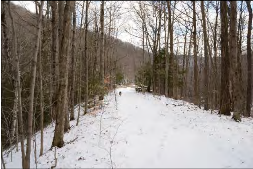
Roadbed, appx. 3,800' long Cuts, fills, retaining wall, signal footings
