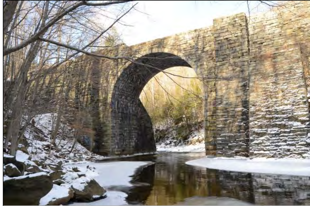
Bridge No. 6, 1840–1844, appx. 550' long, 75' high, 54' span
