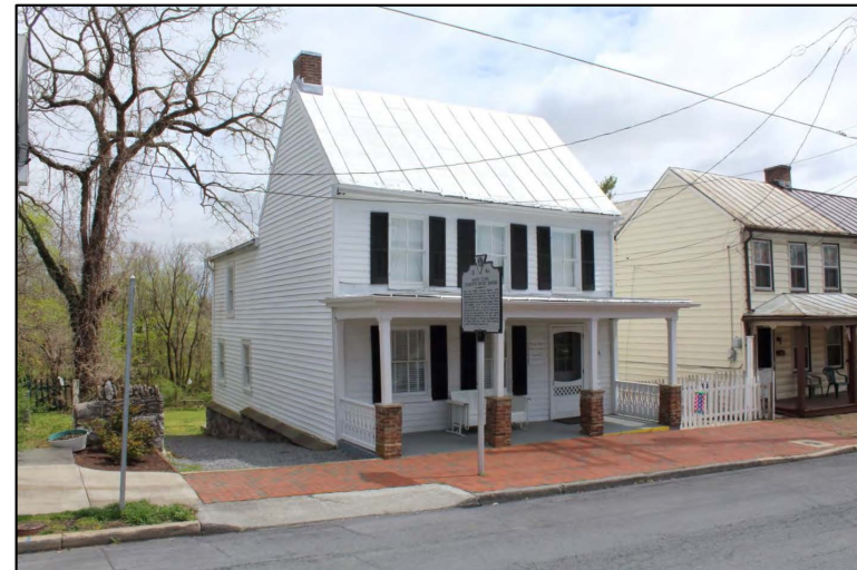
Before and after renovation
