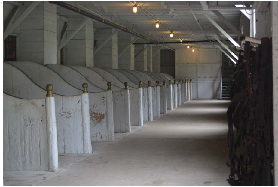
First floor horse stalls, Horse Barn, 2015
