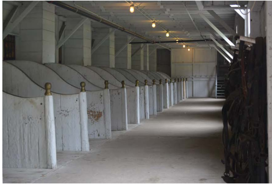
First floor horse stalls, Horse Barn, 2015
