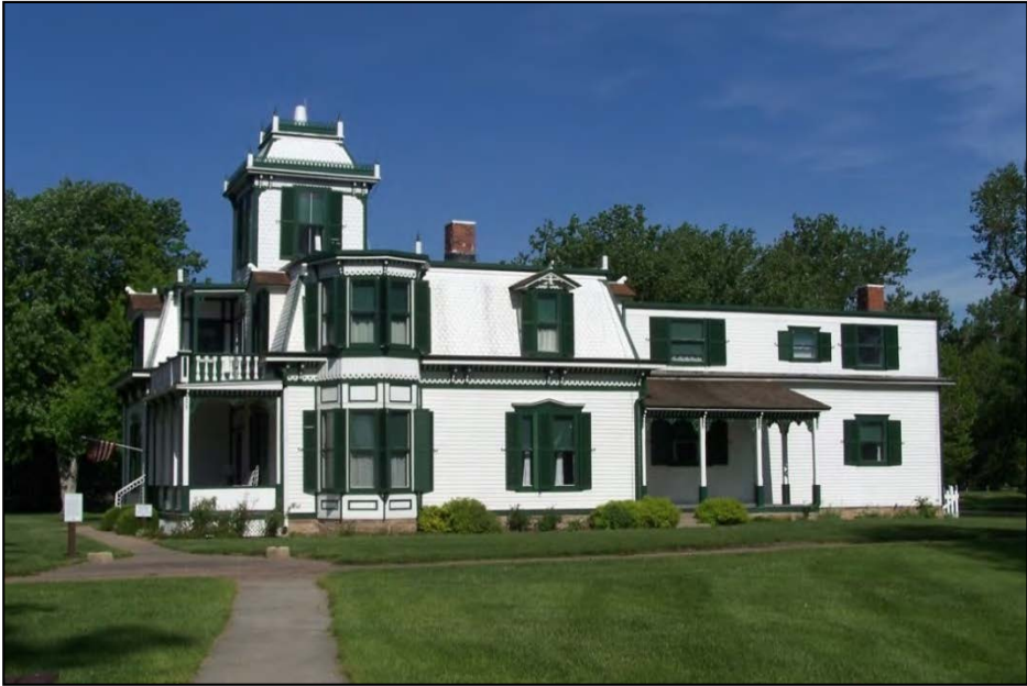
Ranch House, east elevation, 2014
