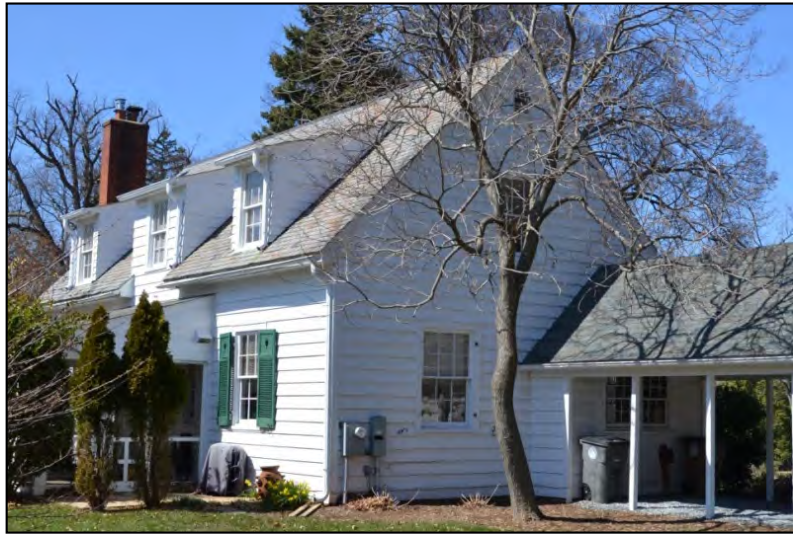
Cottage rear & side
