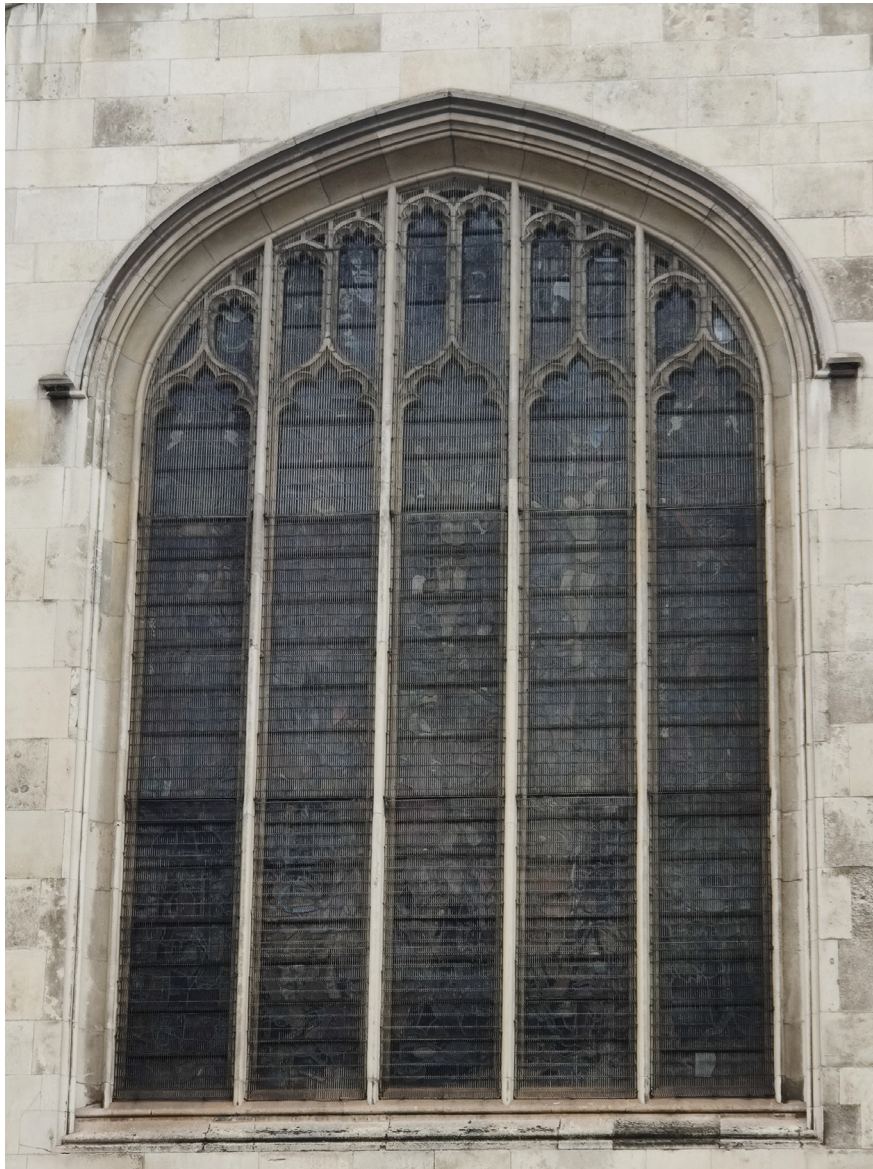
Wire screens provide an alternative to protective glazing. Source: Stéphanie Machabée.
