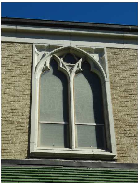
Plastic protective glazing will cloud and yellow over time. Source: Jason Church.
