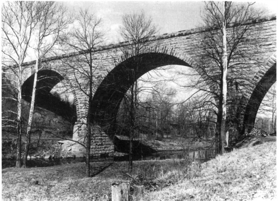
*The Baltimore and Ohio Viaduct over the Black River, near Lodi, Medina County, Ohio, is a monumental masonry civil engineering structure. The photograph shows the timeless simplicity of the stone arched viaduct built in 1892 on the main line of the Baltimore and Ohio, linking Chicago with the East. (Eric Johannesen, 1975)*
