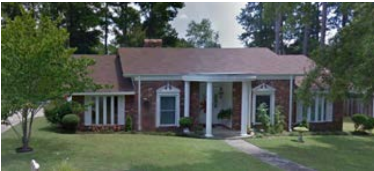
Figure 3: 422 Flowers Street, Fordyce, AR, built between 1965-1983. Note the rounded, one-bay entry porch and the broken pedimented windows on either side of the porch (image from Google Earth taken in 2013; reconnaissance survey by Arkansas Historic Preservation staff in 2022 confirmed the picture is accurate).
