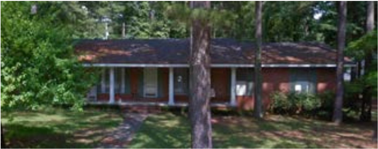
Figure 5: 2001 Pine Forest Lane, constructed between 1965-1983. The house has the same porch detailings as its across-the-street neighbor ( image from Google Earth taken in 2013; reconnaissance survey by Arkansas Historic Preservation staff in 2022 confirmed the picture is accurate ).
