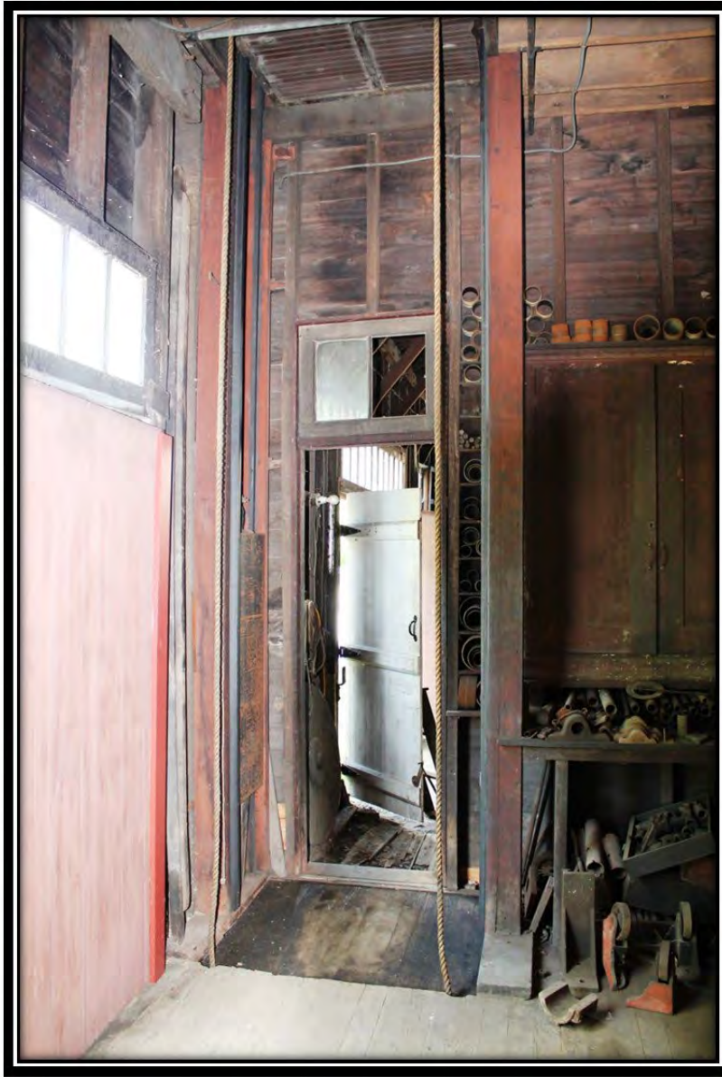
Photograph 22. PA_Greene County_W.A. Young & Sons Foundry and Machine Shop_0022. Hand-operated elevator, facing east.
