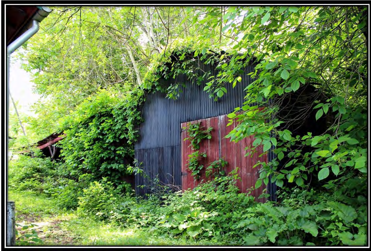
Photograph 37. PA_Greene County_W.A. Young & Sons Foundry and Machine Shop_0037. Oil house and storage shed, facing southeast.
