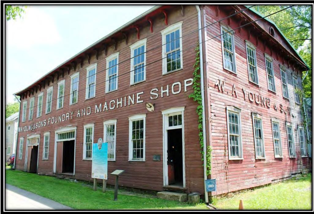
Photograph 1. PA_Greene County_W.A. Young & Sons Foundry and Machine Shop_0001. North (front) and east elevations, facing southeast.
