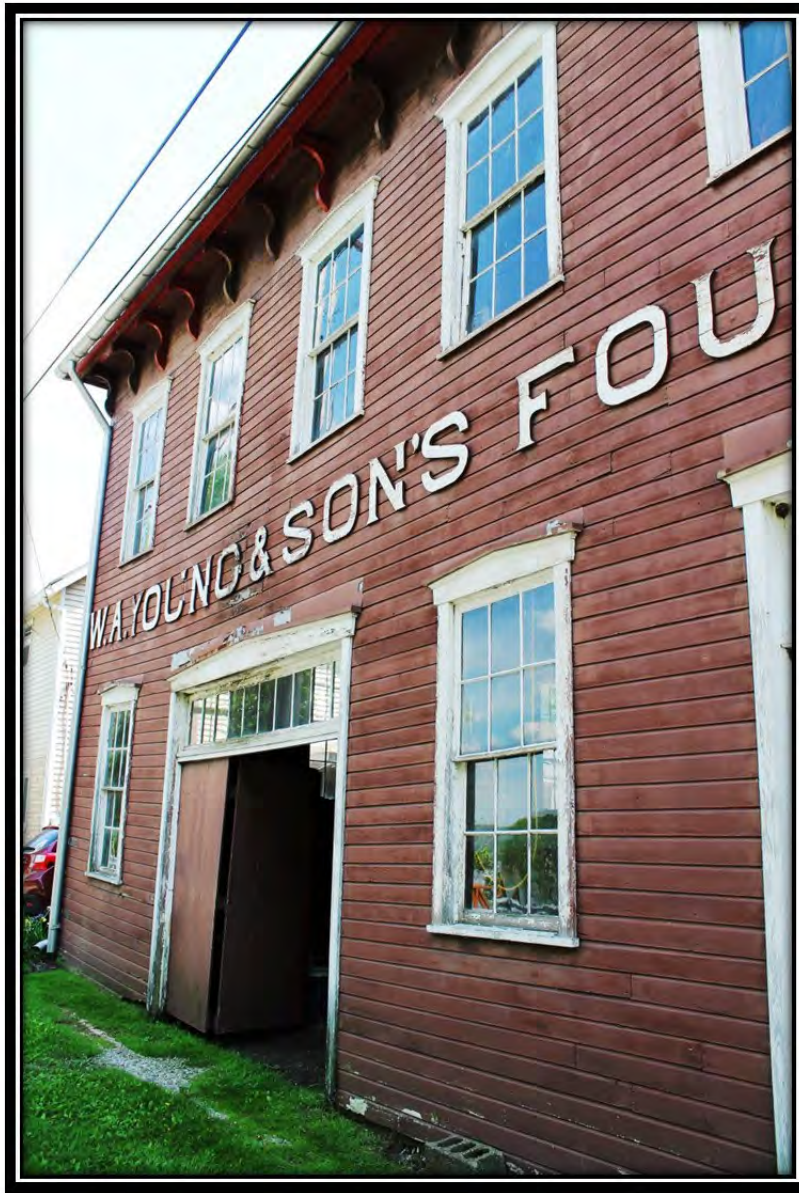
Photograph 4. PA_Greene County_W.A. Young & Sons Foundry and Machine Shop_0004. North (front) elevation of the Foundry, facing southeast.
