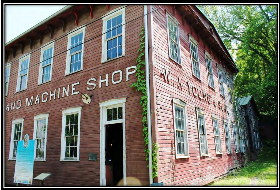
Photograph 3. PA_Green_County_W.A. Young and Sons Foundry and Machine Shop_0003. West Elevation facing south.
