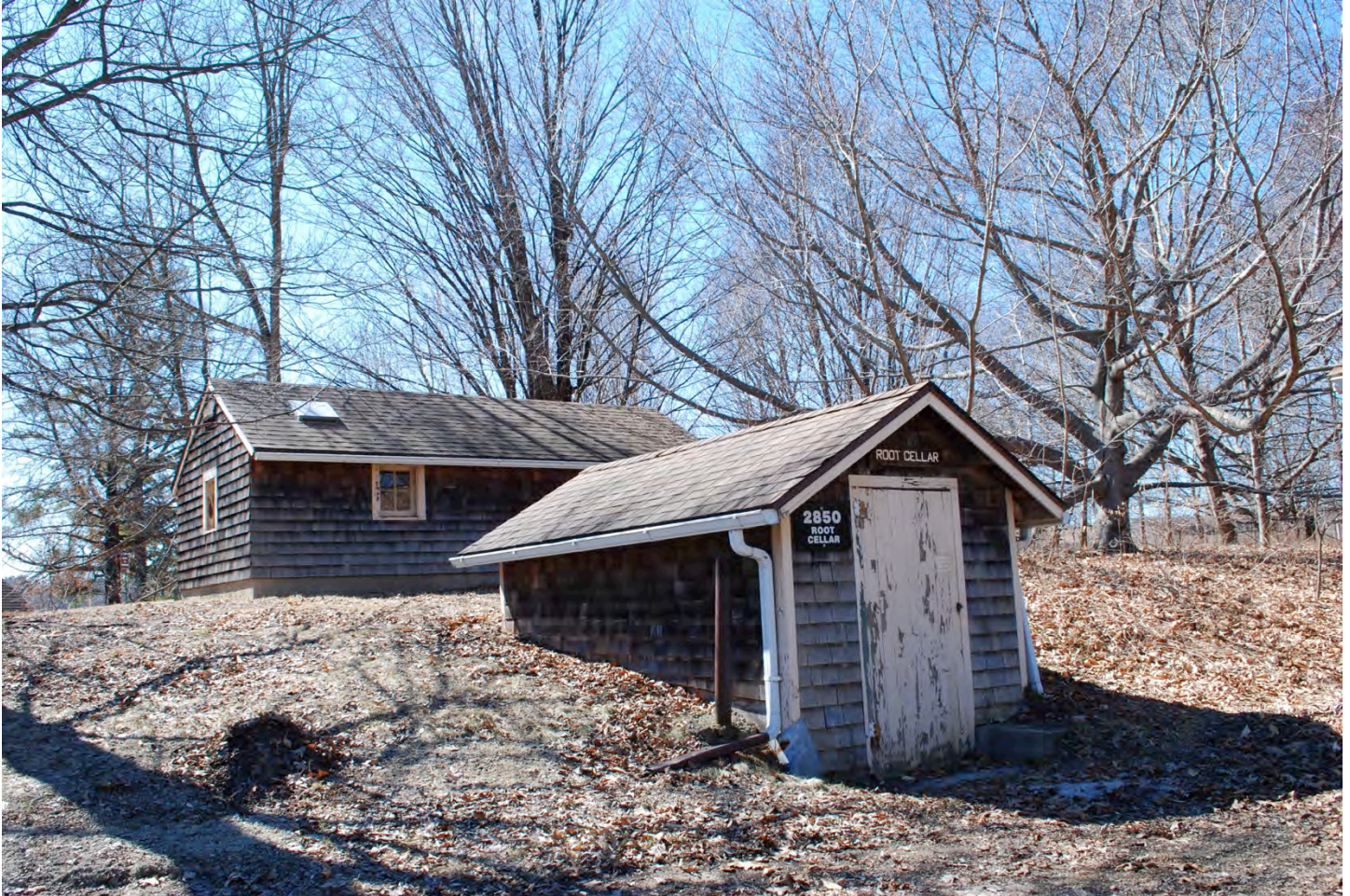
WI_DaneCounty_University of Wisconsin Arboretum_0014 Root Cellar and Main Pumphouse, camera facing westerly.
