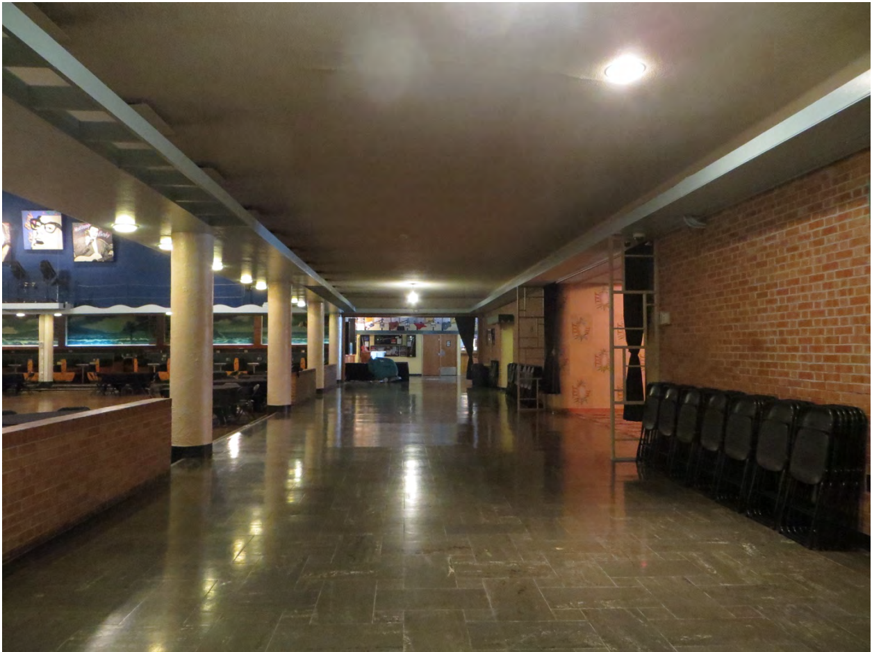
Photograph 20: Interior - Ballroom promenade, looking east with lobby opening at right and dance floor at left. The ballroom promenade remains unaltered from the original and through the period of significance, with plan and finishes retained. (McDowell, 2018)
