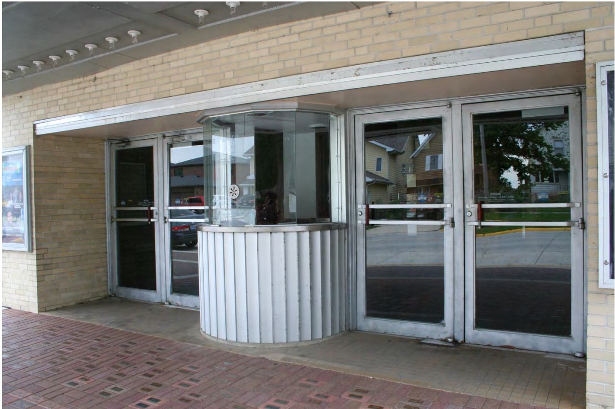
Photograph 8: Exterior Detail - Primary (south) entrance, ticket booth and doors. The ticket booth is accessed from the entrance vestibule and retains all original features. The doors retain Bakelite handles. The red pavers are non-historic alterations, but the buff-colored tile abutting the entrance doors is original. (McDowell, 2018)
