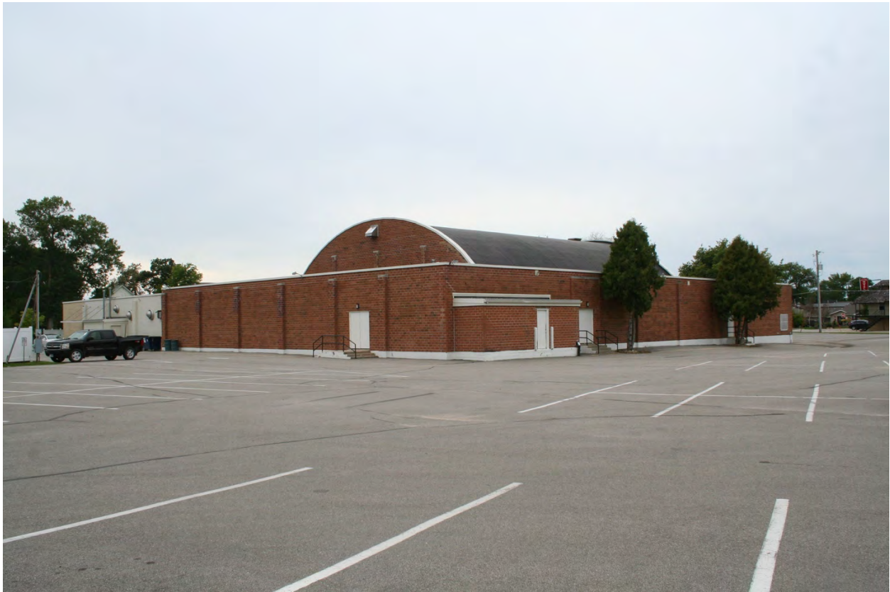
Photograph 6: Exterior - View of the north and west elevations, looking south. The barrel roof over the ballroom dominates the building from the rear perspectives. (McDowell, 2018)
