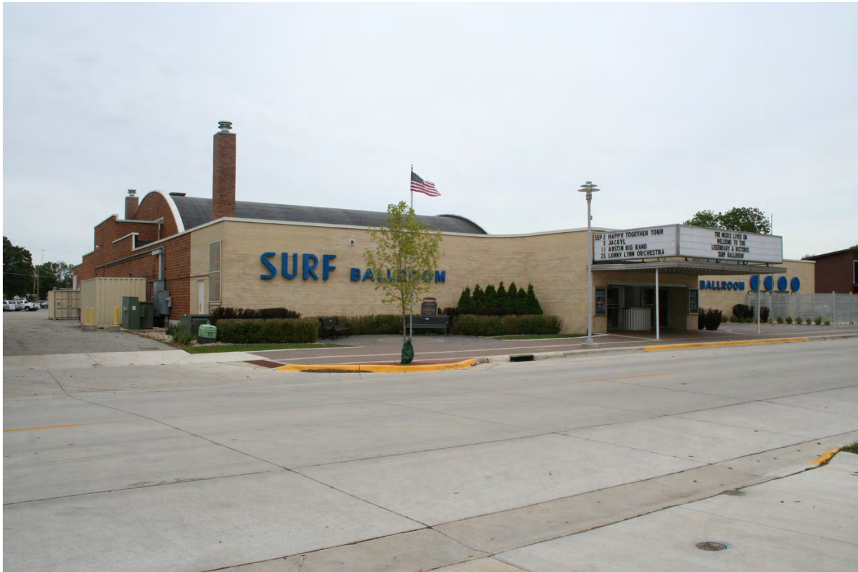
Photograph 5: Exterior - View of the façade (south) and west elevations, looking northeast. From this perspective, the juxtaposition of roof forms is well understood. The view also shows the 1994-era landscaping and the 2012 bronze marker commemorating the property's listing on the National Register of Historic Places. (McDowell, 2018)
