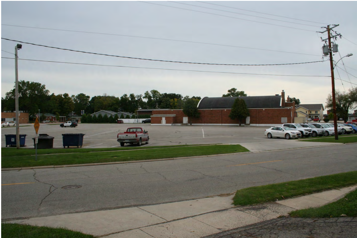
Photograph 3: Site View - Looking south. In this view, the barrel roof over the ballroom is in full view. A shallow section of roof at the west (right) end of the barrel roof marks the stage fly space. The property has included a large parking area from 1948, though the surfacing has been replaced multiple times. (McDowell, 2018)
