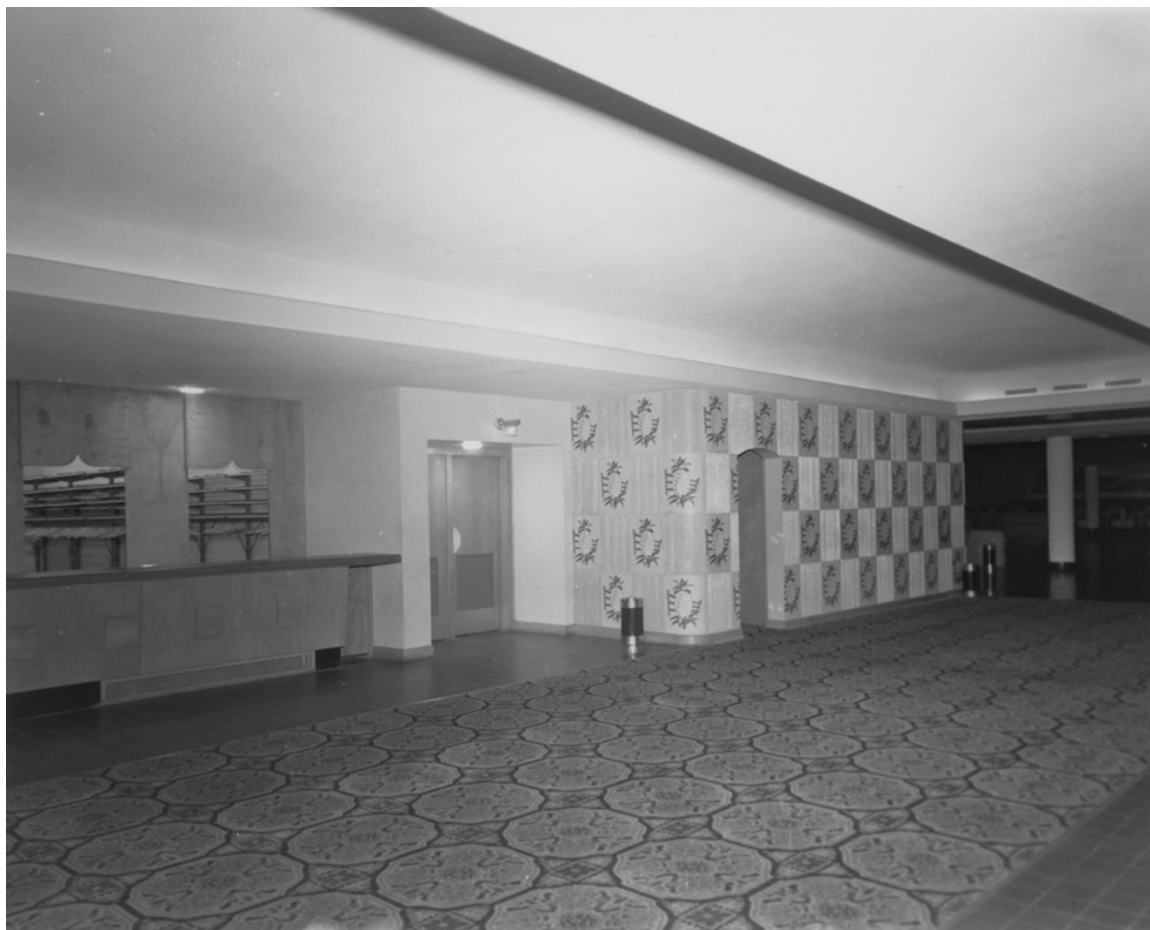
Historic Image 7: Interior – Lobby, looking northwest – 1949. Source: Surf Ballroom and Museum.
