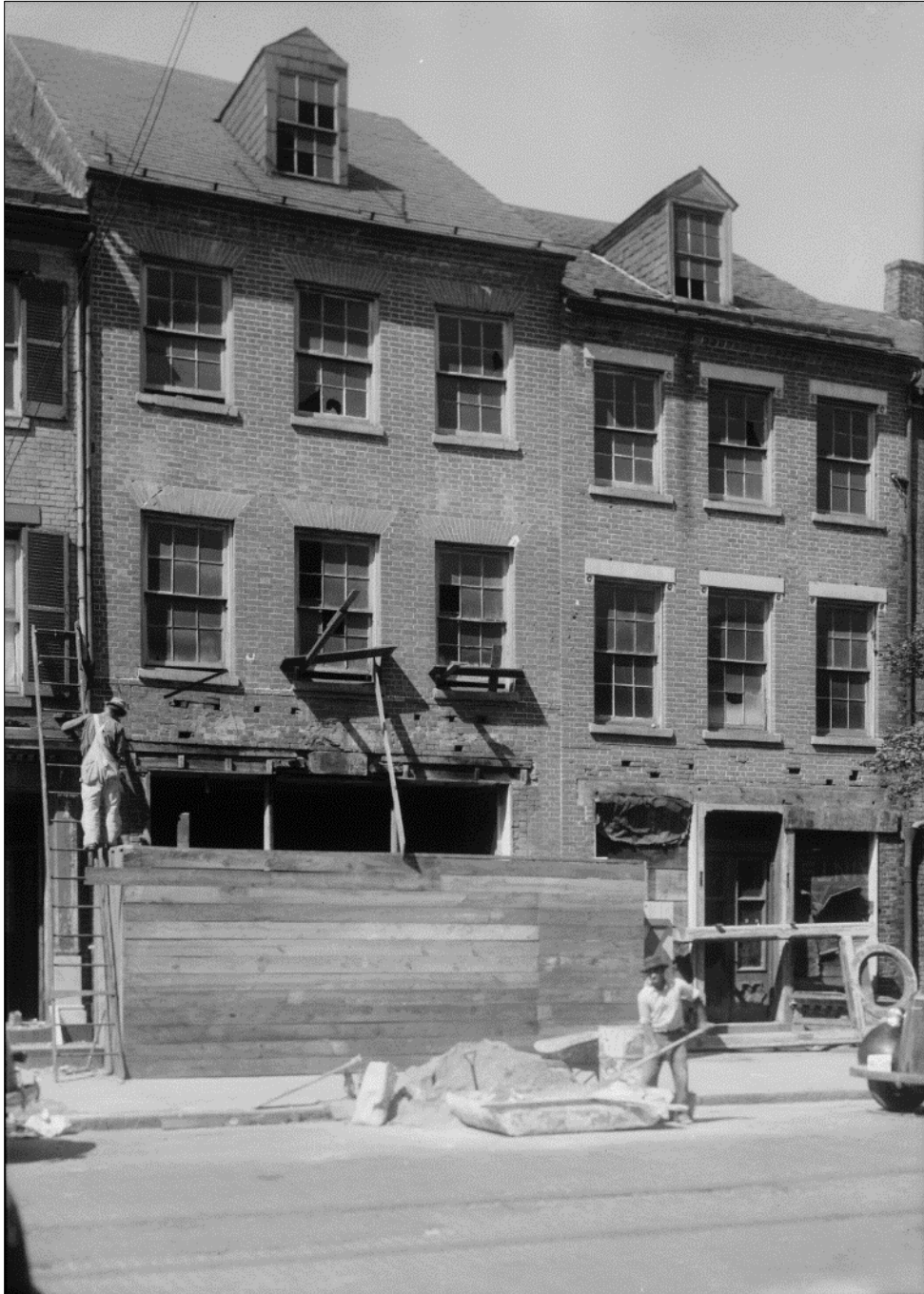
Figure 4. STABLER-LEADBEATER APOTHECARY SHOP, Alexandria, Virginia During reconstruction of storefronts, ca. 1936.
