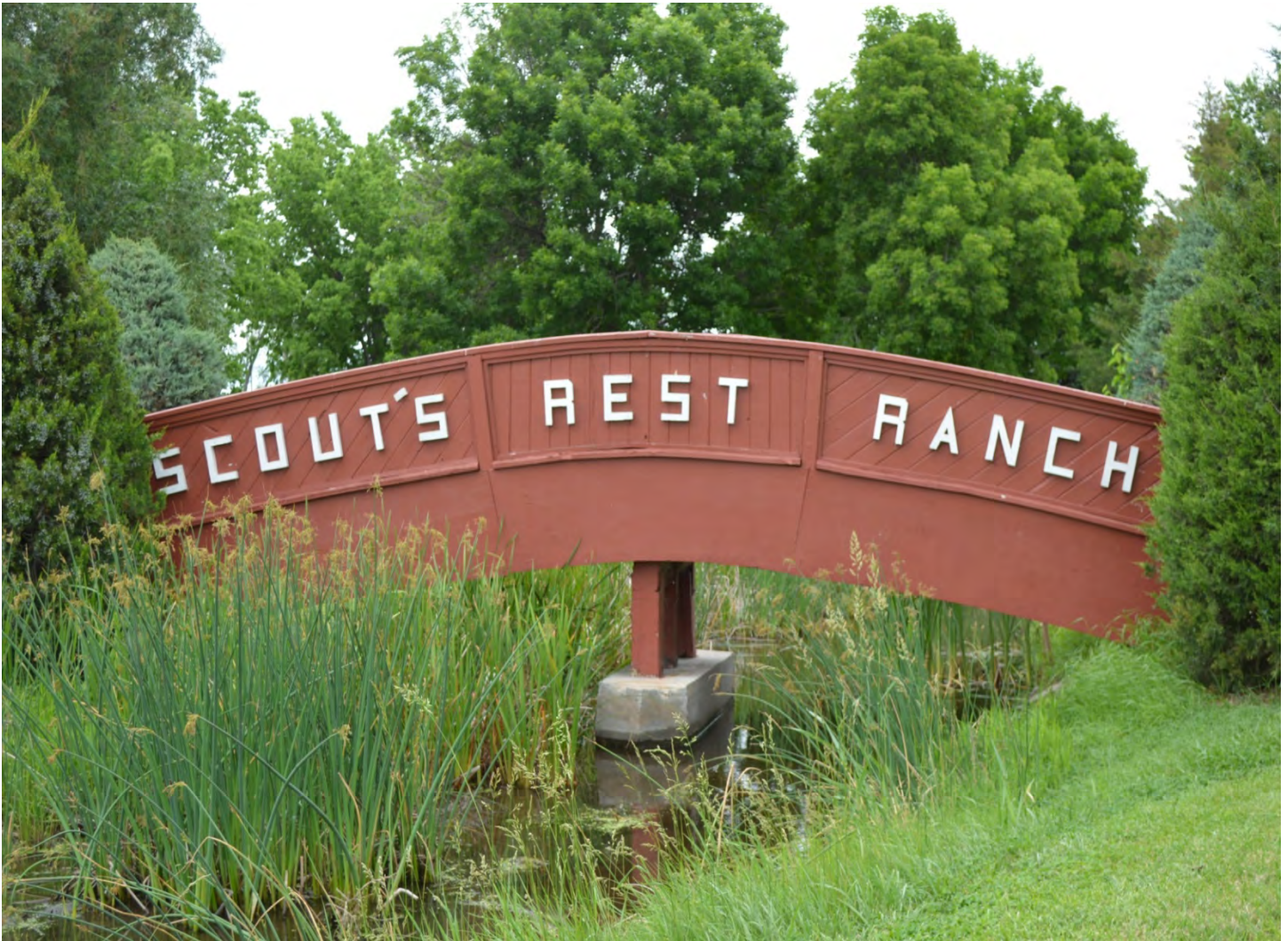
SCOUT'S REST RANCH HEADQUARTERS, North Platte, Nebraska Wooden Arch Footbridge Photo by Hannah Braun, June 2015
