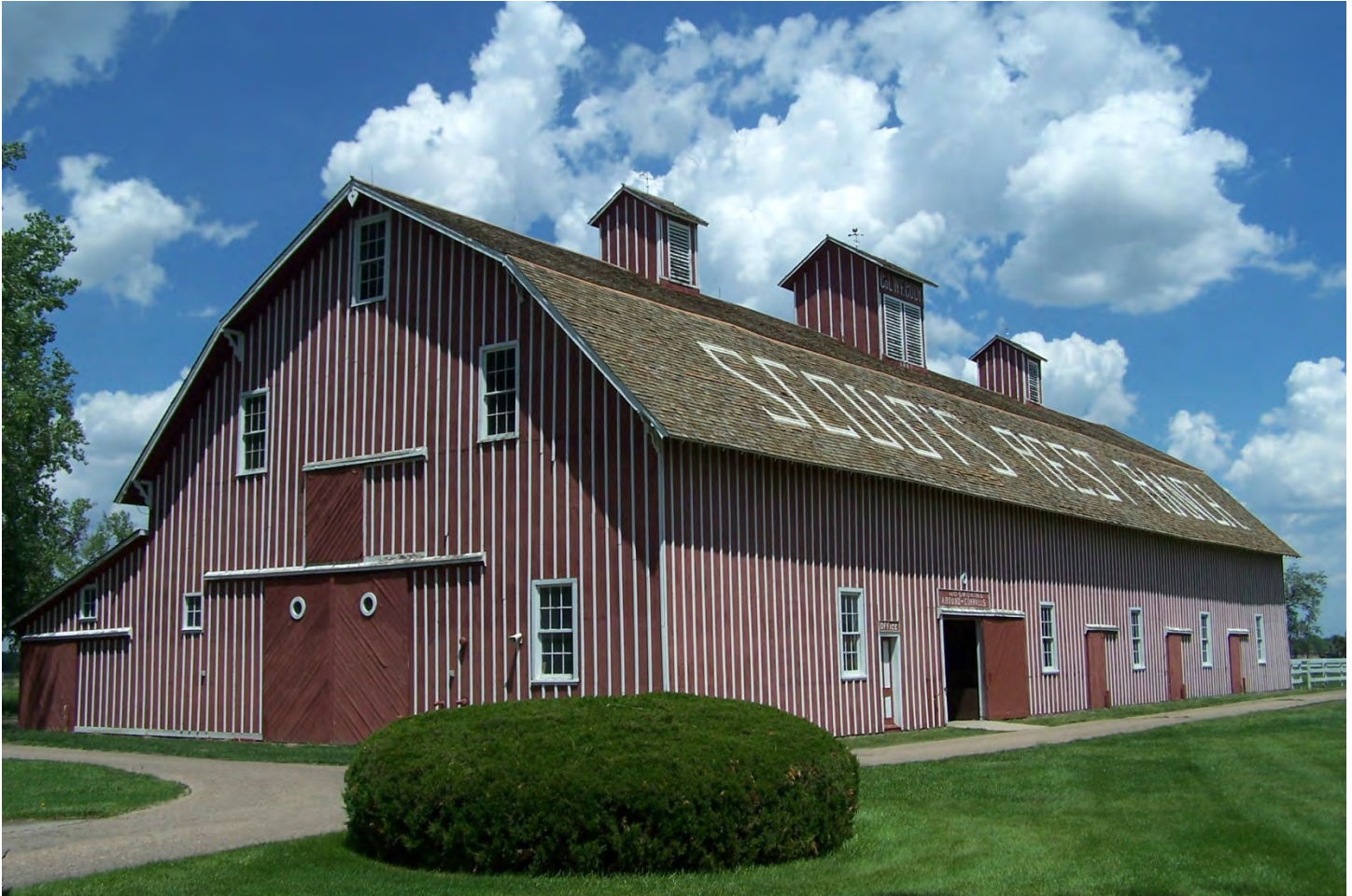
SCOUT'S REST RANCH HEADQUARTERS, North Platte, Nebraska Horse barn, west (main) façade and south elevation Photo by Hannah Braun, May 2014
