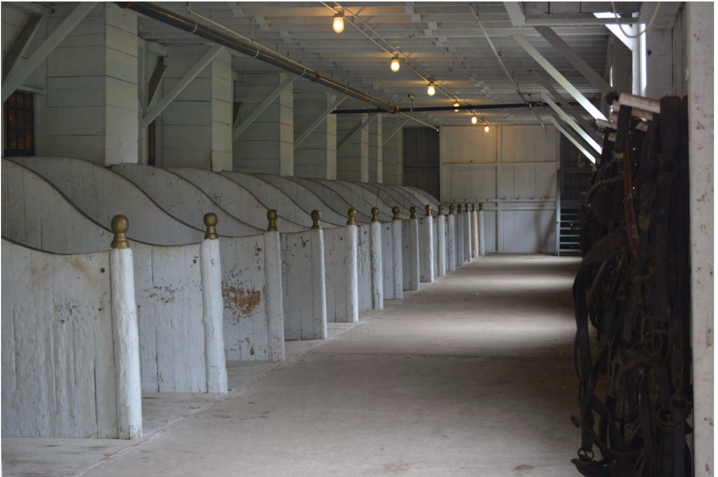
SCOUT'S REST RANCH HEADQUARTERS, North Platte, Nebraska Horse Barn first floor interior, horse stalls Photo by Hannah Braun, June 2015
