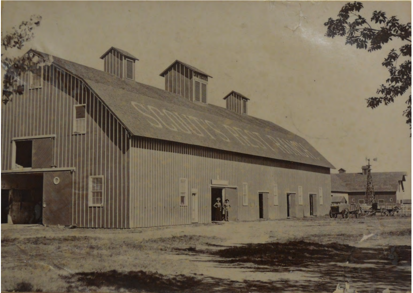
Figure 3: SCOUT'S REST RANCH HEADQUARTERS, North Platte, Nebraska West and south elevations of the horse barn with T barn and windmill beyond, ca. 1891–1904. Courtesy of Buffalo Bill State Historical Park, Archive room safe, Album 6 "Scout's Rest Ranch, Restoration, Welcome Wigwam," SSR-100, BB-117-834.
