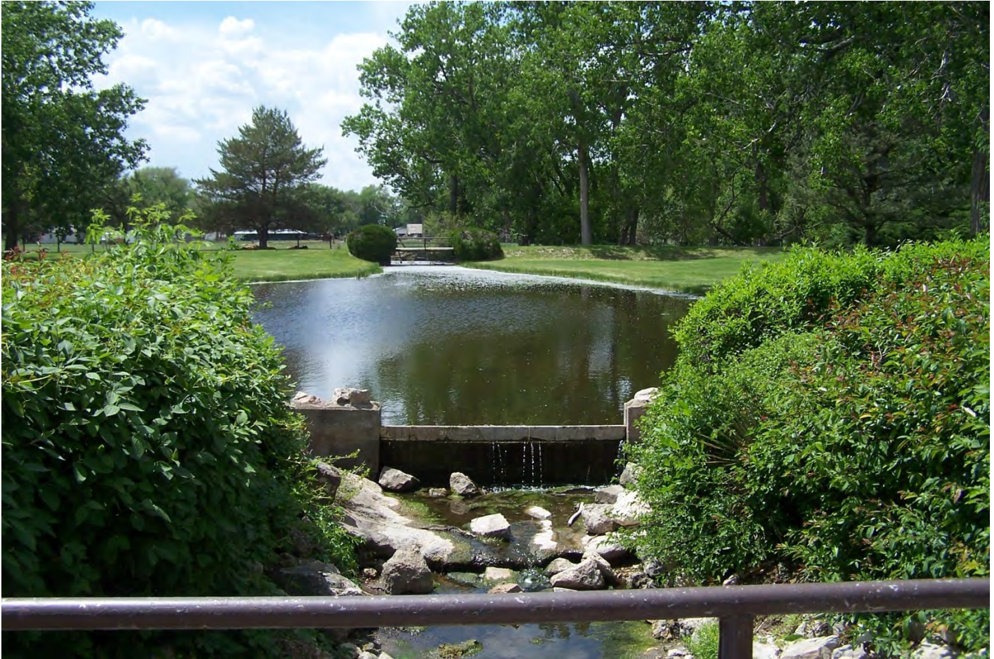
SCOUT'S REST RANCH HEADQUARTERS, North Platte, Nebraska Diversion Dam and Diversion Pond Photo by Hannah Braun, May 2014
