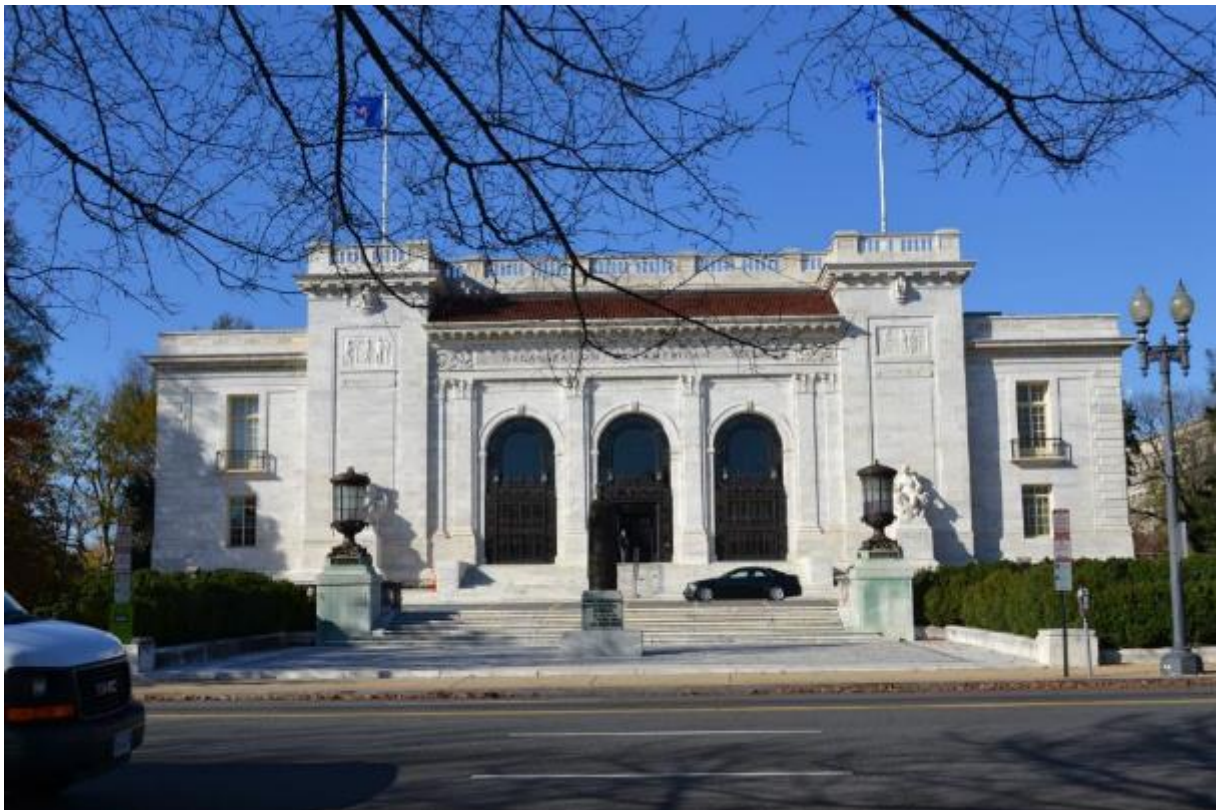
Photograph 3: View west to front façade facing 17th Street (S. C. Salvatore, 2015).
