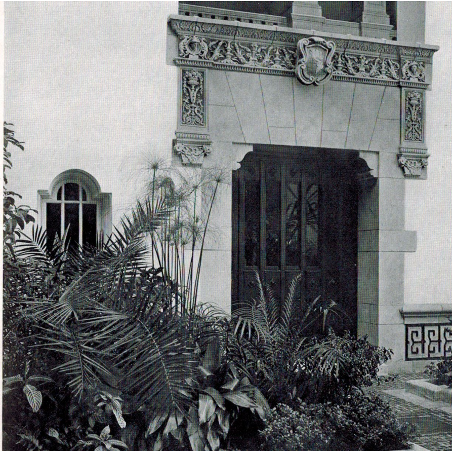
Historic Photo 7: View of one of the small doorways and window in the patio showing the original light configuration. Source: Barrett, Pan American Union (1911), 110.
