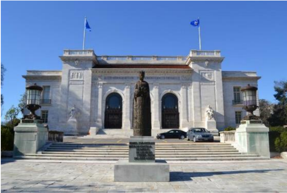
Photograph 6: View west to front façade with statute of Queen Isabella (1966), (S. C. Salvatore, 2015).
