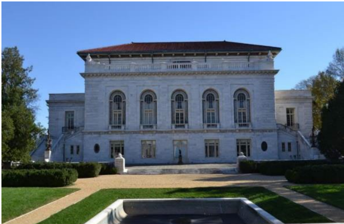
Photograph 5: View west to front façade facing 17th Street (S. C. Salvatore, 2015).
