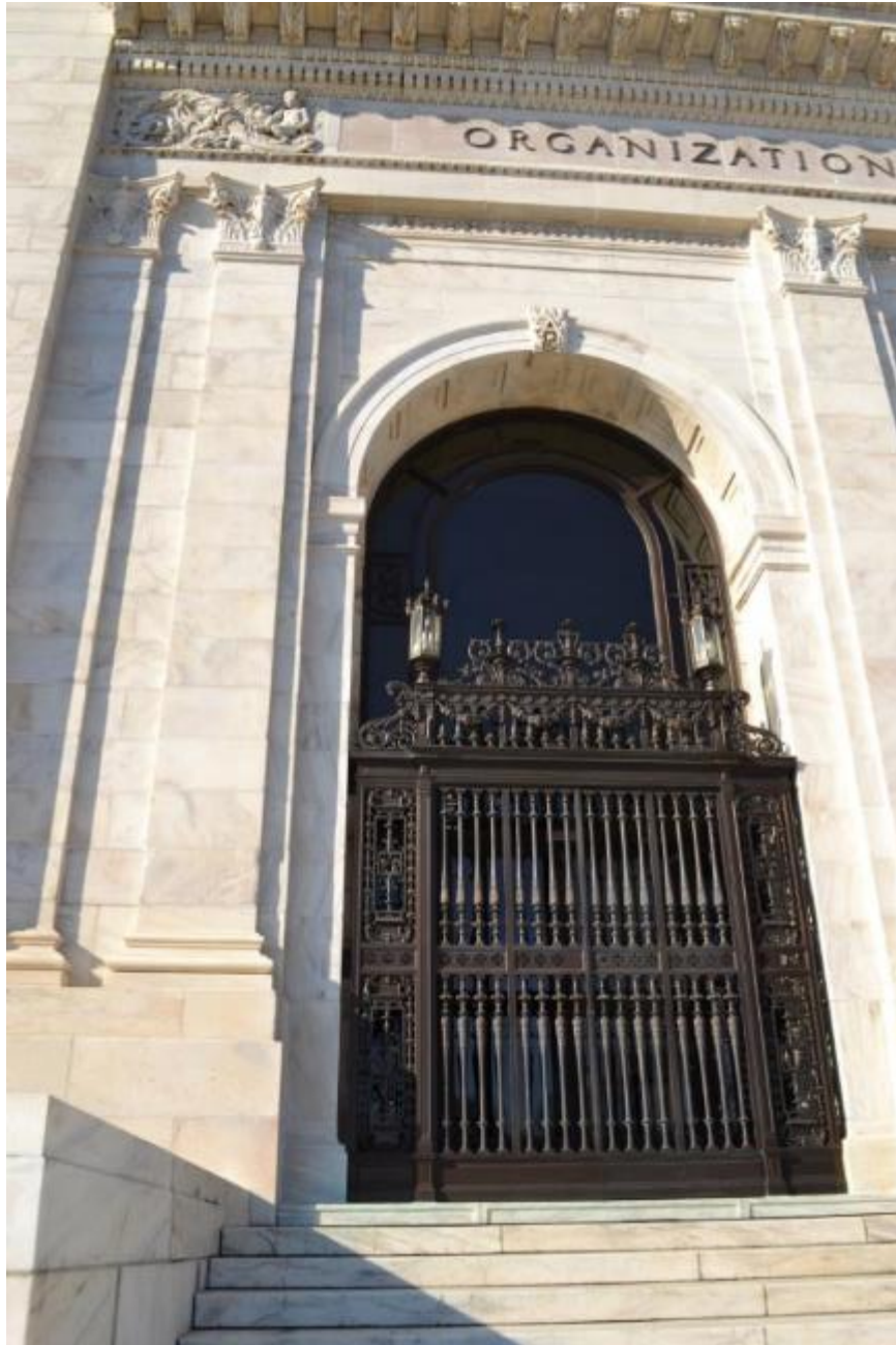
Photograph 5: Detail of southernmost gated entry. (S. C. Salvatore, 2015).
