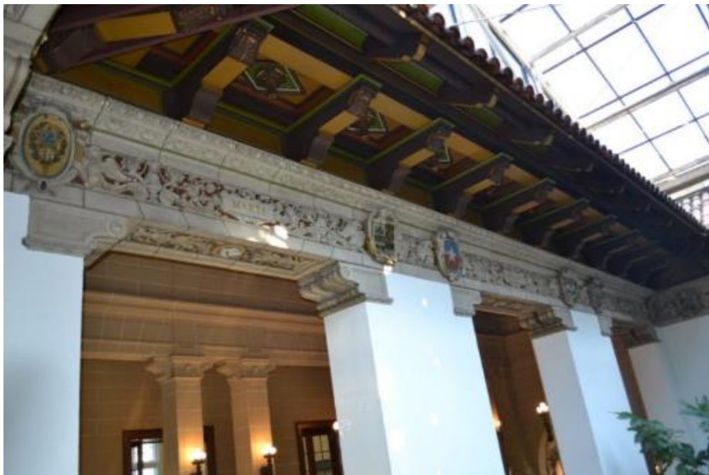
Photograph 8: View from second floor to close-up of patio frieze with coats of arms of founding countries interspersed with names of important people. Above are the overhanging decorative roof eave and the glass roof (S. C. Salvatore, 2015).
