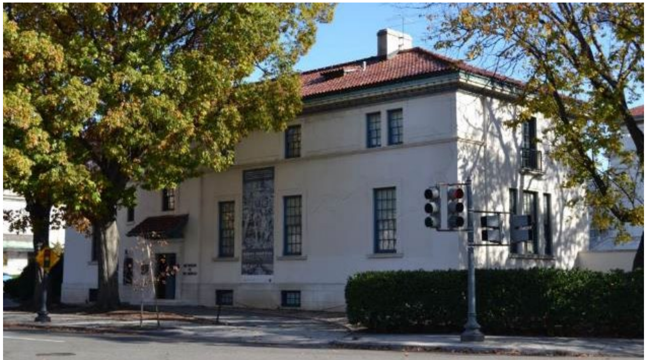
Photograph 16: View looking northeast at the annex west (front) and south sides (S. C. Salvatore, 2015).
