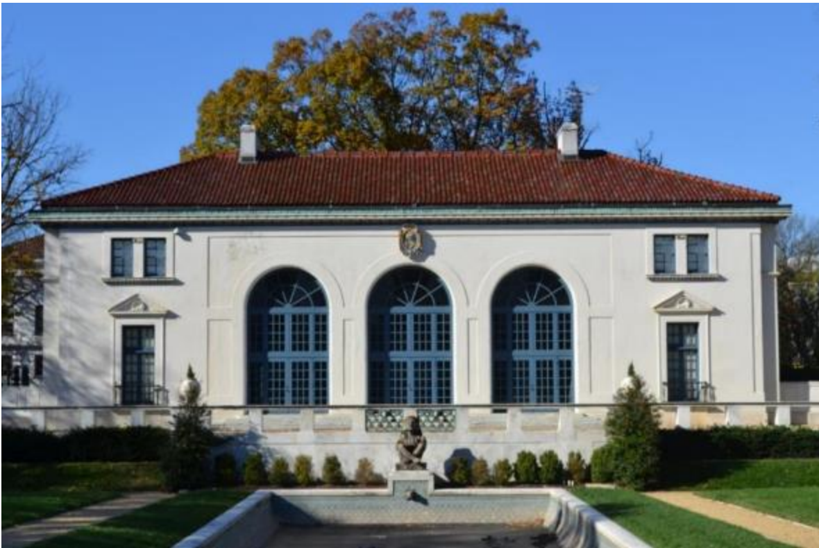
Photograph 15: View looking west showing Aztec god sculpture at pool, rear (east elevation) of the annex where arched openings lead into the loggia (S. C. Salvatore, 2015).
