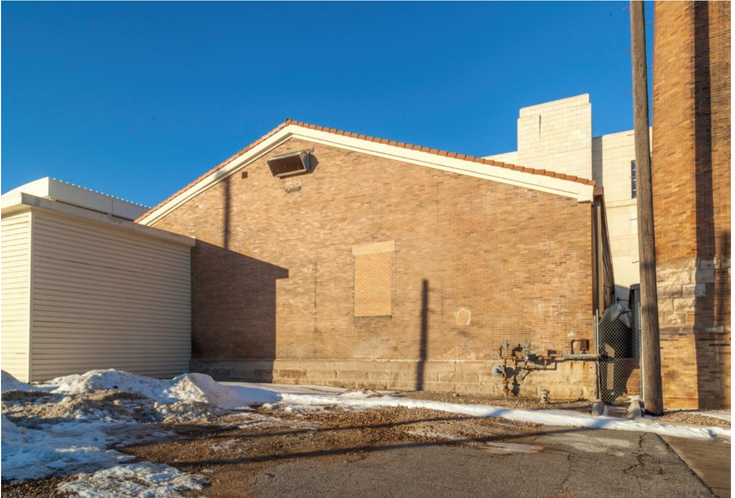
OMAHA UNION STATION, 1899, BOILER HOUSE, EAST WALL
