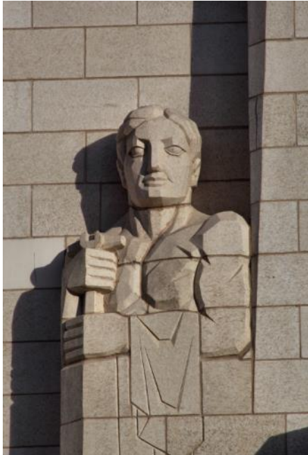
OMAHA UNION STATION, 1931, WEST ENTRANCE DETAIL: ARTICULATED TRACK WORKER HOLDING A SPIKE HAMMER
