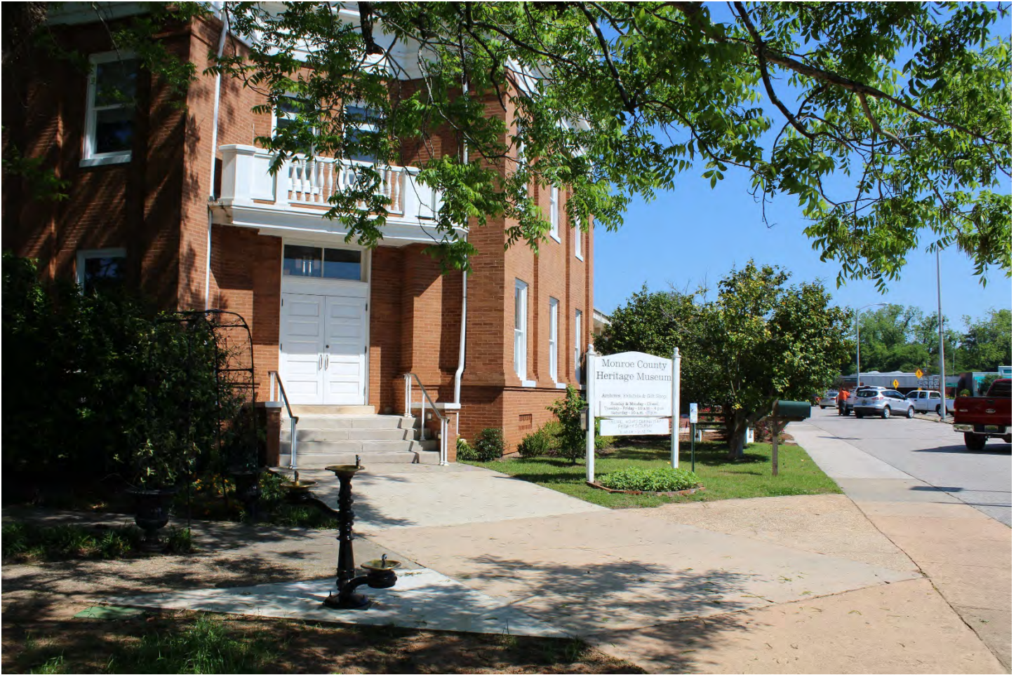
Photo 2 of 14 Southeast entrance to courthouse, looking north. May 2017.
