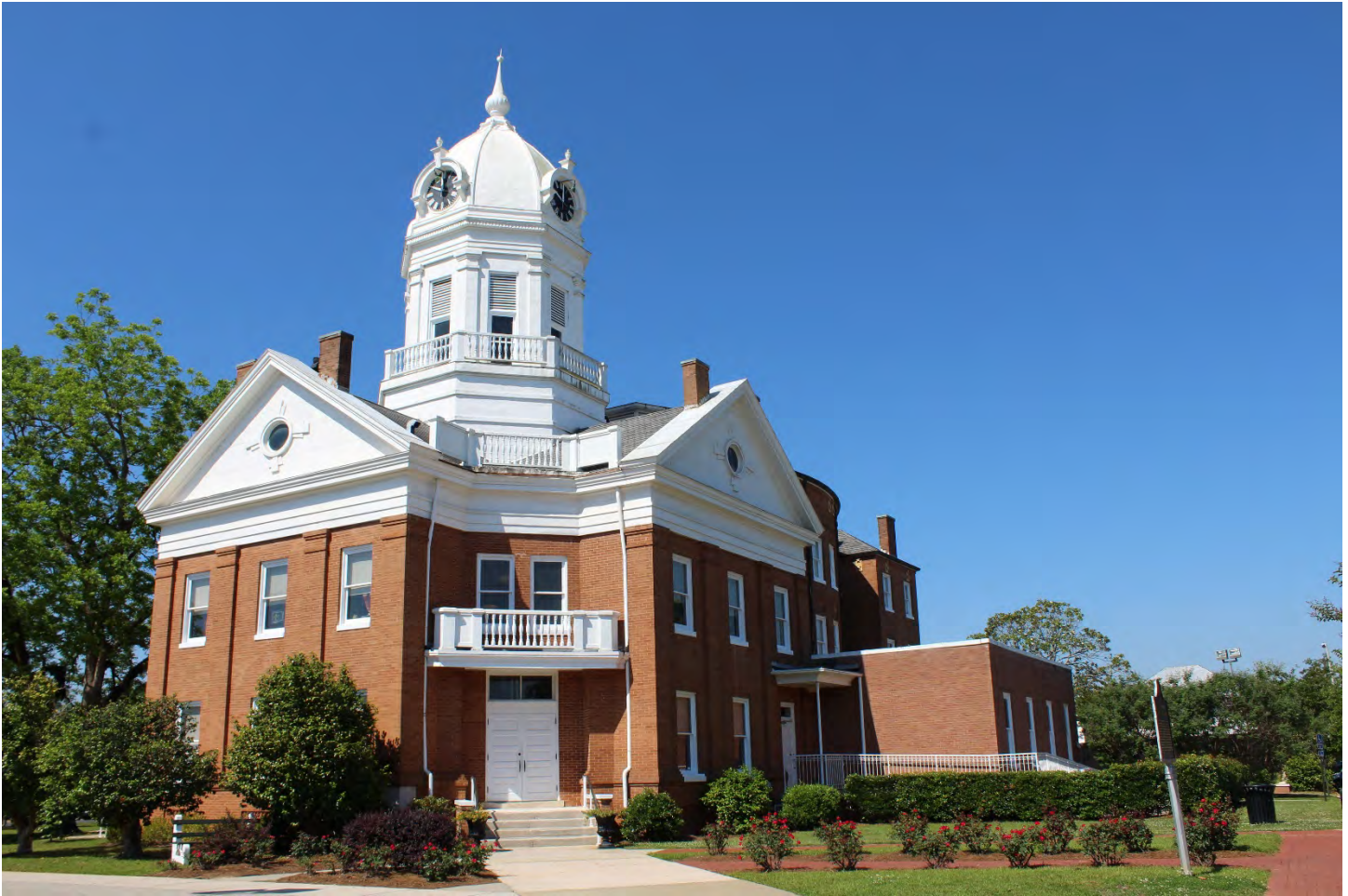
Photo 1 of 14 Courthouse, looking southwest. May 2017.
