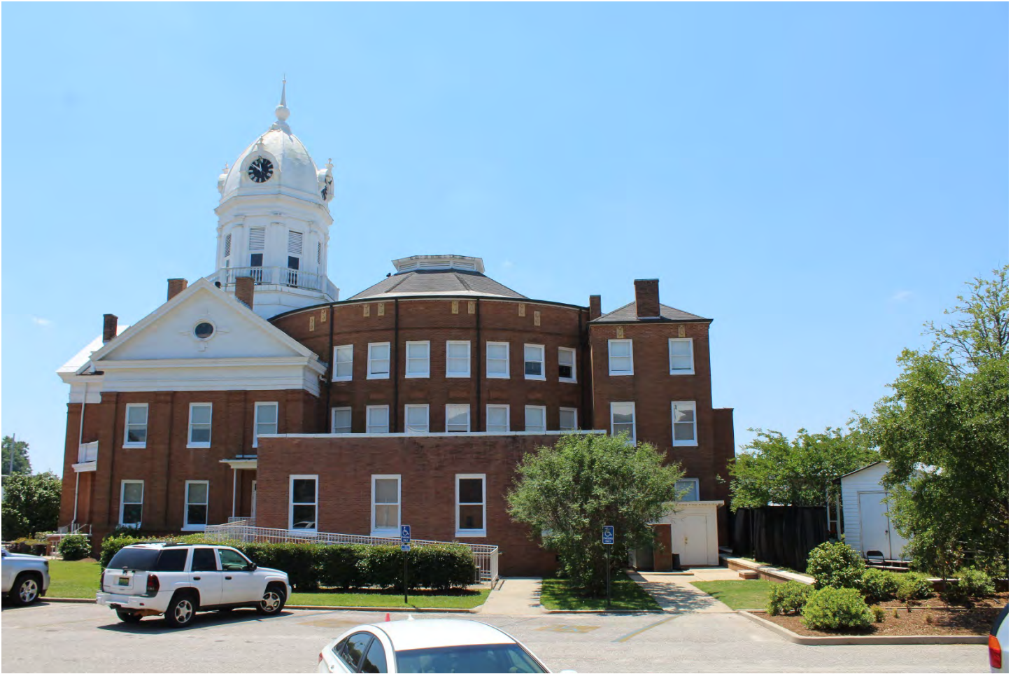
Photo 5 of 14 North (rear) elevation of courthouse, looking south from 1963 courthouse. May 2017.
