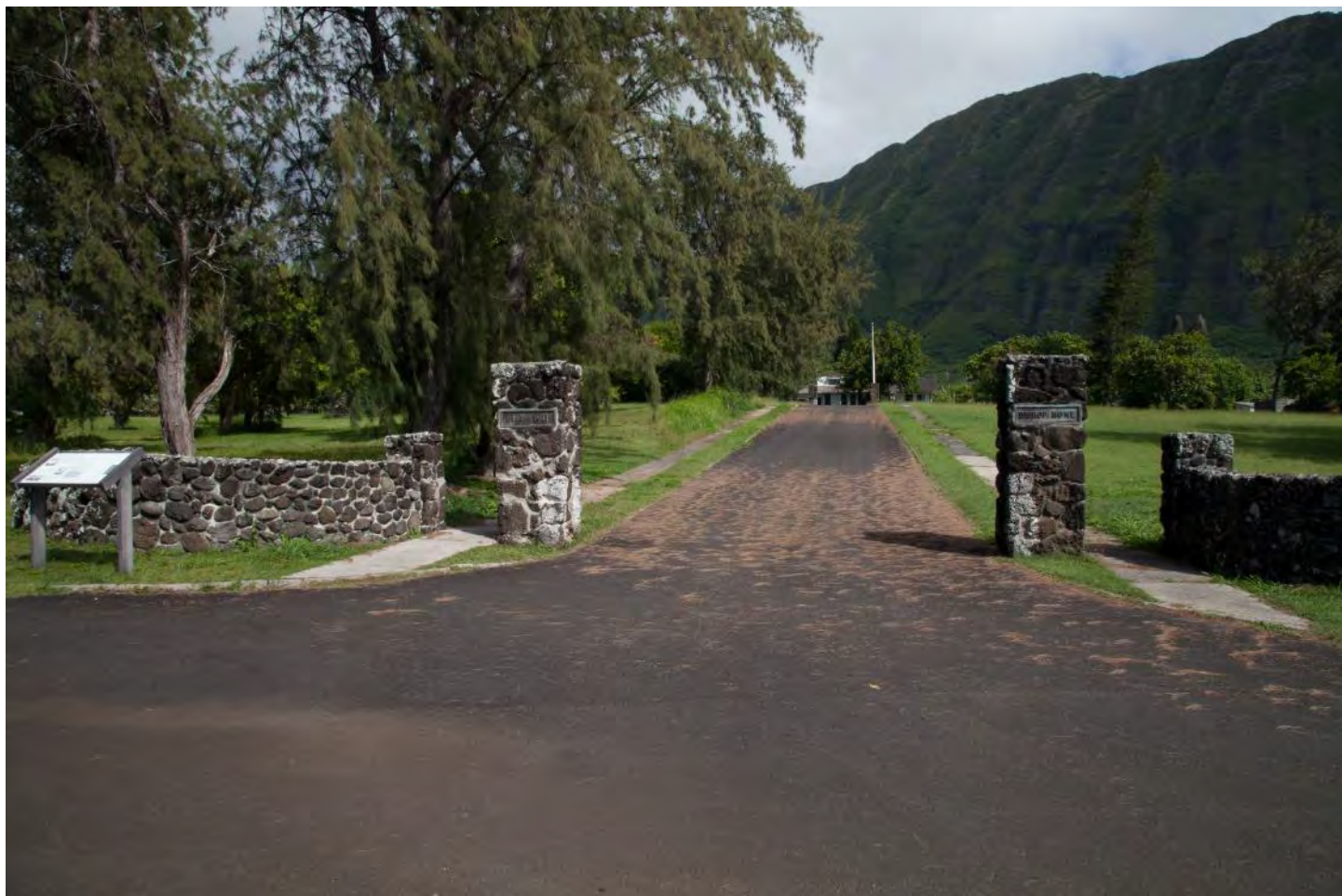
Photo 26: Stone and mortar pylons at the entrance driveway to the Bishop Home at the corner of School Street and Puahi Street, camera facing southeast. These are part of the Bishop Home Walls and Entrance Gates (830) Portions of the Bishop Home Roads and Curbs (832) and Bishop Home Sidewalks (861) are also visible.
