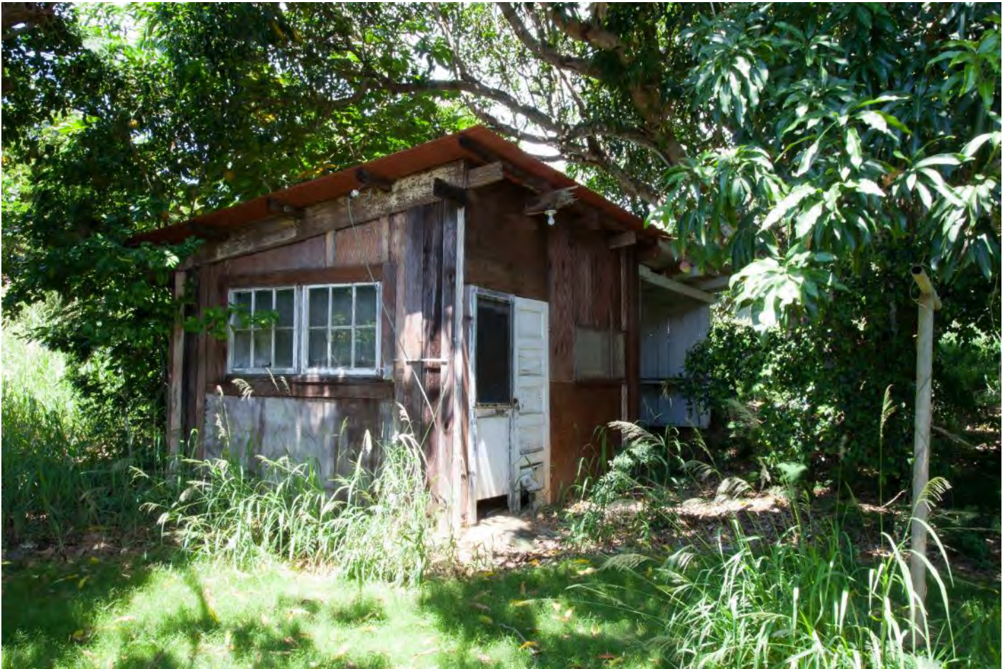
Photo 73: Puahi Street Storage Building 520 (520), camera facing northeast. This is an example of an outbuilding constructed of recycled materials.
