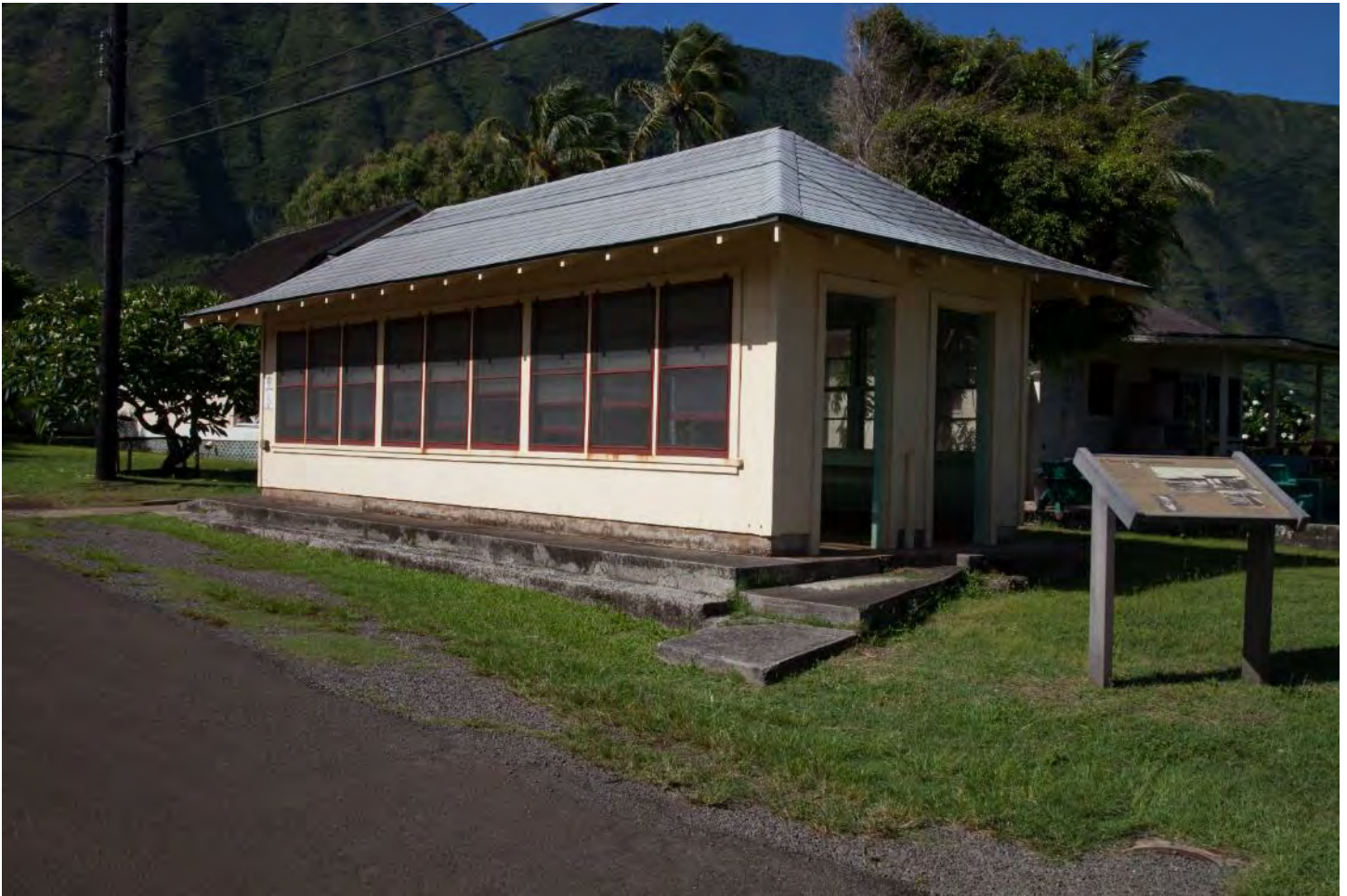
Photo 31: Visitors' Pavilion (278BV), camera facing southwest. This building was constructed in 1933 to provide a space for settlement residents to meet with visitors. Initially a wire screen ran down the length of the room to ensure separation. This was removed and replaced with a two-foot-wide table in the 1940s.
