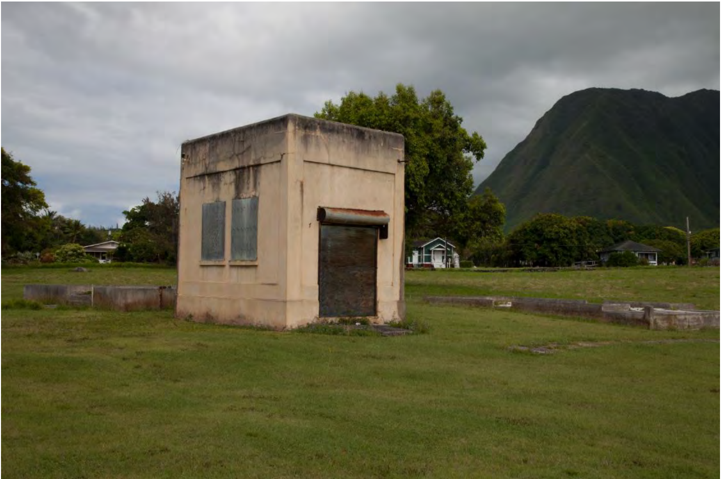
Photo 24: Bishop Home Boiler Plant (7aBH), camera facing east-southeast.
