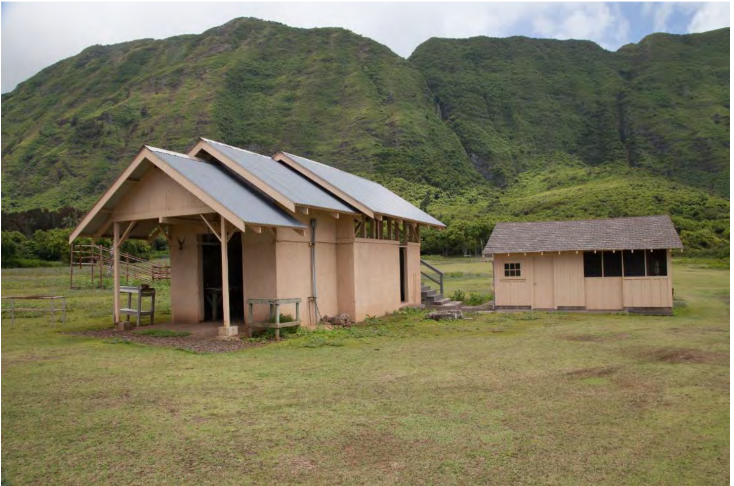
Photo 37: Slaughterhouse (630) in the left foreground and Slaughterhouse Restroom (258), camera facing southeast. The metal pipe rail loading ramp is partially visible behind and to the left of the slaughterhouse. The slaughterhouse equipment is still inside the building and is used by residents who hunt in the area.
