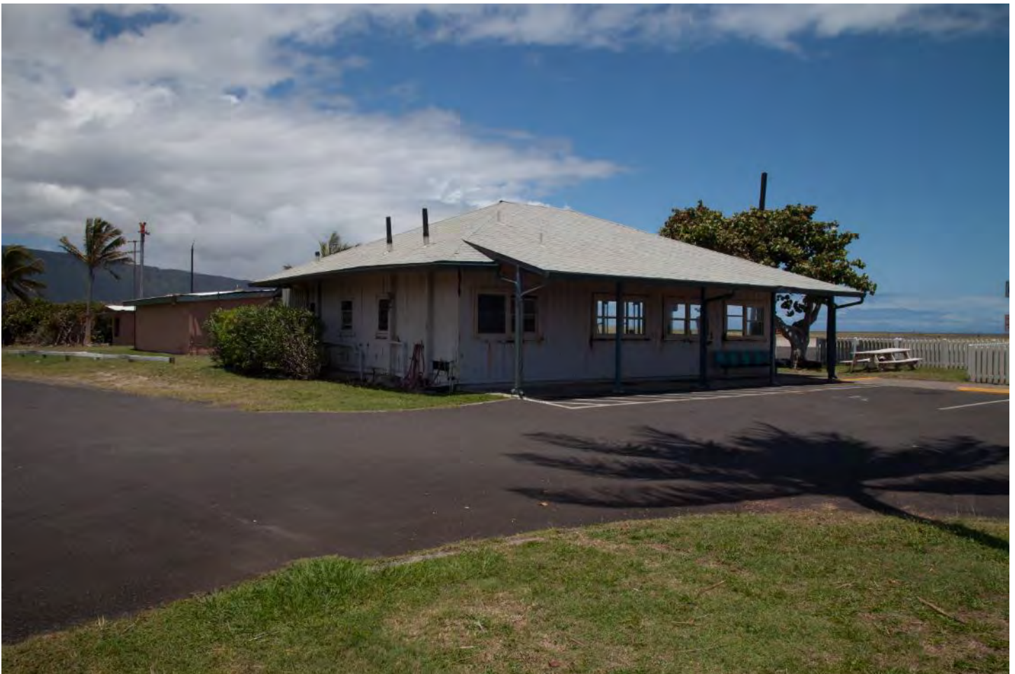
Photo 2: Airport Terminal (703), camera facing southwest.
