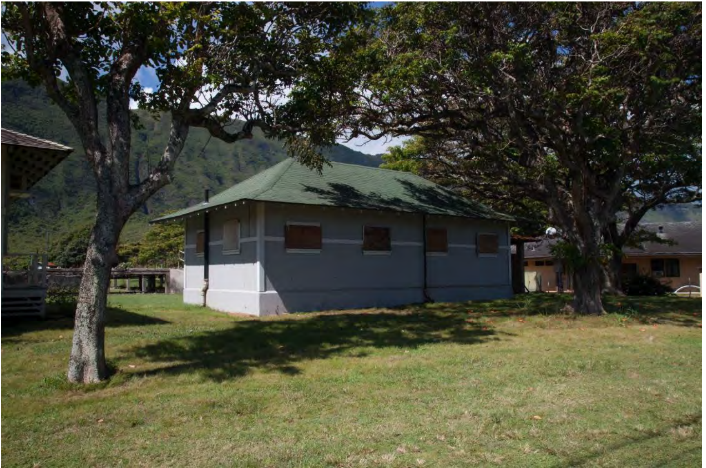
Photo 59: Fumigation Room (283BH), camera facing southwest. Connected to the historic hospital (now a ruin) by a walkway, this is where mail, clothing, and anyone leaving the settlement for a short period of time were fumigated. This unpopular practice was ended in the 1940s after the introduction of sulfone drugs. Later, the building was used for the custom manufacture and fitting of shoes. Shoemaking materials are still inside.
