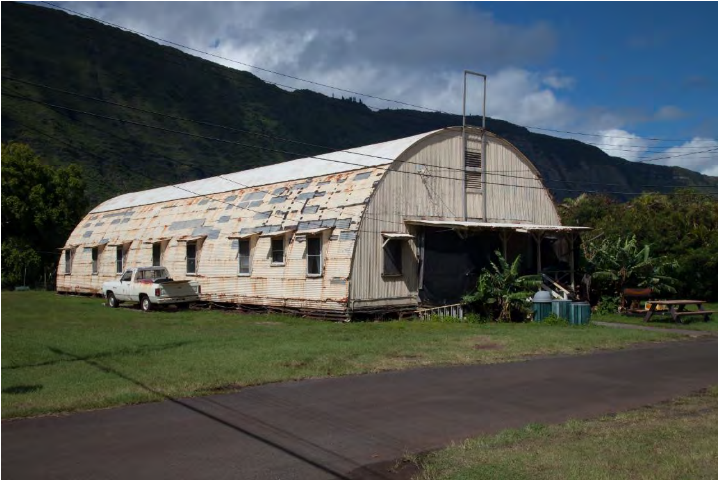
Photo 32: Quonset Dormitory (10BV), camera facing southwest.
