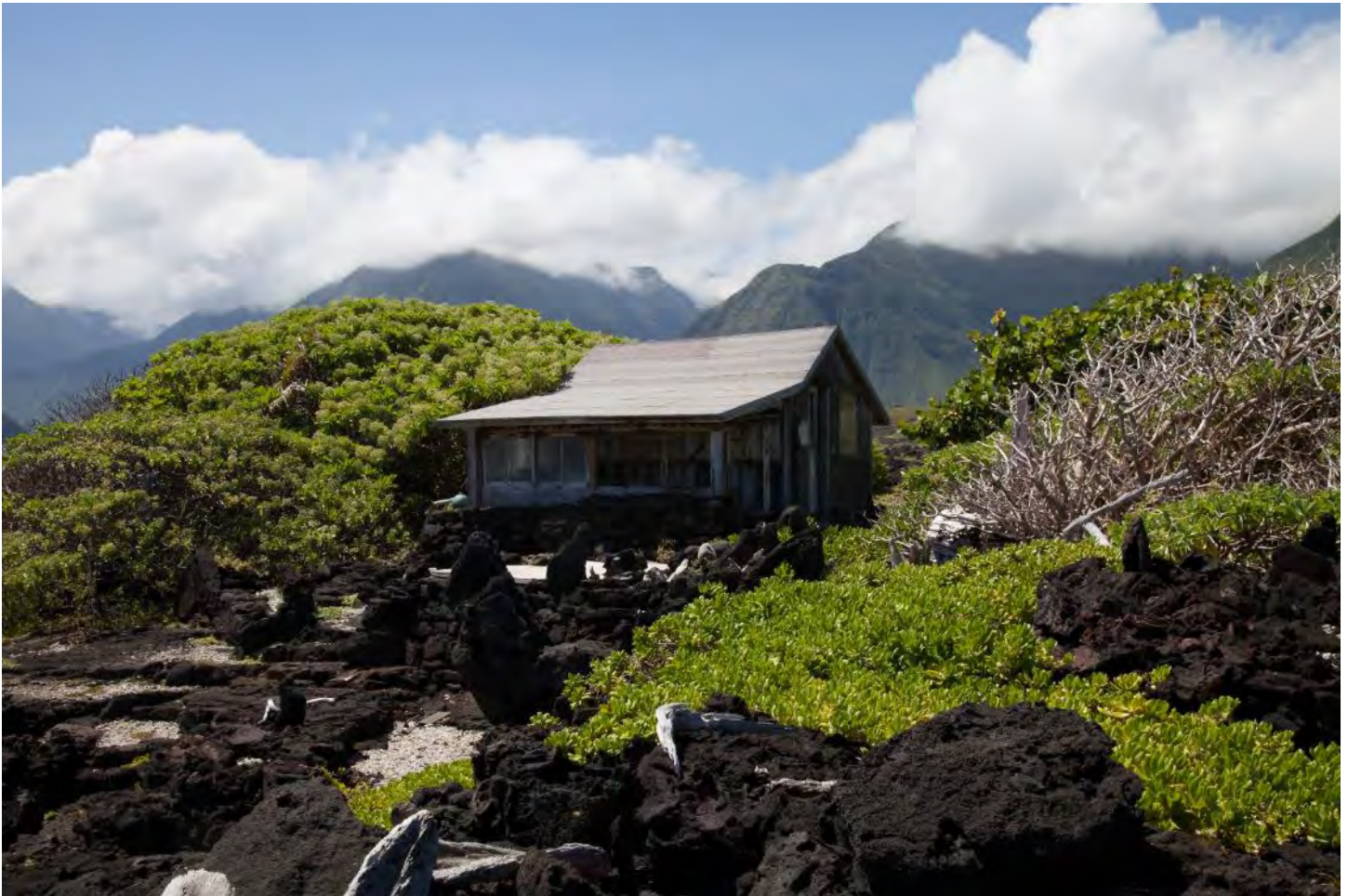
Photo 12: Richard Marks Beach House (856), camera facing southeast. The outdoor “hot tub” comprised of an old bathtub perched on stacked lava rocks is partially visible on the first terrace.
