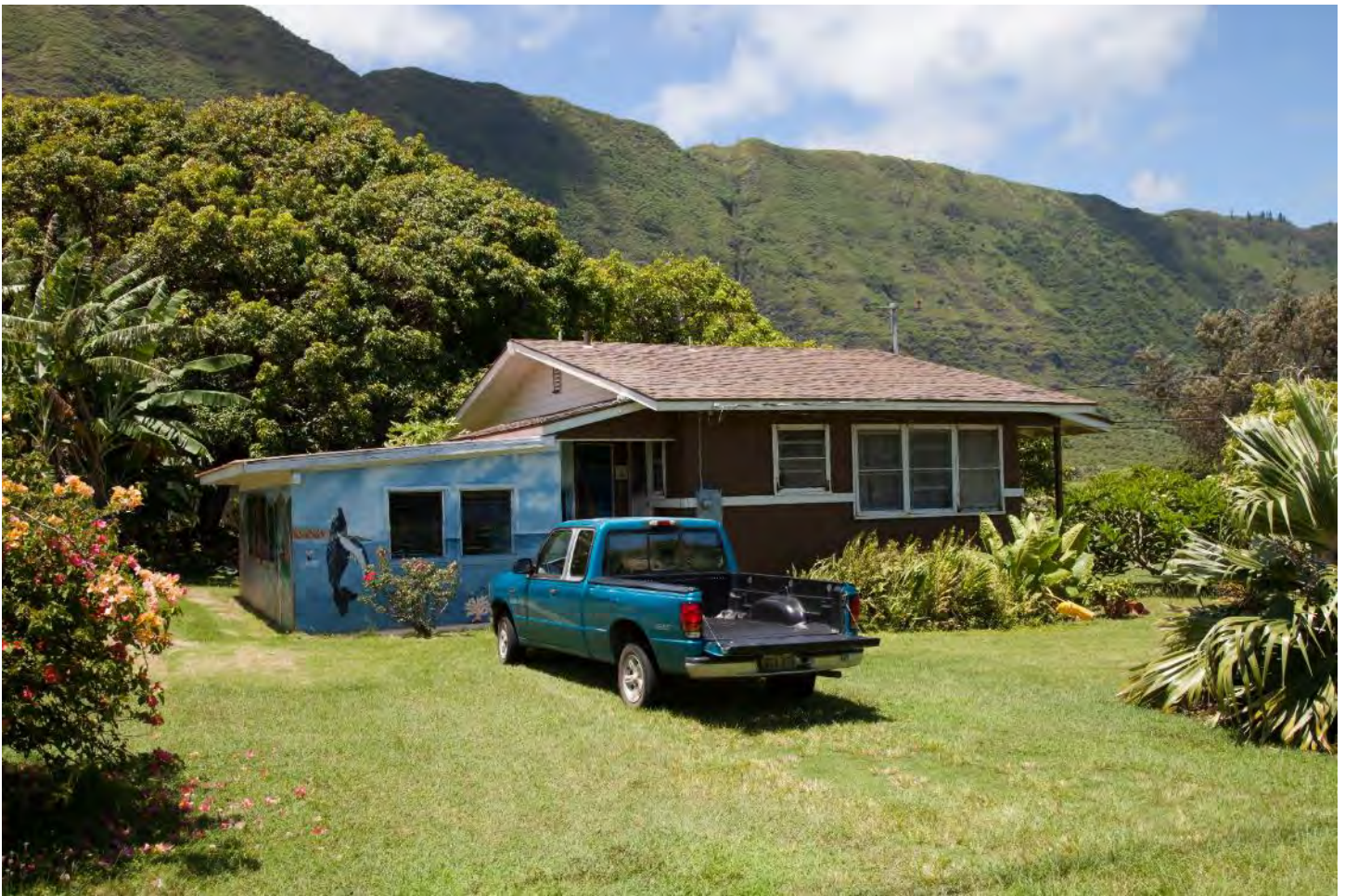
Photo 66: Lourdes Taghoy Residence (153-56), camera facing south.
