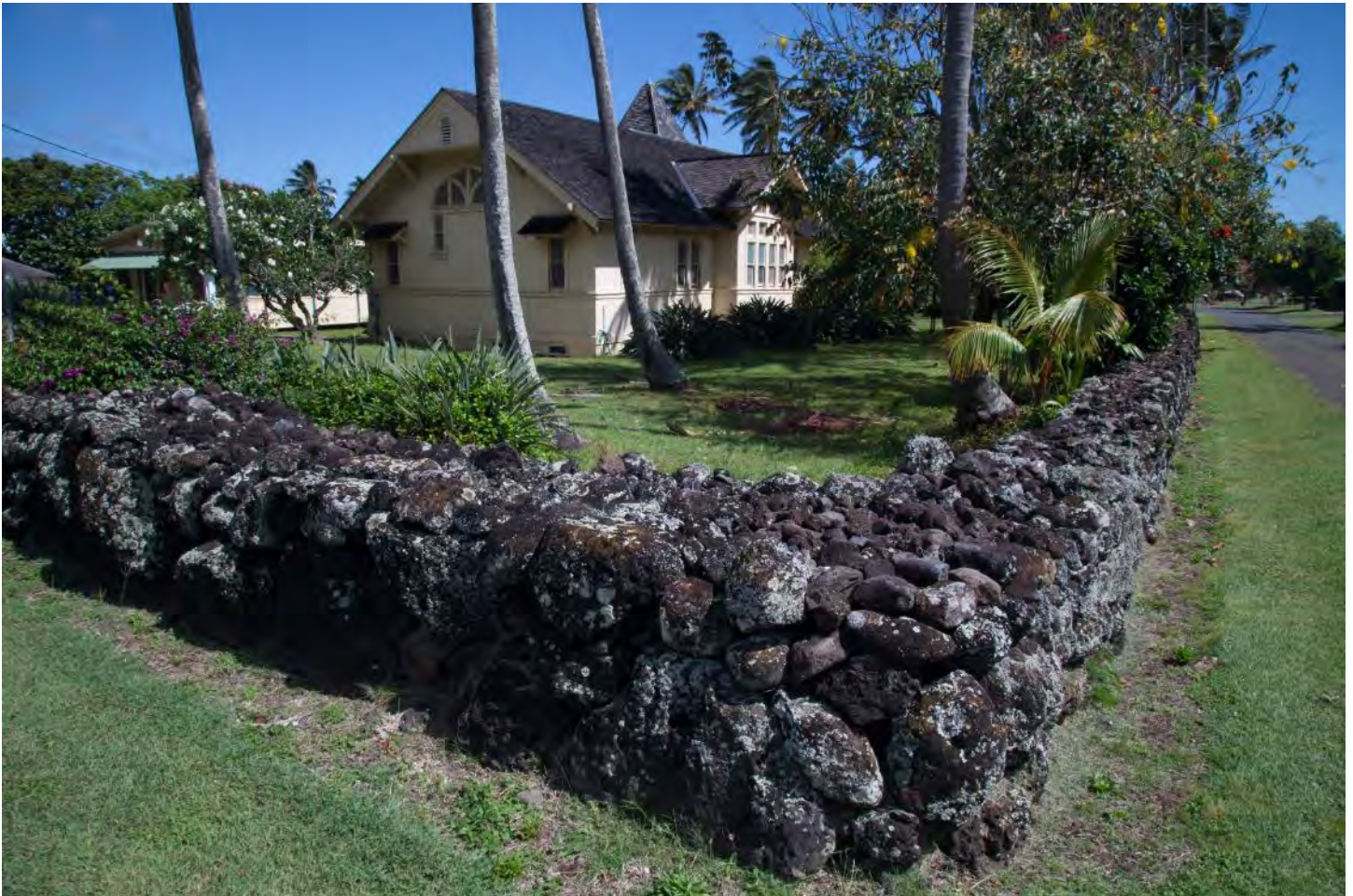
Photo 45: Kana'ana Hou Church (286) with a portion of the churchyard wall (841) in the foreground, camera facing northwest.
