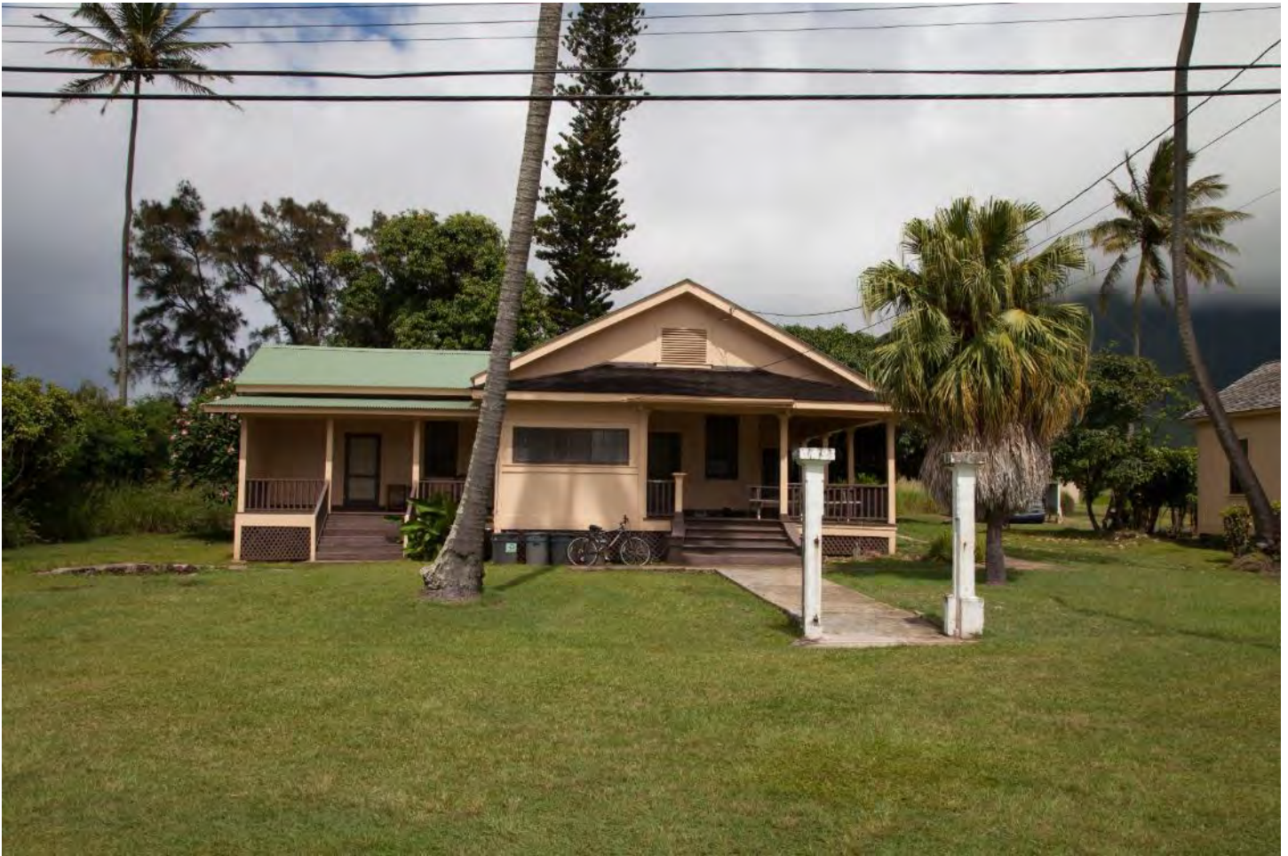
Photo 42: Resident Physician's Residence (10SR), camera facing east. The concrete gate posts at the entry walkway likely date to the early 1930s and are part of the contributing Staff Row Picket Fence Footing and Gate Posts (870).
