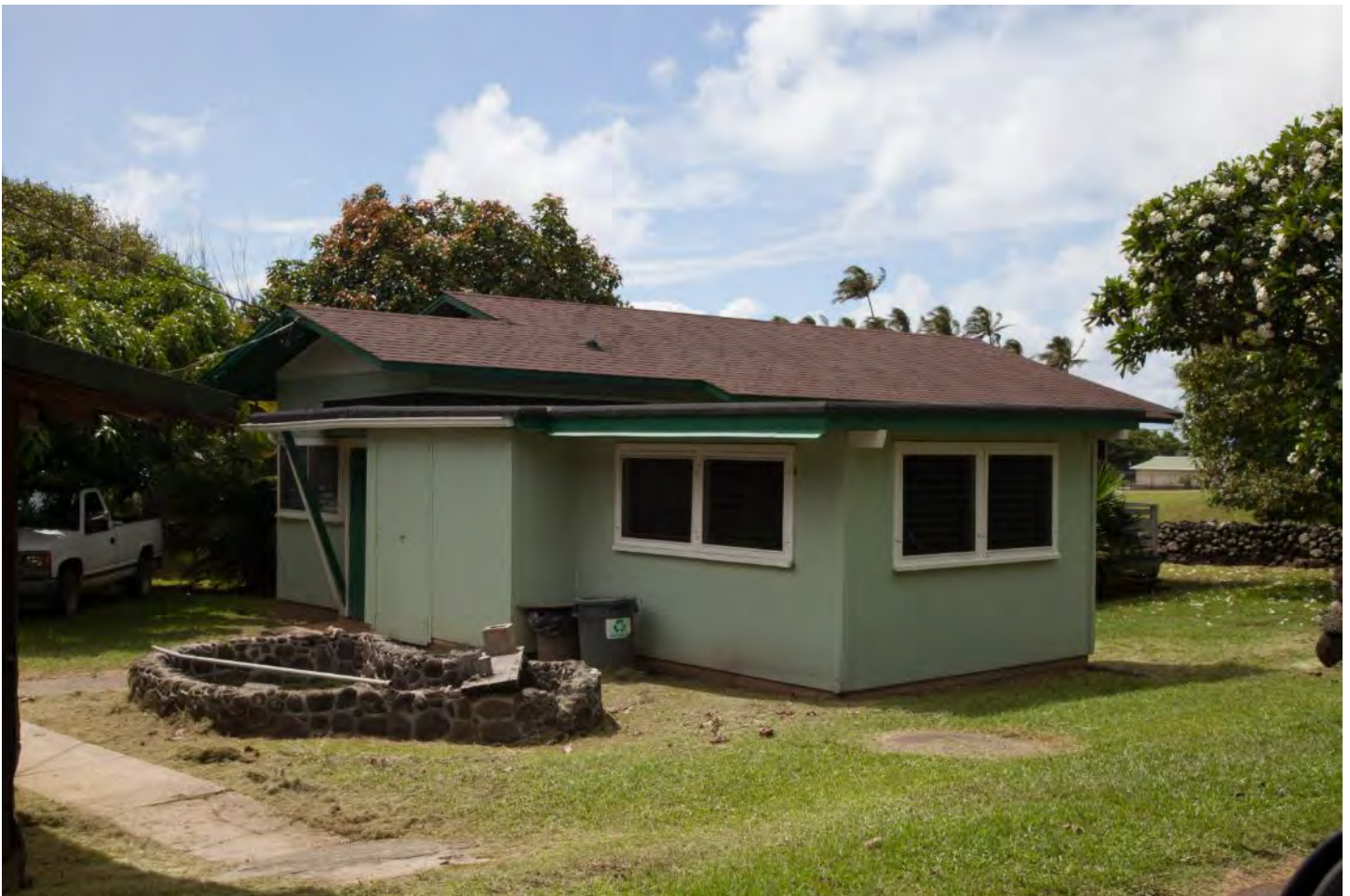
Photo 64: John Arruda Residence (121-64), camera facing northwest. A mortared rock fish pond is in the front yard.
