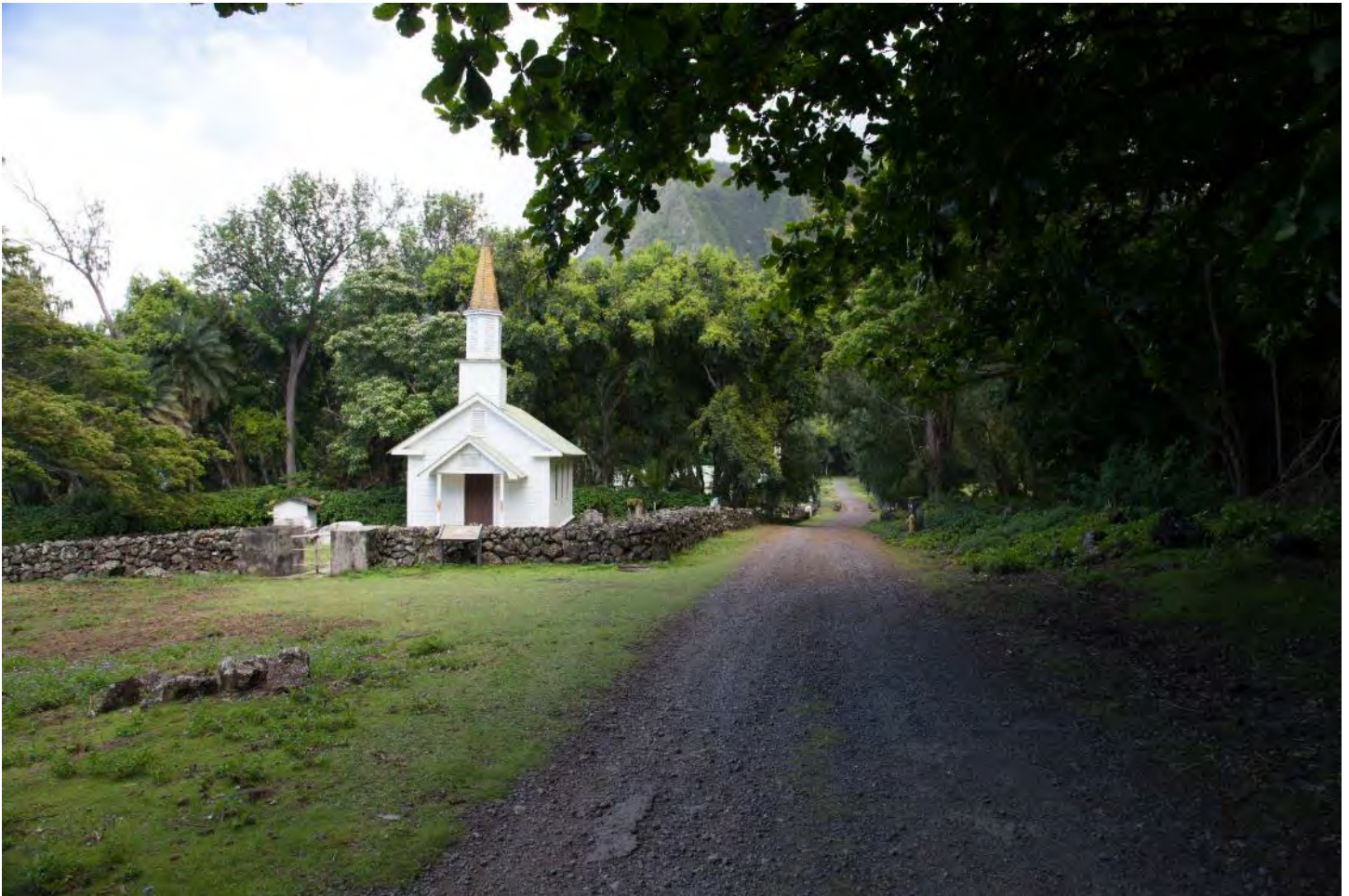
Photo 6: Damien Road in Kalawao, camera facing southeast. Siloama Church (710) is visible.
