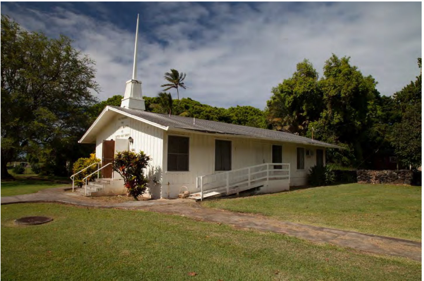
Photo 48: Latter-day Saint Chapel (257), camera facing northeast. A portion of the encircling churchyard wall (842) extends to the right of the chapel.
