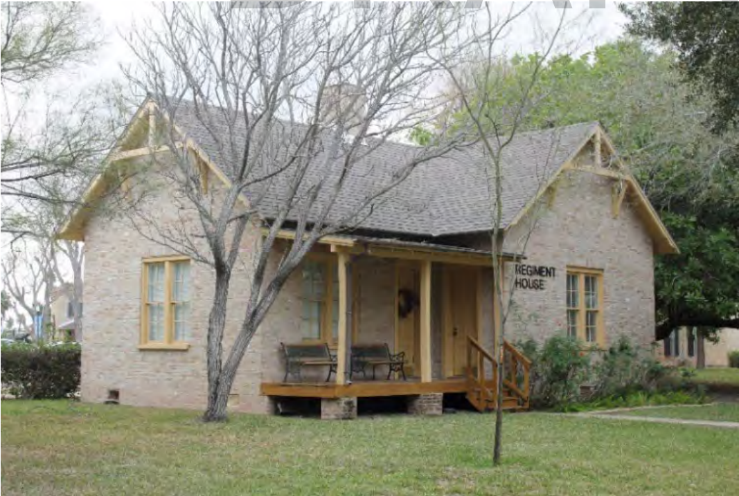
Photograph 24: Section C, Chapel/Officers' Guest House, west view.
