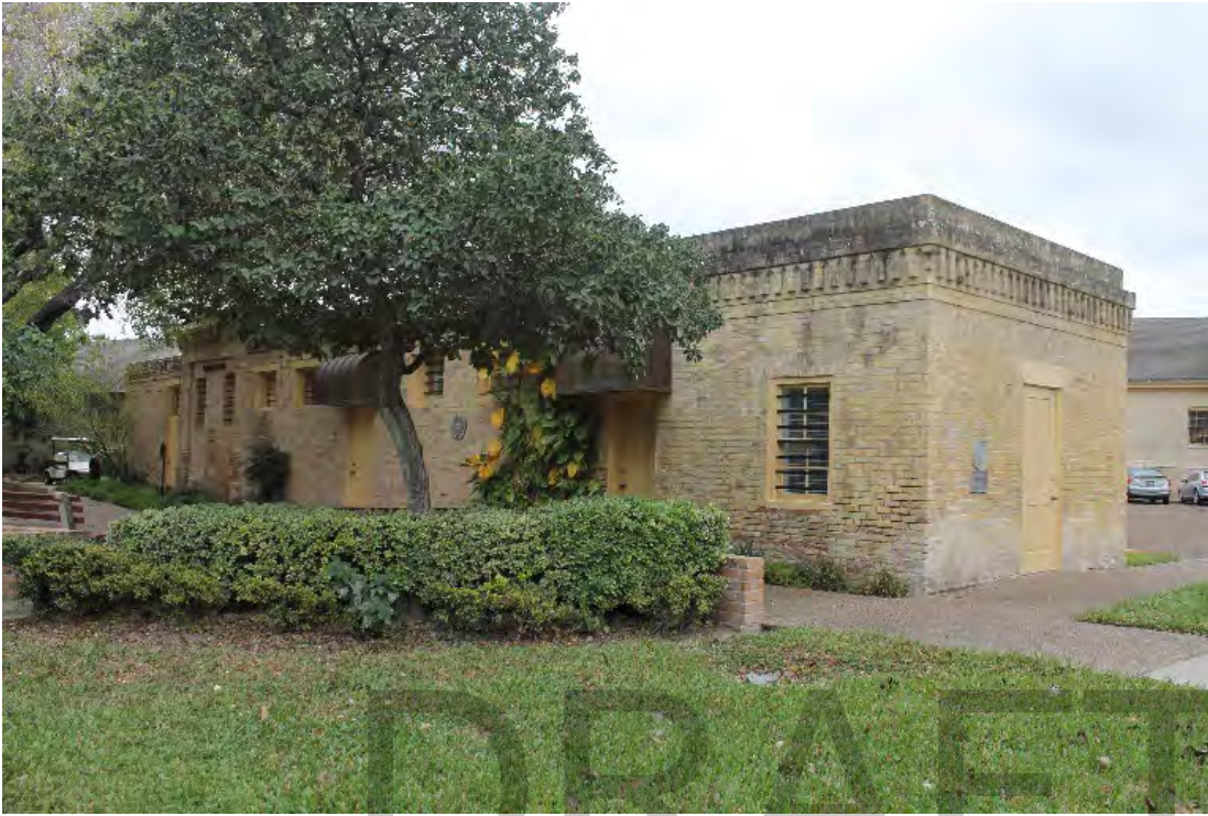
Photograph 19: Section C, Morgue/Laundry Storage Building, southeast view.
