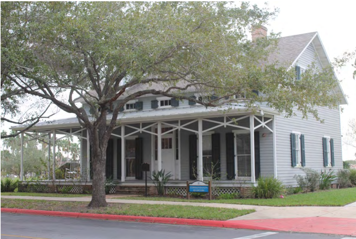
Photograph 14: Section C, Commandant's Quarters, southwest view.
