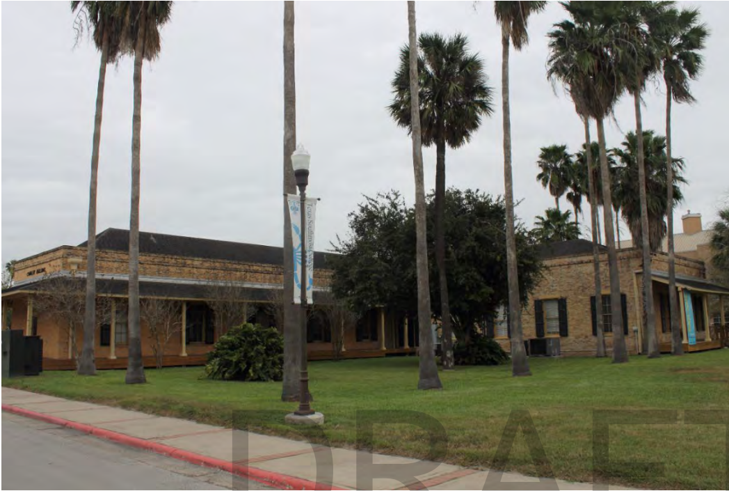
Photograph 11: Cavalry Barracks, northwest view.
