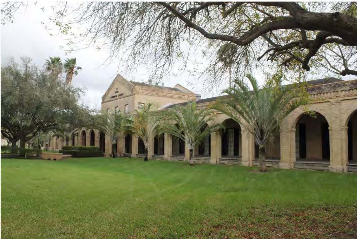
Photograph 16: Hospital Building, southeast view.
