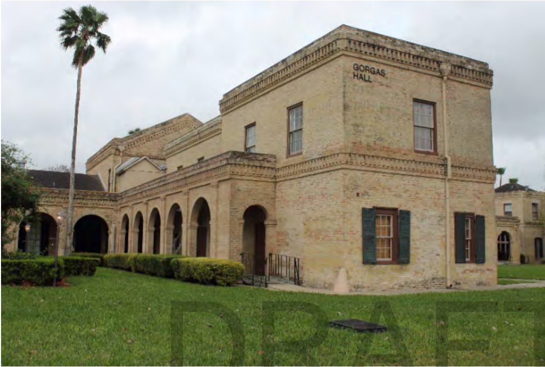
Photograph 15: Section C, Hospital Building, northeast view.
