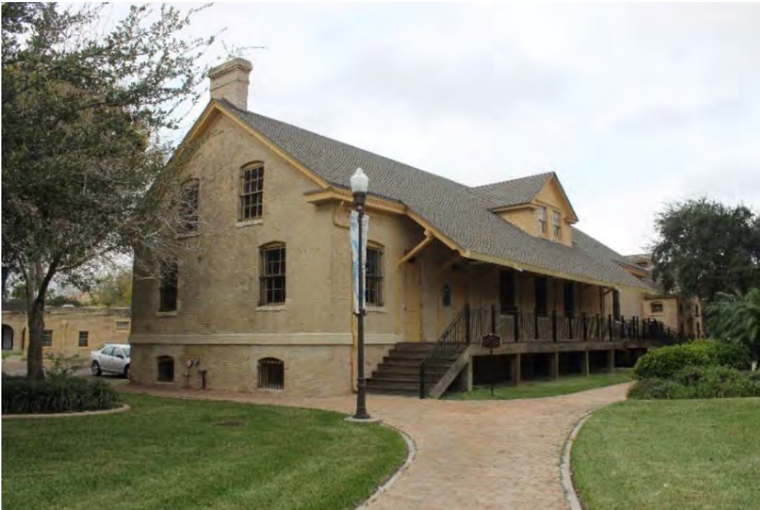
Photograph 20: Section C, Commissary, north view.
