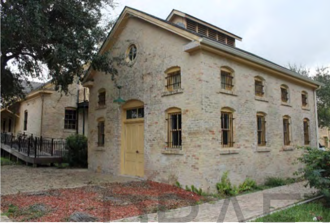
Photograph 23: Section C, Bachelors' Non-commissioned Officers' Quarters/Commissary Annex, west view.
