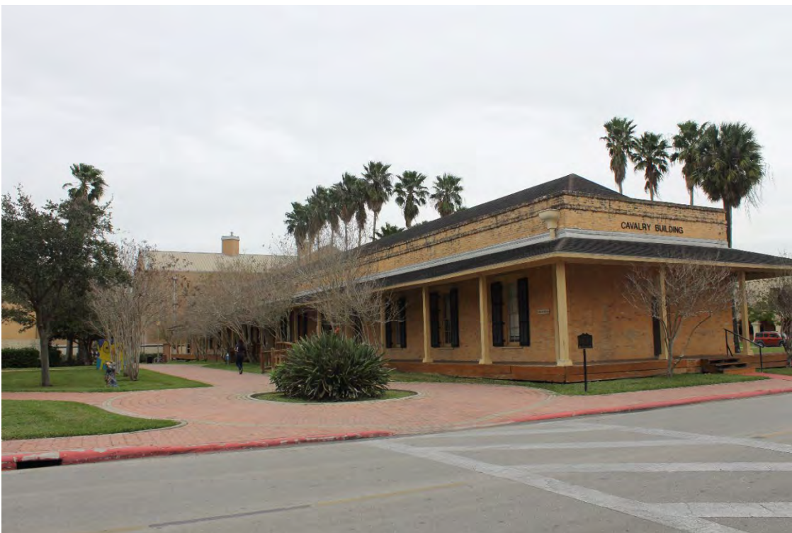
Photograph 10: Section B, Cavalry Barracks, from Gorgas Drive, northeast view.
