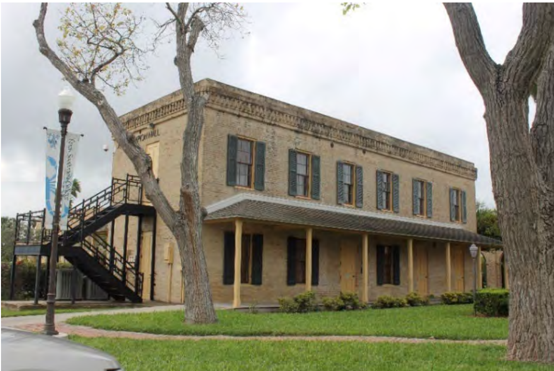
Photograph 18: Section C, Medical Laboratory, northwest view.
