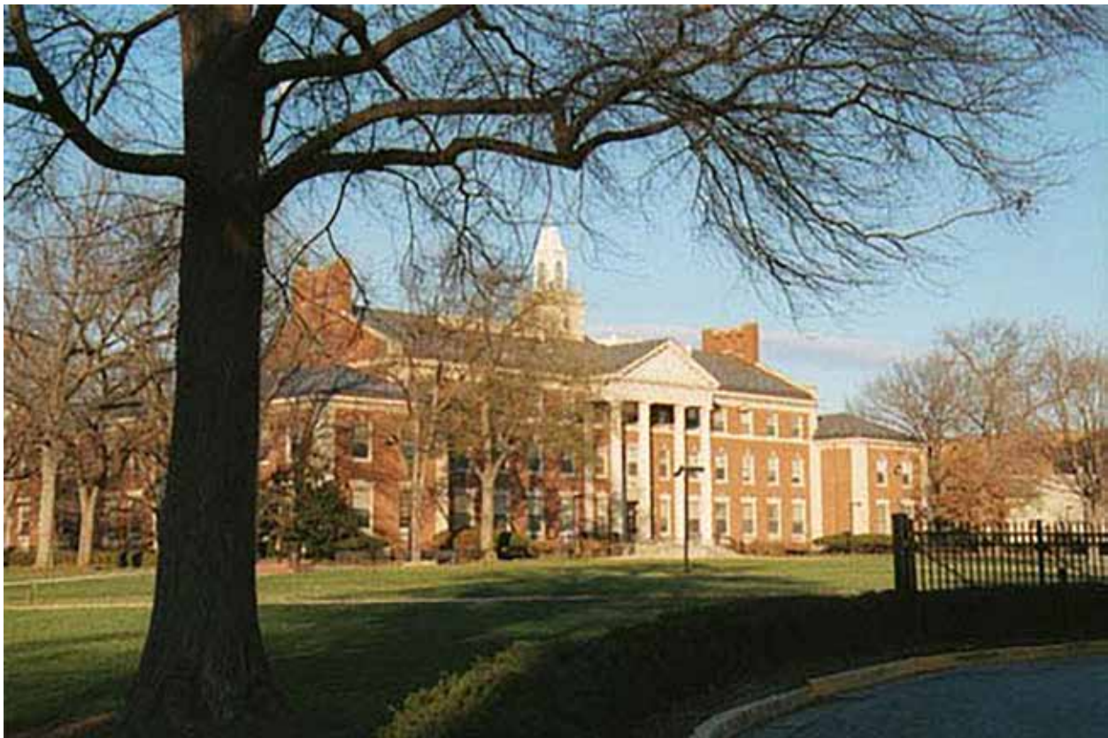
Frederick Douglas Memorial Hall, Howard University, Washington, D.C. (Courtesy of Howard University, photograph by Mohamed Mekkawi).
