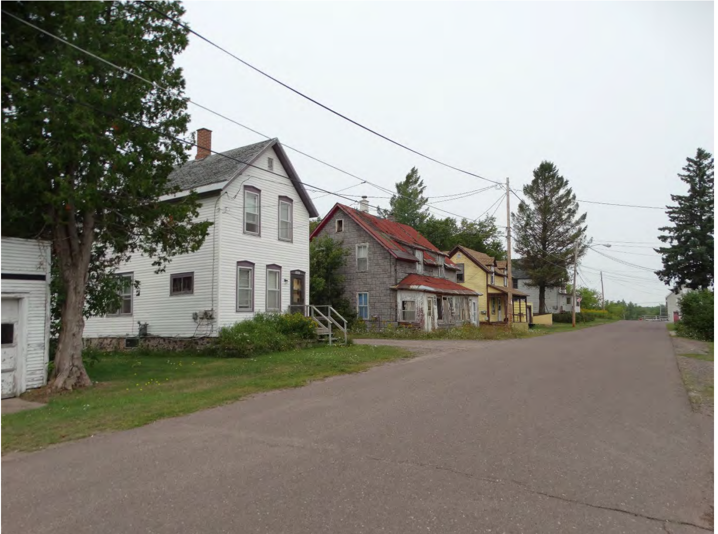
Blue Jacket Housing Location Landscape Character Area E. Worker housing along Fourth Street (left to right: Map ID#s 240, 242, and 241).
