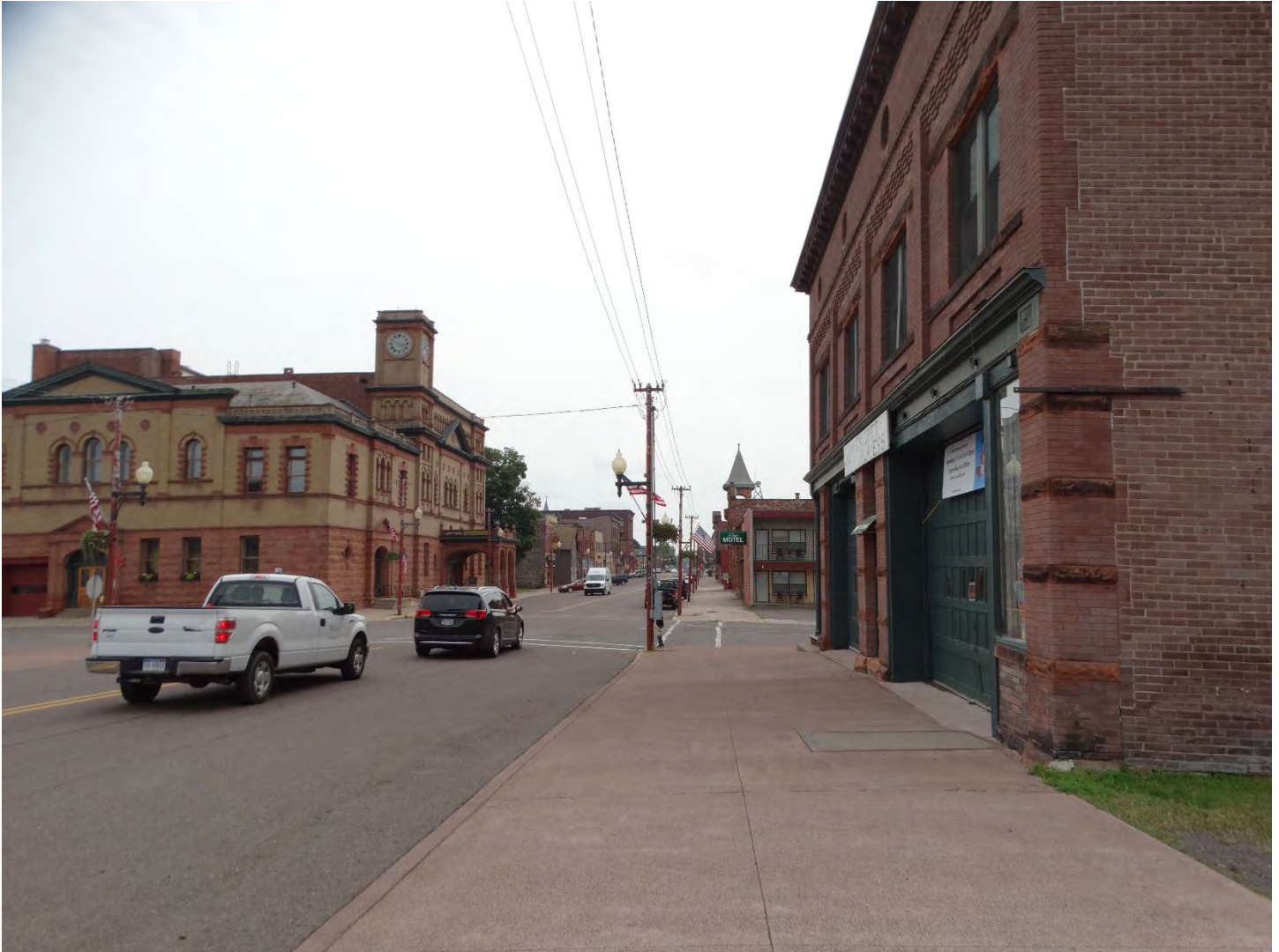
Civic Core Landscape Character Area D. The Calumet Theater (Map ID# 188) is on the left side of Sixth Street and the Schumaker Building (Map ID# 190) on the right.
