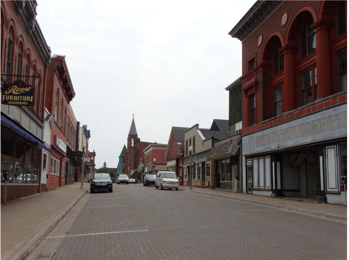
Civic Core Landscape Character Area D. Commercial buildings line Fifth Street (left foreground, left to right: Map ID#s 111 and 110; right foreground: Map ID# 112). Temple Square is in the distance.
