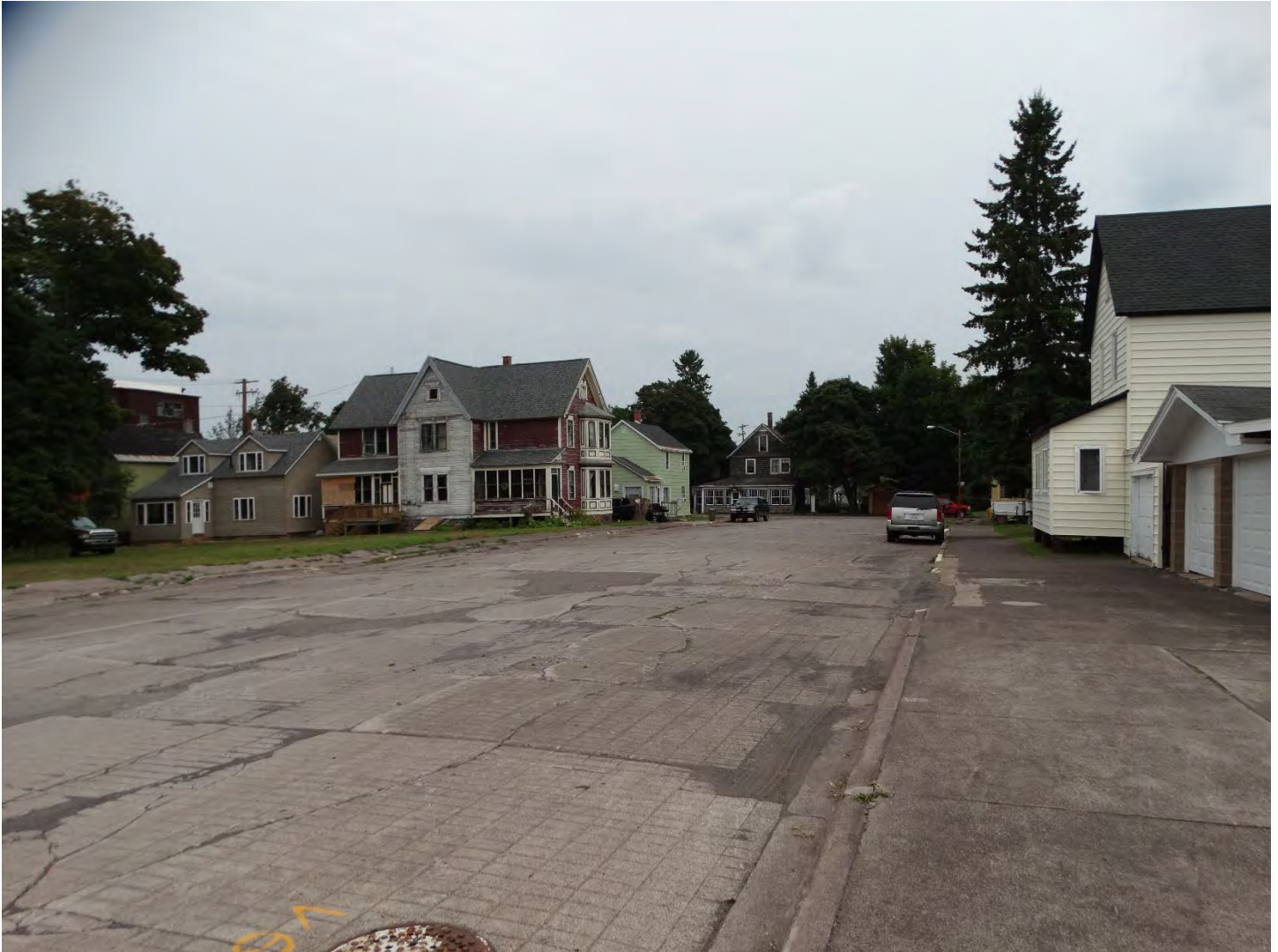
Village of Calumet Housing Location Landscape Character Area F. On the left side of Seventh Street is a lot containing three workers housing residences, including the former St. Anne's Rectory (right to left: Map ID#s 376, 377 and 378).
