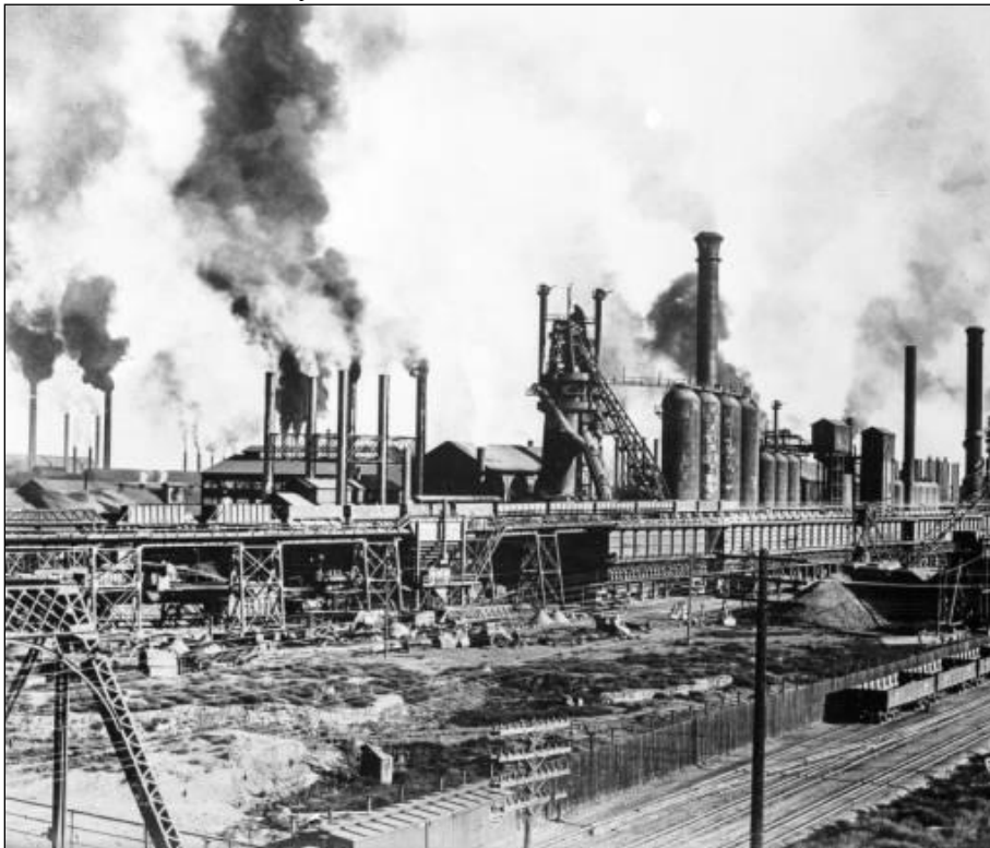
Figure 10. CF&I's Minnequa Works steel plant covered a large tract in the southern part of Pueblo, Colorado. Courtesy of Denver Public Library, Western History and Genealogy Department, photograph by Theodore Anderson, image number X-10630, ca. 1913-20, Denver, Colorado.
