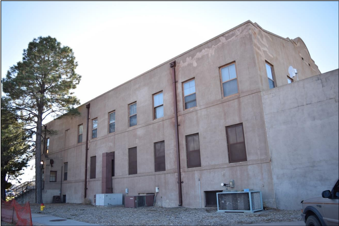
Photograph 15. Office annex (east wall), with post-1960 addition to right. View southwest.
