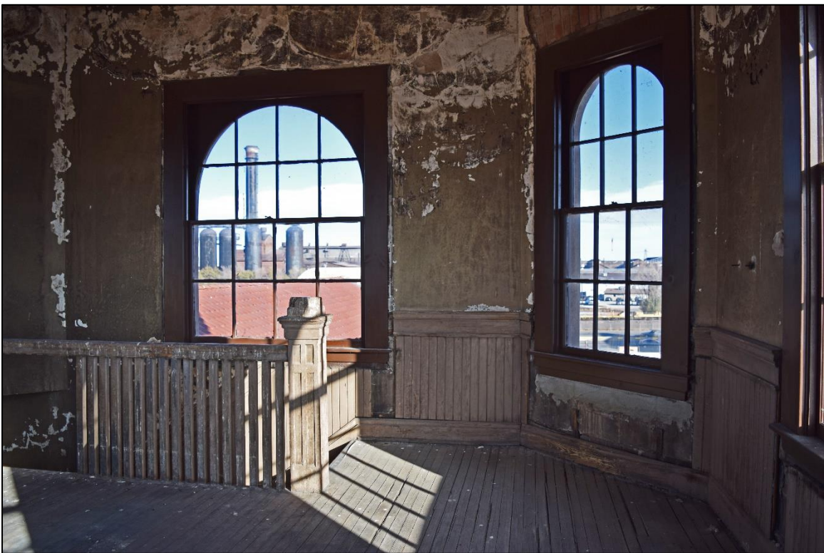
Photograph 8. Office building interior of fourth-story drum with former steelwork visible through window. View east.
