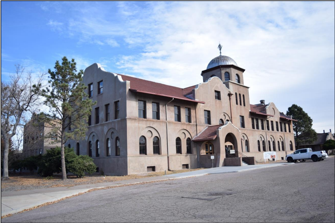
Photograph 3. Office building (front and west wall), with west wall of office annex (left) and dispensary/employment office (right). View northeast.
