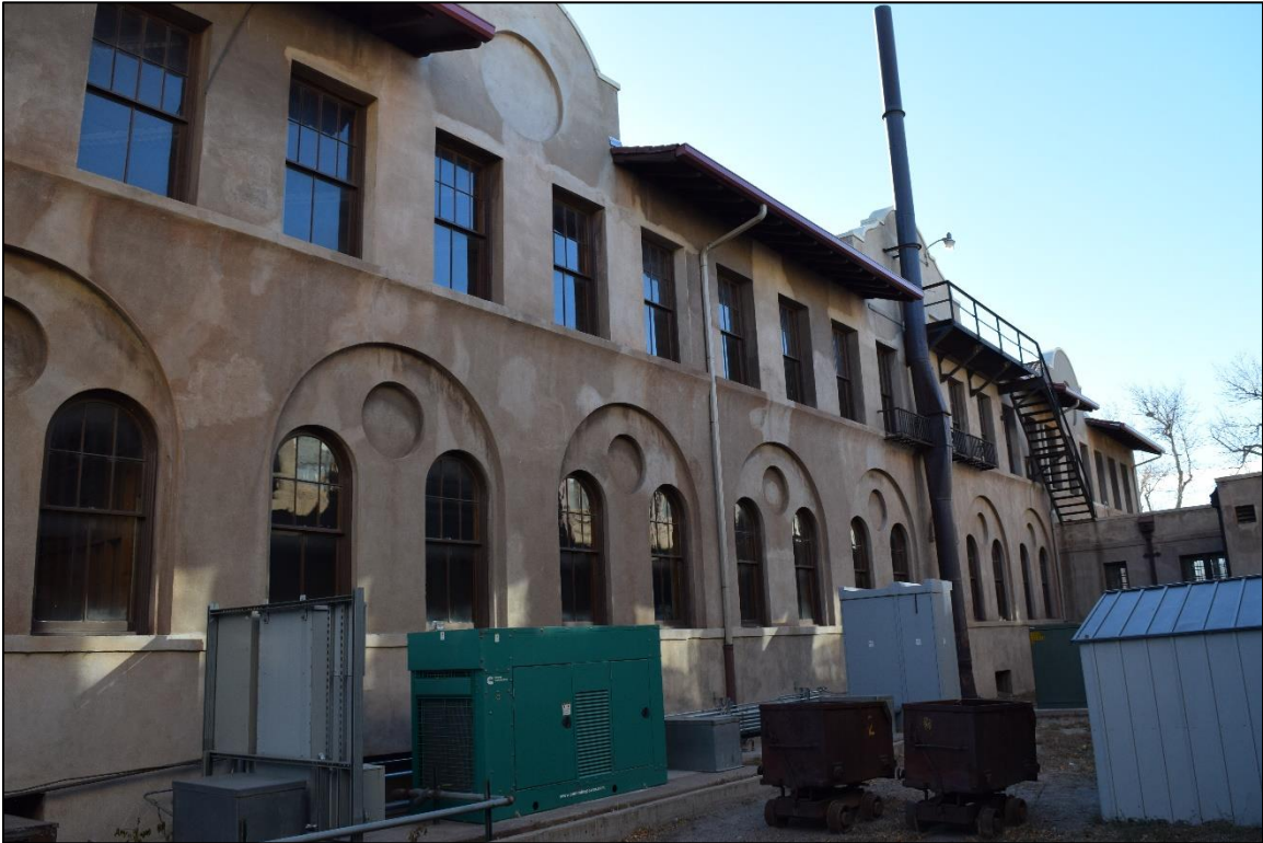
Photograph 5. Office building rear (north wall) with connector to office annex at right. View west-southwest.
