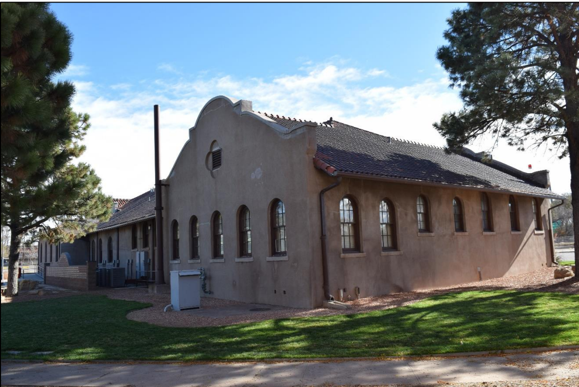
Photograph 10. Dispensary/employment office rear (north wall) and west wall. View southeast.
