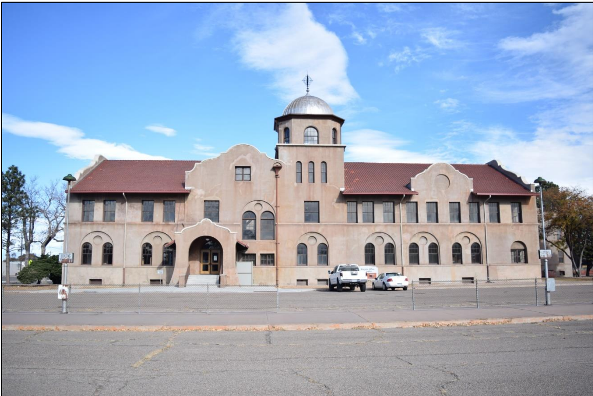
Photograph 2. Office building front (south wall). View north.
