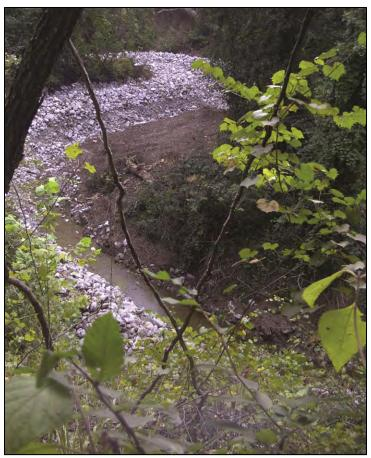
Figure 5.4. Longitudinal peaked stone toe dike placed in the bottom of Harlin Bayou by the U.S. Army Corps of Engineers. *Photo: Diana Greenlee*
