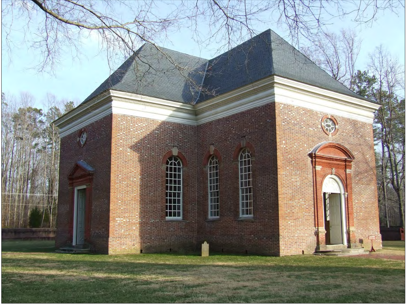
FIGURE 9. CHRIST CHURCH, A HISTORIC EPISCOPAL CHURCH IN LANCASTER COUNTY, WAS BUILT BETWEEN 1732 AND 1735
