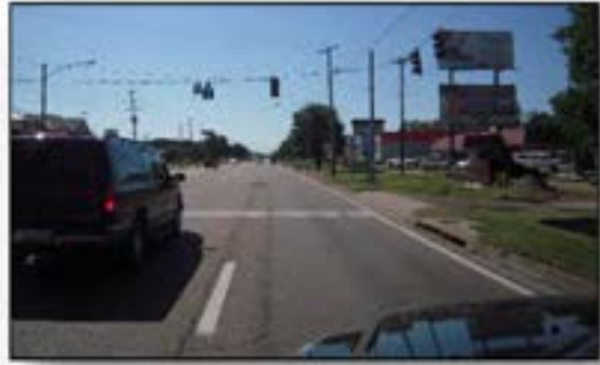
This strip commercial corridor serving as a gateway for one MHNHA community could be anywhere in America.
